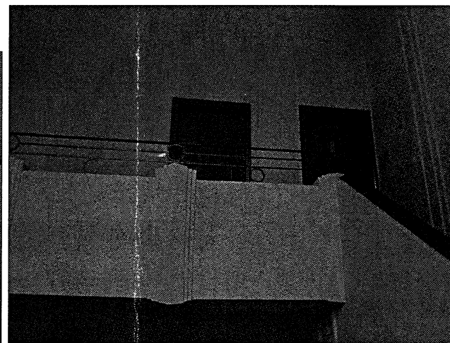
BALCONY RAILING CAMERA POSITION 6
