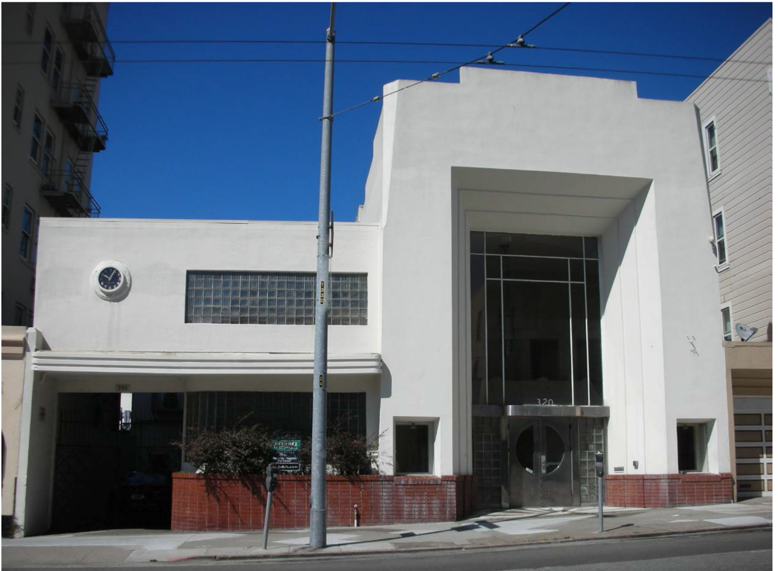
Current condition, front façade, facing north.
