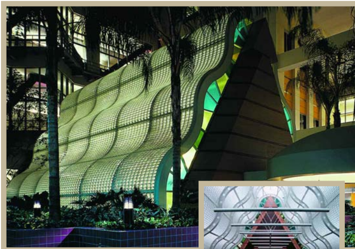
Veteran's Administration Hospital Chapel, Detroit, MI Architect: Smith, Hinchman & Grylls, Inc. // DECORA® Pattern
