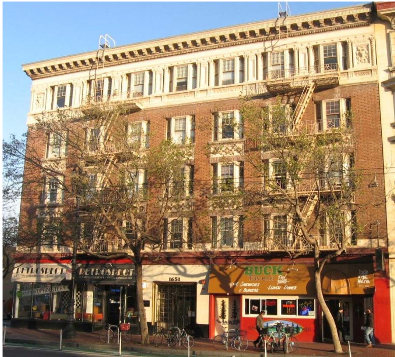
Figure 8 - 1649 Market Street, Market Street elevation
