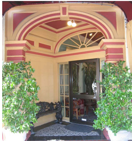
Figure 33 - 1666 Market Street, entry paneling
