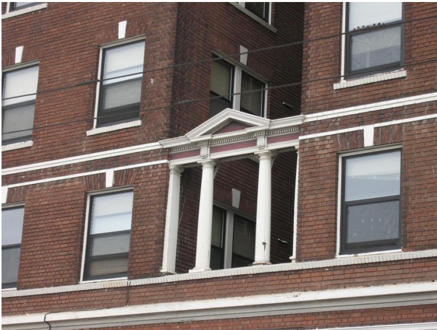
Figure 7 - 20 Franklin light court and pediment detail
