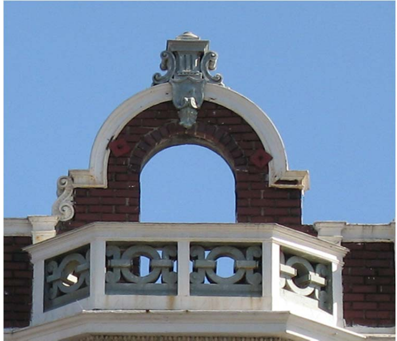
Figure 28 - 1693 Market St, parapet detail
