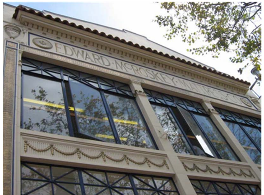
Figure 24 - 1687 Market, upper floor detail
