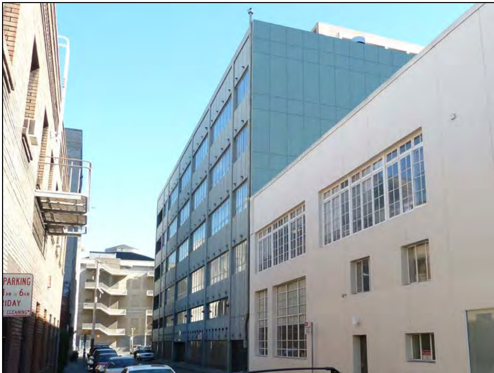
Photograph 3: 150 Hayes Street, north and west sides, camera facing east, 11/4/13.
