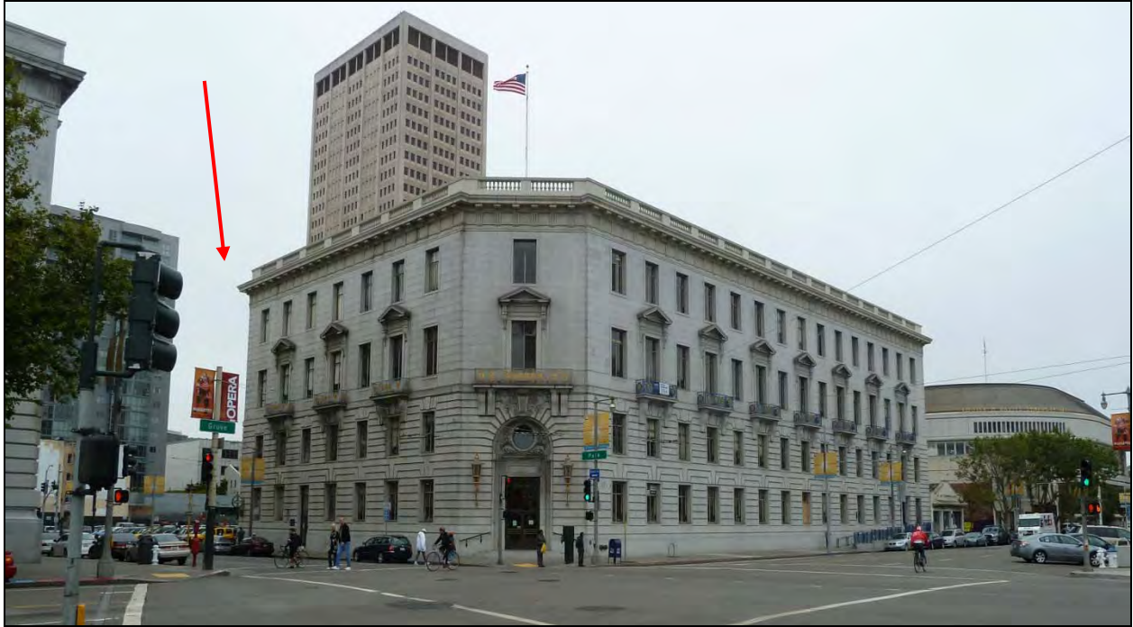
Figure 5: Department of Public Health Building Proposed project location indicated with red arrow
