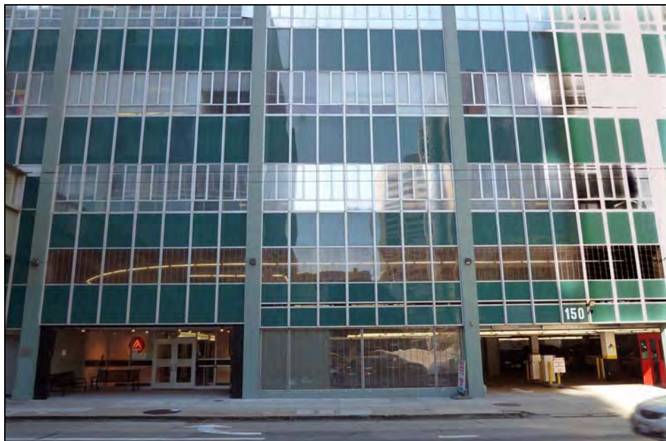
Photograph 5: 155 Hayes Street, south side detail, camera facing north, 11/4/13.
