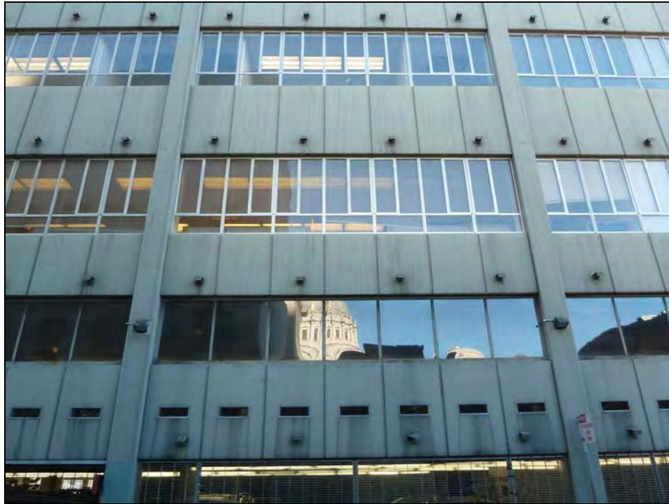
Photograph 6: 155 Hayes Street, north side detail, camera facing south, 11/4/13.
