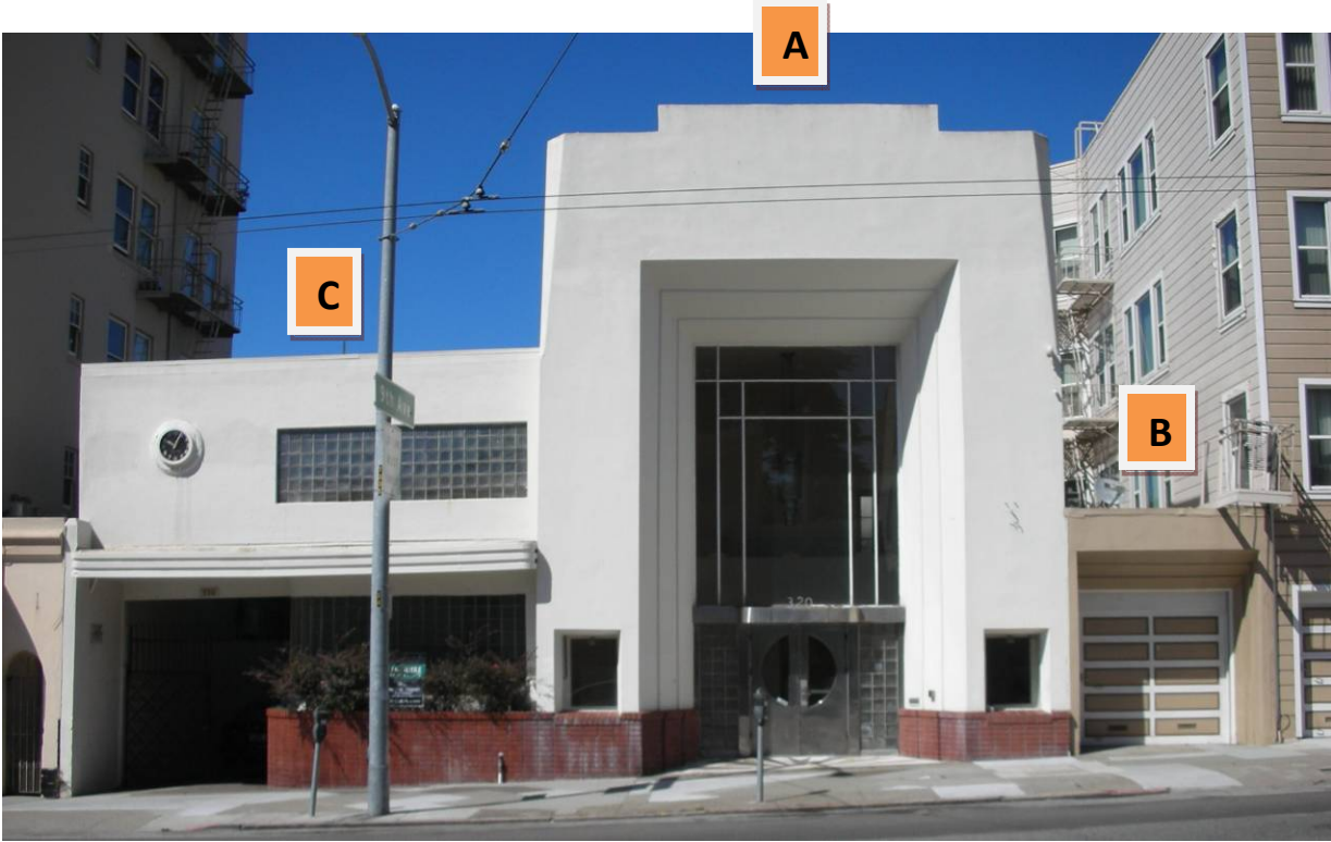
The original building consisted of the tall center structural bay (A), a garage added later in 1932 (B), and a horizontal addition in 1940 (C).
