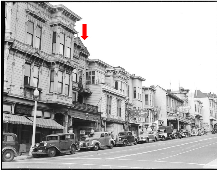
Figure 9: 1686-1690 Post Street is visible in this July 3, 1942 view looking northeast on Post Street at the Japanese-American commercial district. At that time the storefront was occupied by the Nippon Drug Co. Source: Dorothea Lange, National Archives and Records Association.
