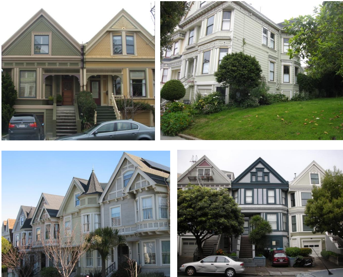
Clockwise from top left: A pair of small-scale mirrored cottages on Carmelita Street; detail view of the direct connection between a house on Waller Street and Duboce Park; a row of Nelson's 2 1/2 story over raised basement Queen Anne buildings on the west side of Pierce Street; and a row of Nelson's houses on Pierce Street, several of which feature applied stick work reminiscent of the Tudor style.
