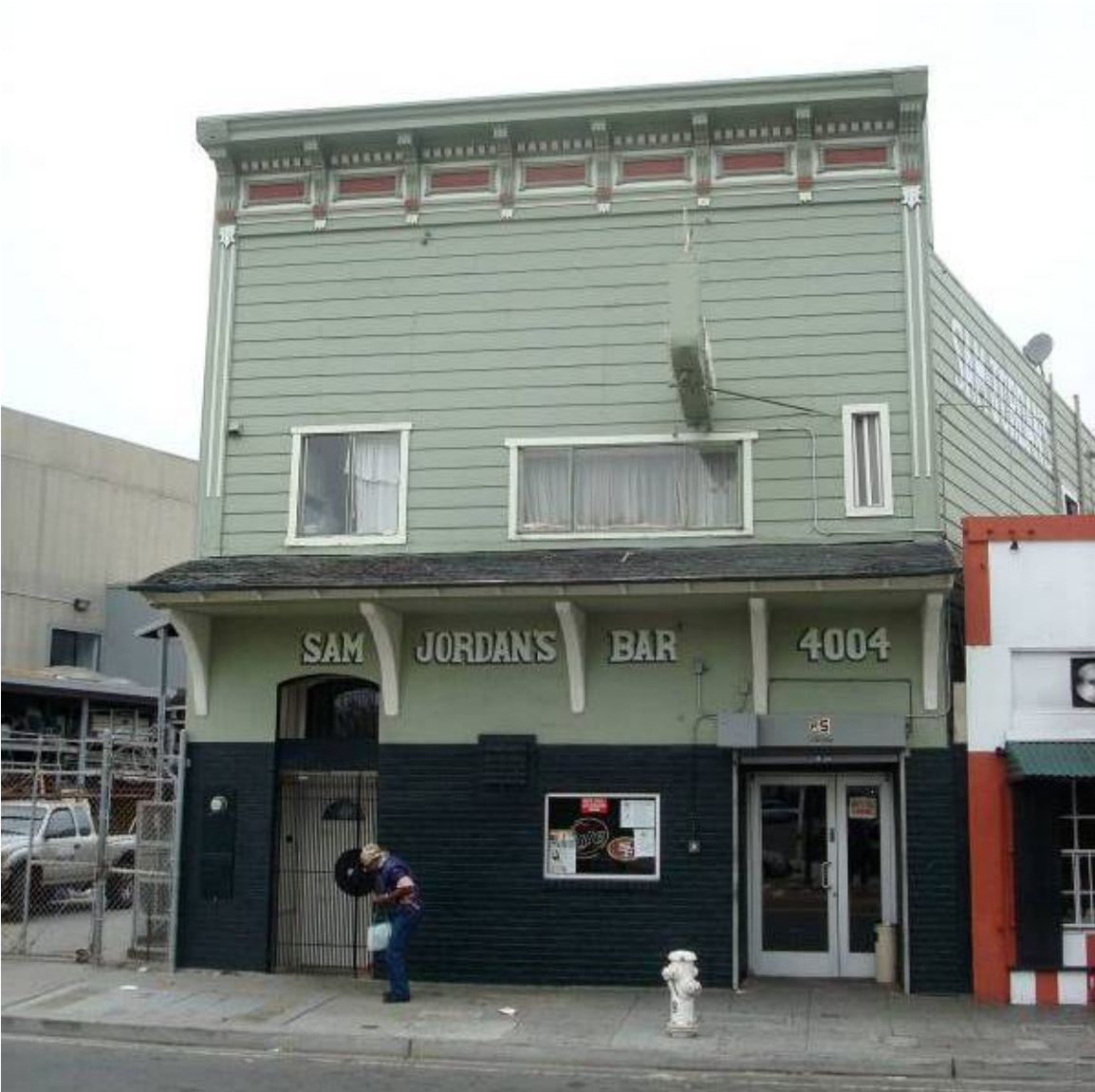
4004-4006 Third Street, Sam Jordan's Bar, primary facade.
