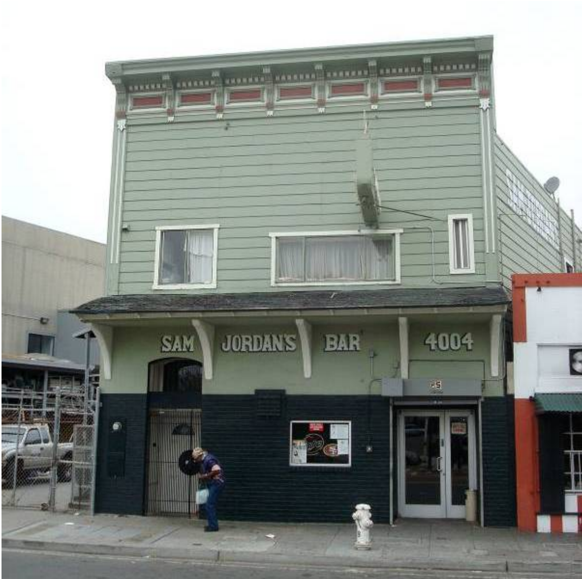
4004-4006 Third Street, Sam Jordan's Bar, primary facade.
