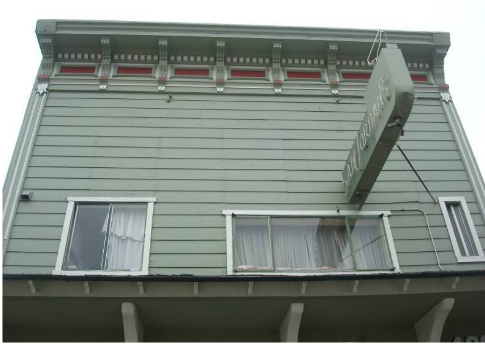
Second story, primary facade.
