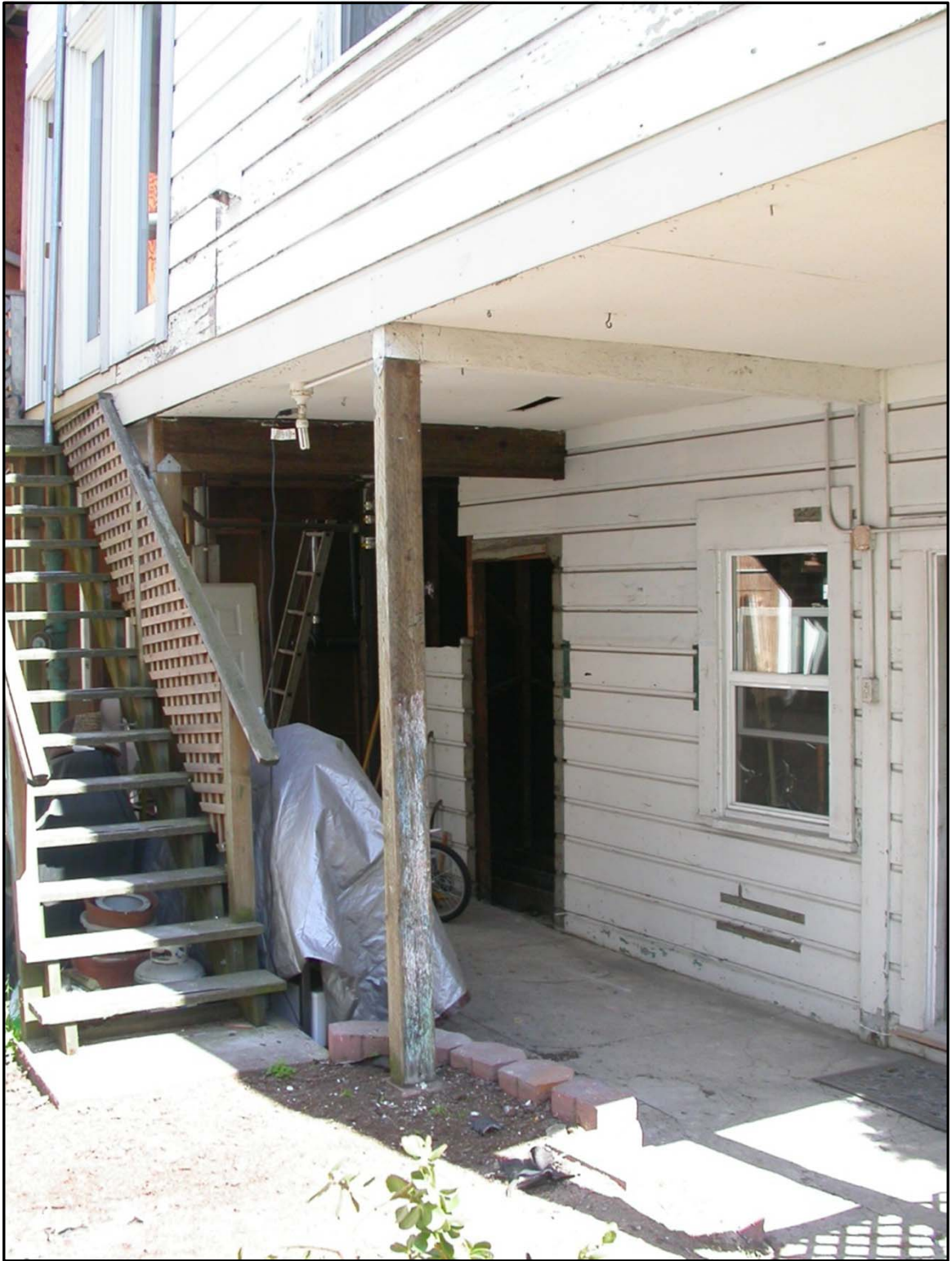
Subject Property, Rear Façade, Area of Work
