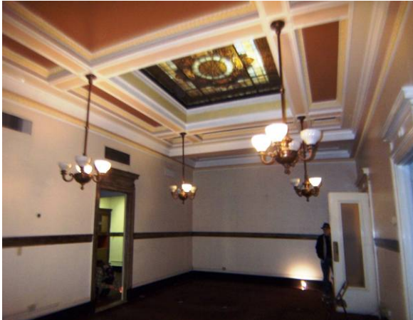
Figure 40. Waiting/Reception Room (S-9) located on the second floor south. Note historic light fixtures and skylight. Source: KVP 2009.
