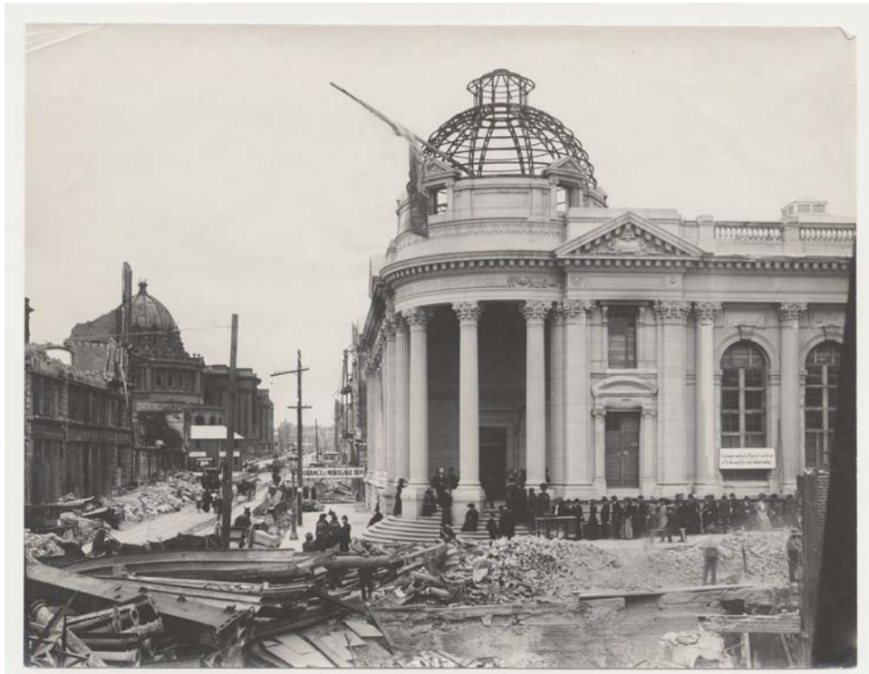
Figure 1. “Hibernia 1906 Opening Day” - after the earthquake and fire
