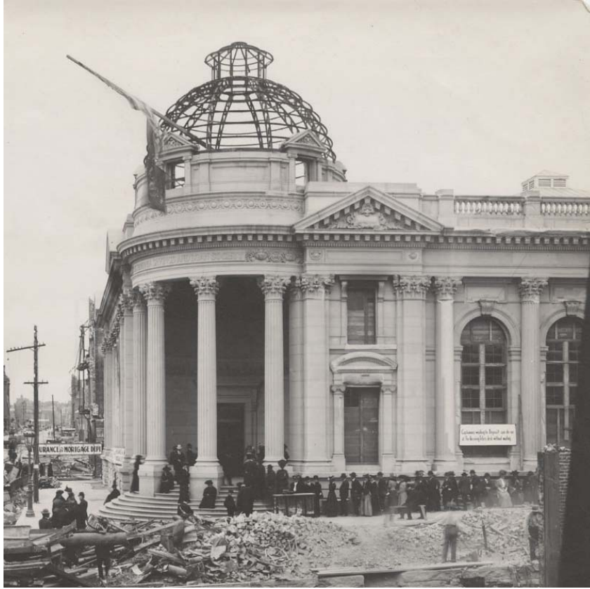
Item 14. Hibernia Bank Building, 1906. Note the shutters over some of the windows. Source: California Historical Society.
