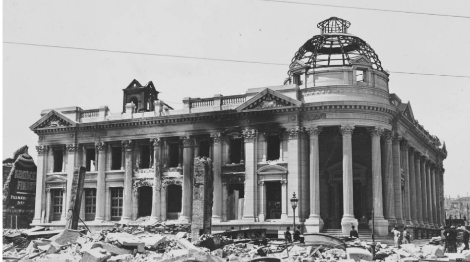
Figure 8. Hibernia Bank Building, April 18, 1906. Note smoke and fire damage above windows and damage to rotunda. Source: California Historical Society.
