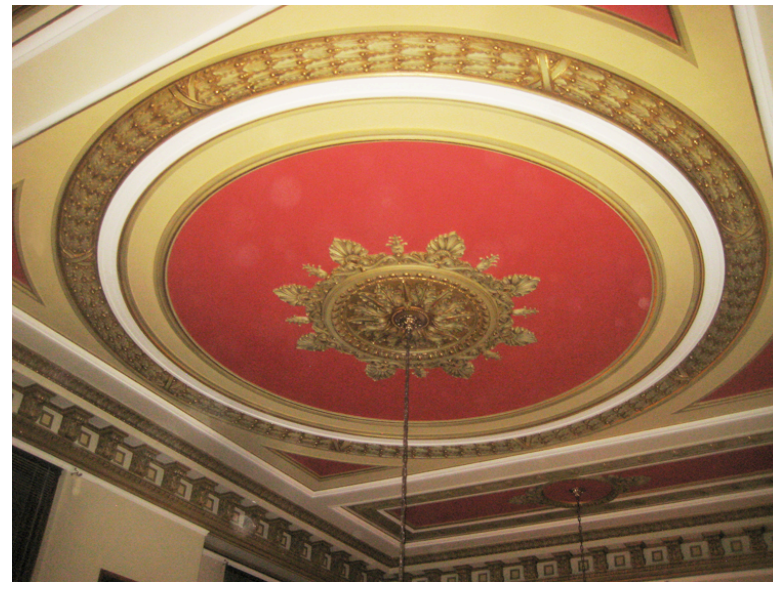
A: View of ceiling in SW Meeting Room.
