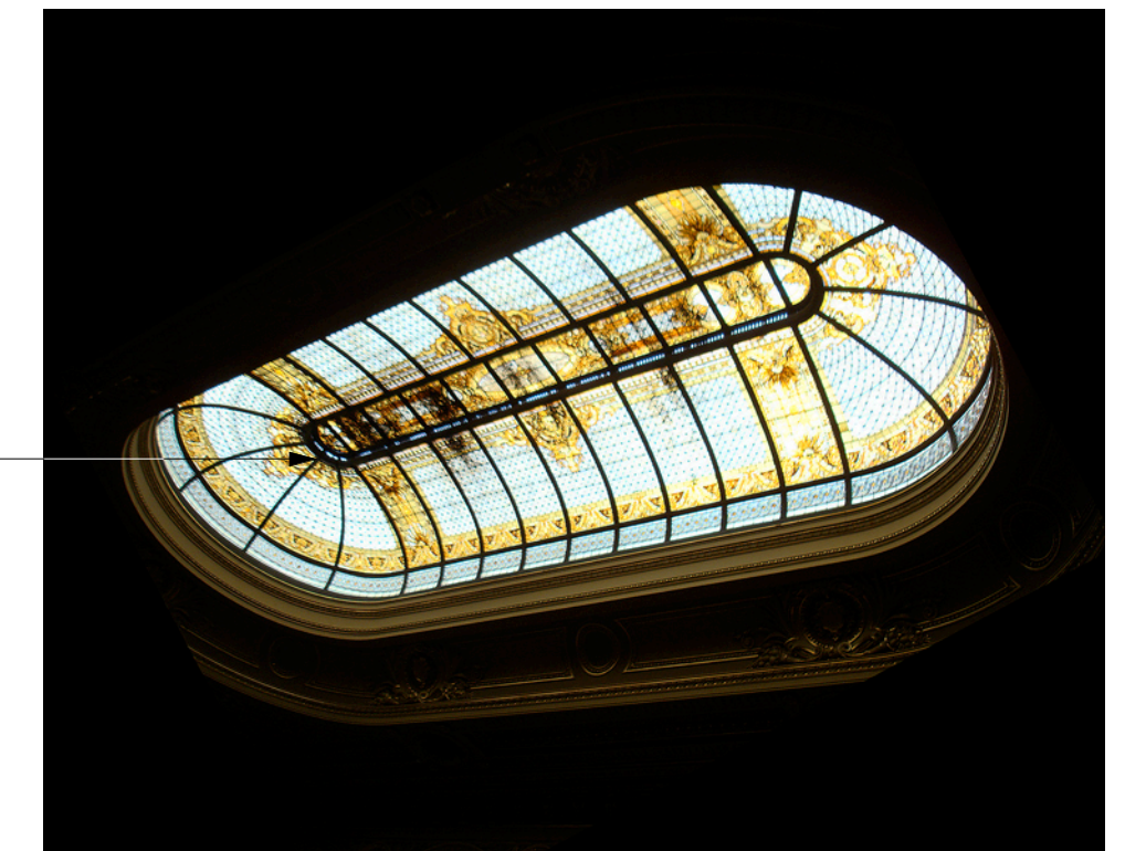
G: View of skylight dome located in the 1905 addition of the Banking Hall. Sprinklers to be located behind upper vent grille to be able to protect glass and leading by bathing surface with water to keep dome intact.
