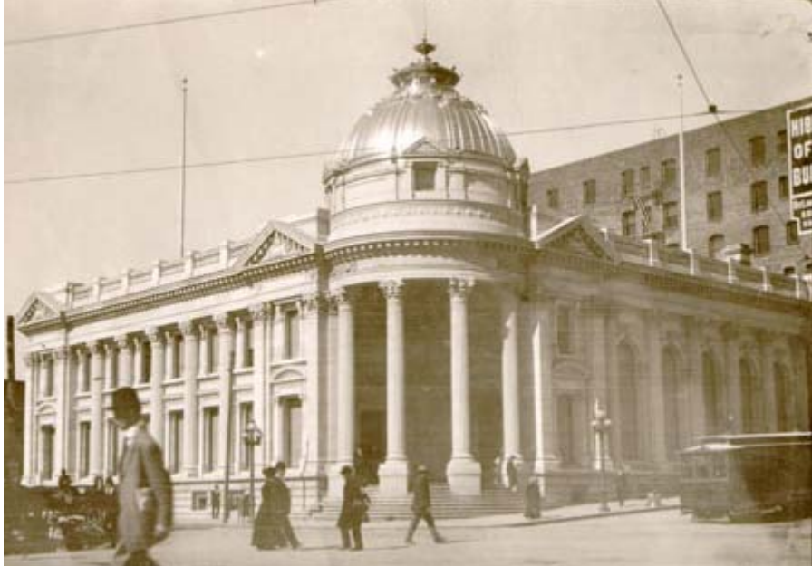
Item 20. Hibernia Bank Building, 1908, repaired after the fire. Note the gleam of the gilded dome. Source: San Francisco History Center, San Francisco Public Library.
