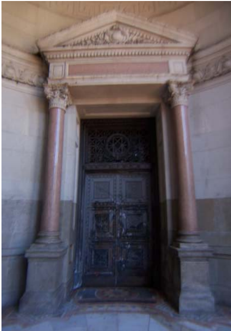
Figure 16. Main entrance located in the rotunda. Source: KVP 2009.
