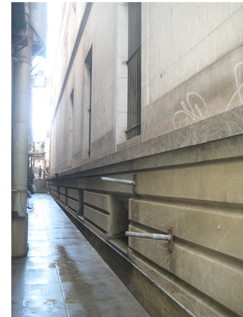
A: View of north side yard looking east
