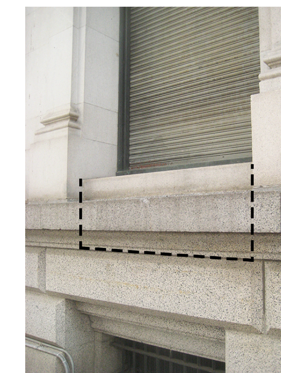
View of west window indicating stone area to be removed and modified.
