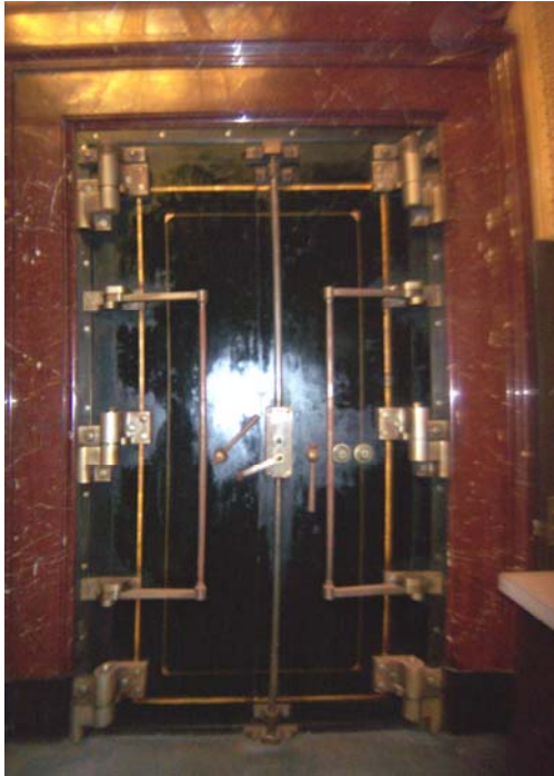
Figure 56. Exterior of vault doors(F-5) in the Banking Hall (F-8). Source: KVP 2009.
