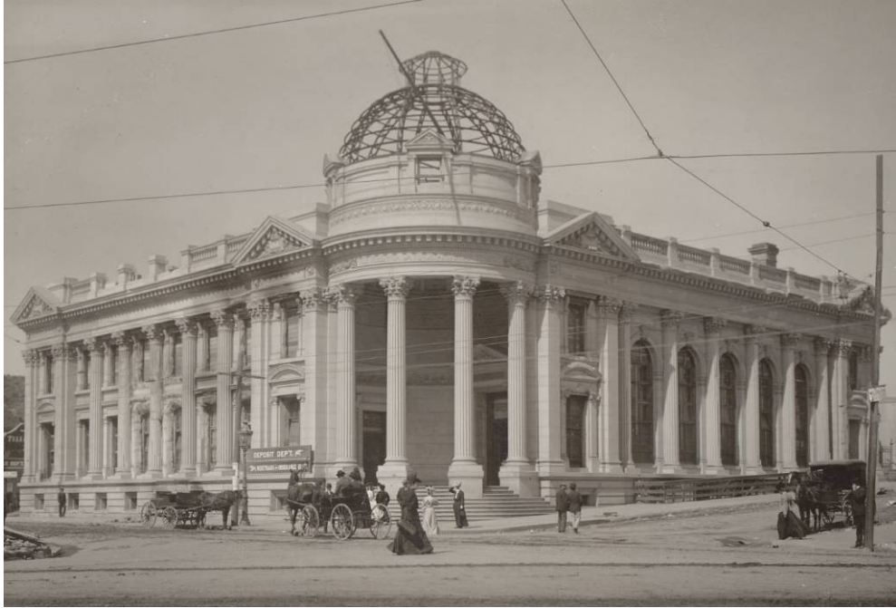
Item 18. Hibernia Bank Building, 1906. Courtesy California State Library, Stanley Mosk Library and Courts Building.
