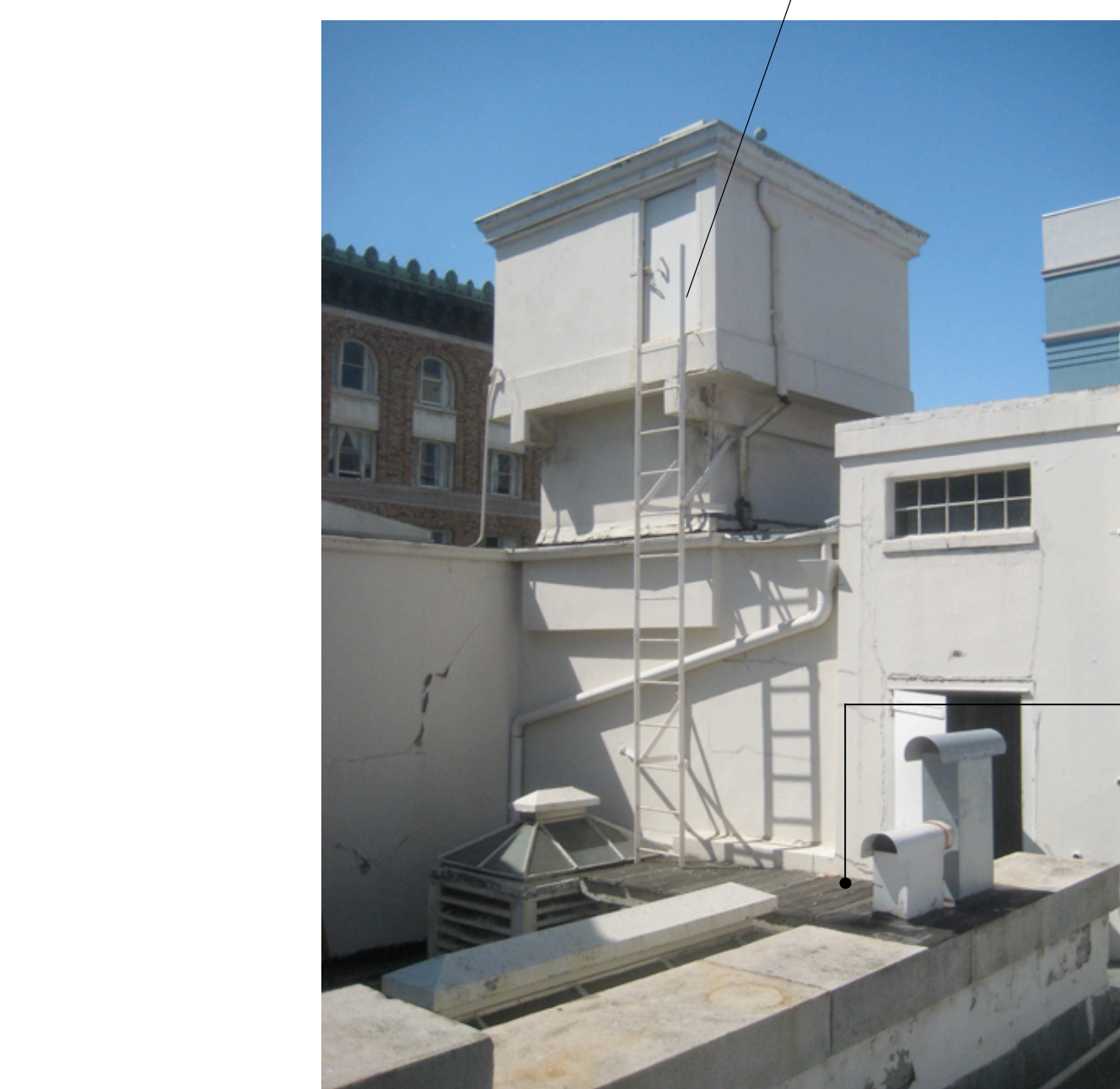
A: View of existing elevator penthouse
