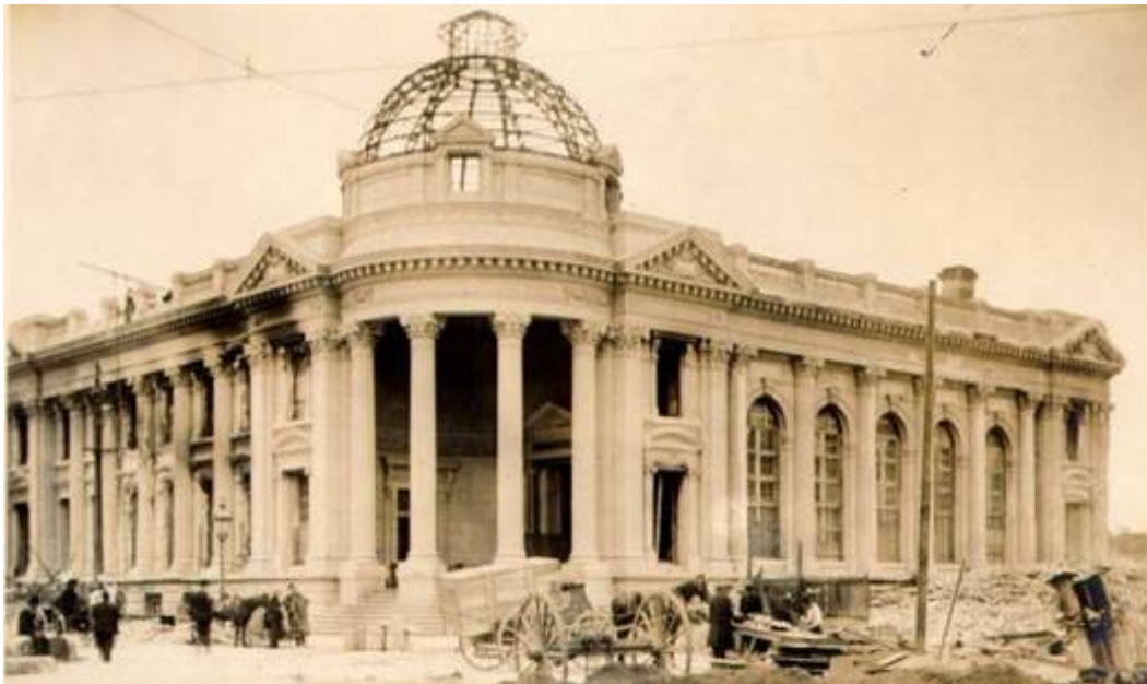
Item 13. Hibernia Bank Building, 1906. Note the window sash at right is different from the current window sash. Source: San Francisco History Center, San Francisco Public Library.
