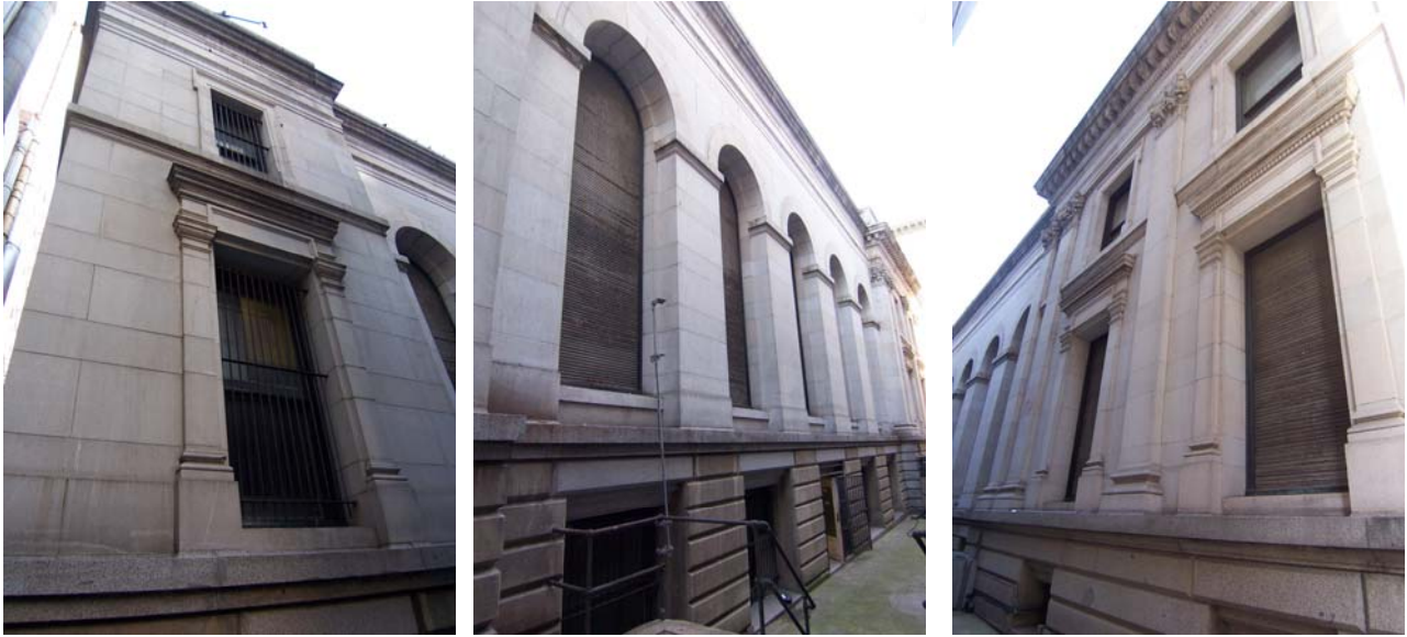
Figure 12. Details of west facade. From left to right: north bay, center bays and south bays.
