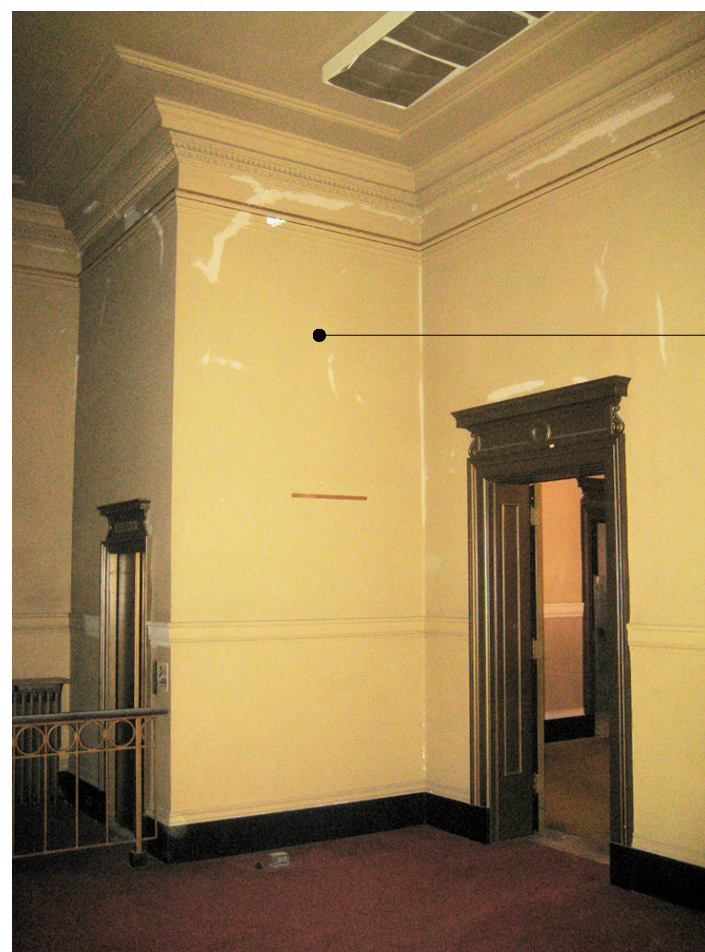
B: View of elevator in the Southeast corner of the customer waiting area. Non-historic fence to be removed (lower left). To accommodate new elevator, the west facing wall of the elevator shaft to be rebuilt, 1'-0" further to the west.
