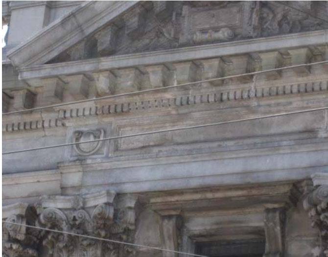
Figure 19. One of two areas of broken dentil molding on the east facade
