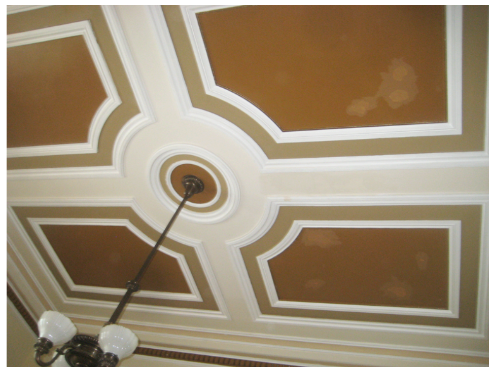
A: View of Customer/Waiting area of 2nd floor offices. Sprinkler heads to be located at center point of inset panels. B: View of ceiling of NW office. Sprinkler heads to be located at center points on either side of the center circular plaque in the east-west (left-to-right) flat panel (cream-colored). C: View of ceiling in Chairman's Office. Sprinkler heads to be centered in center point of light blue flat panel.
