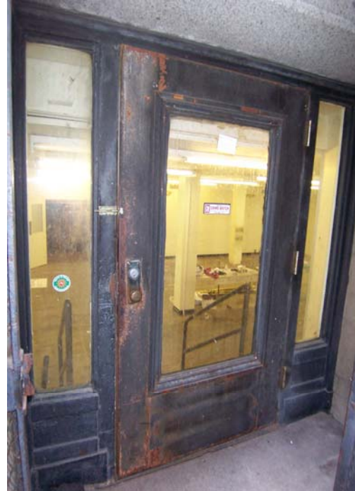
Figure 55. West entrance door, possibly installed in the 1930s. Source: KVP 2009.
