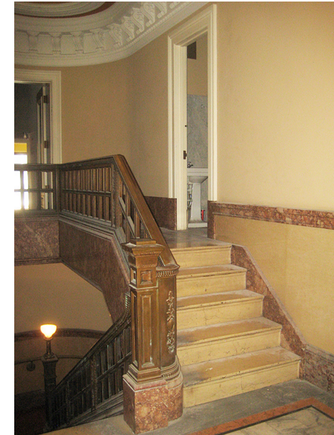
B: View of South stair hall with center door to bathroom removed and frame enlarged to meet required code exit width for new stair to penthouse. Note change of base for door expansion to the south (left in photo).
