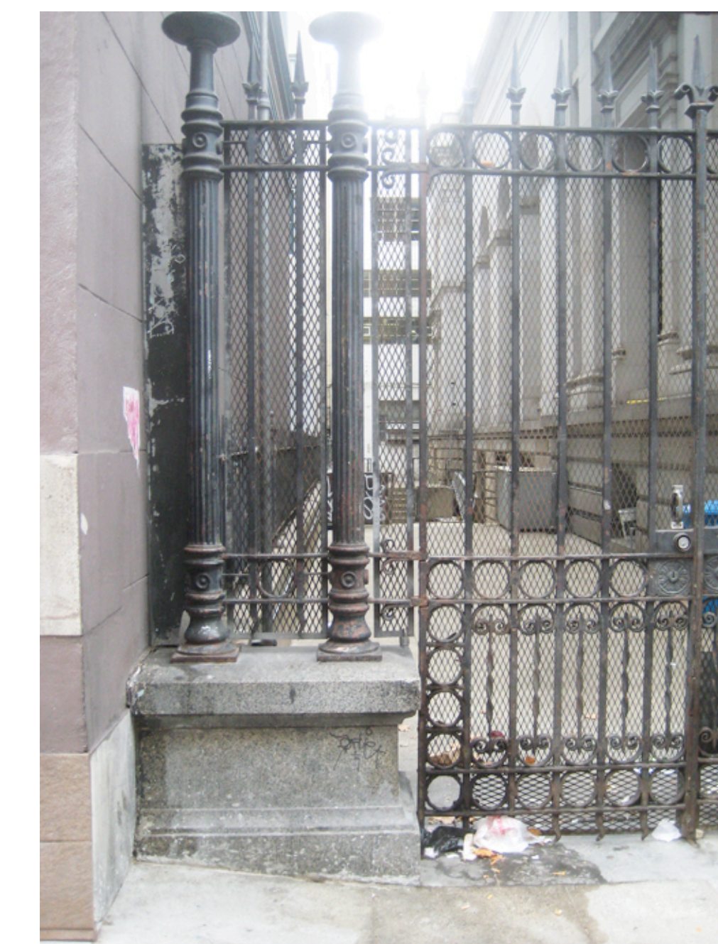
C: Detail of west gate granite base
