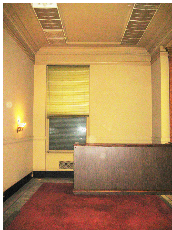
B: View of elevator in the Southeast corner of the customer waiting area. Non-historic fence to be removed (lower left). To accommodate new elevator, the west facing wall of the elevator shaft to be rebuilt, 1'-0" further to the west.
