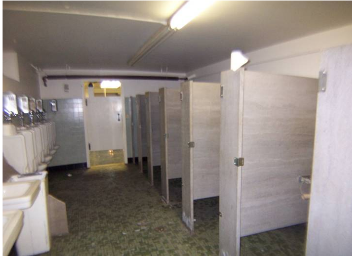
Figure 21. Men's Toilet Room (B-1) located in the basement. Source: KVP 2009.
