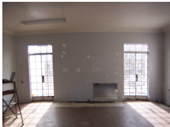
Figure 47. Penthouse (S-15) located on the roof. Source: KVP 2009.
