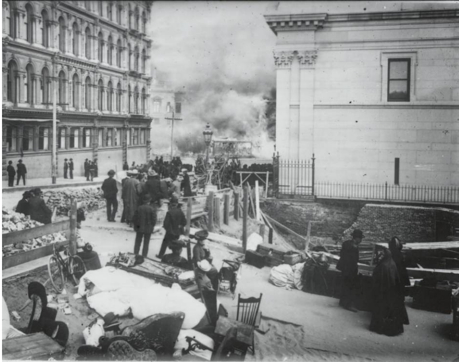
Item 12. North façade of Hibernia Bank Building before the fire, 1906. Source: Bancroft Library, University of California, Berkeley.
