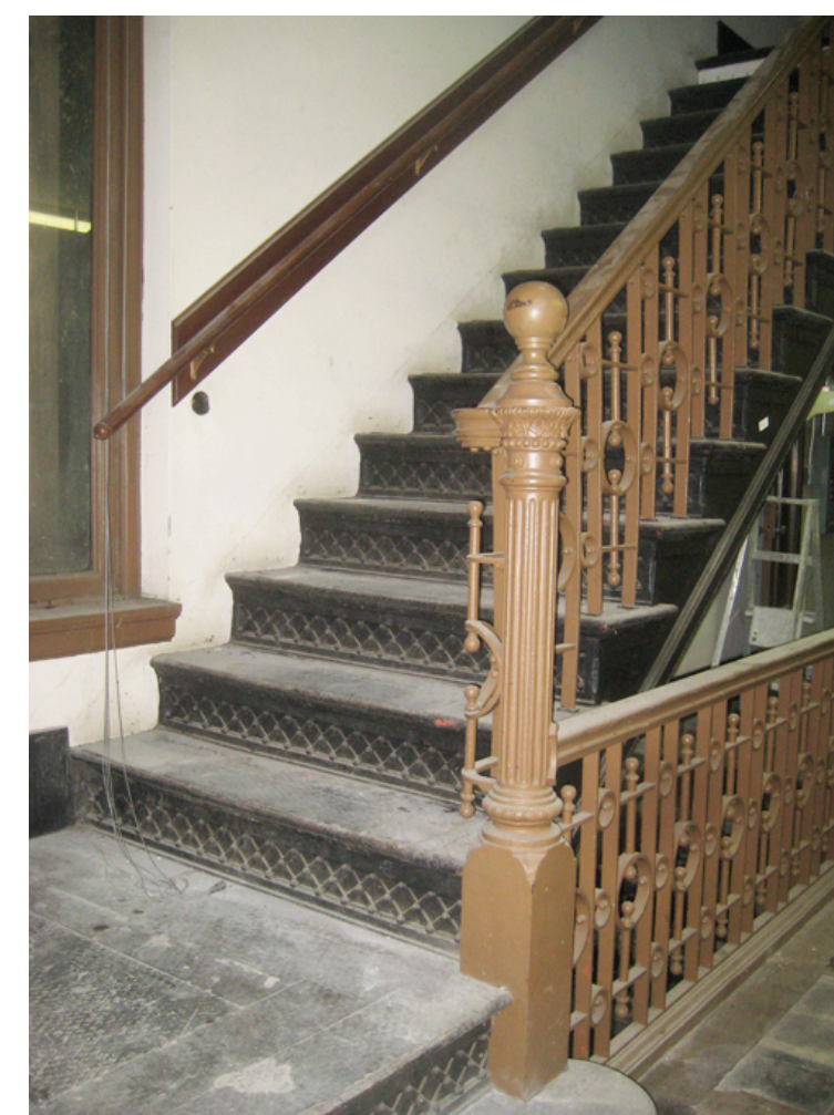
D: View of window to become west exit door from north stair hall
