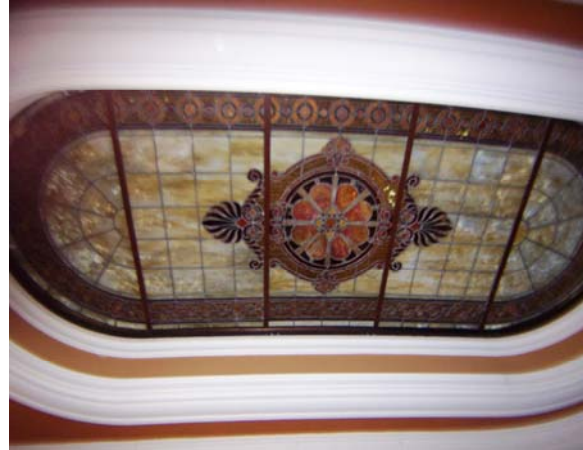
Figure 43. Detail of skylight in Stair Hall (S-10) located on the second floor south. Source: KVP 2009.
