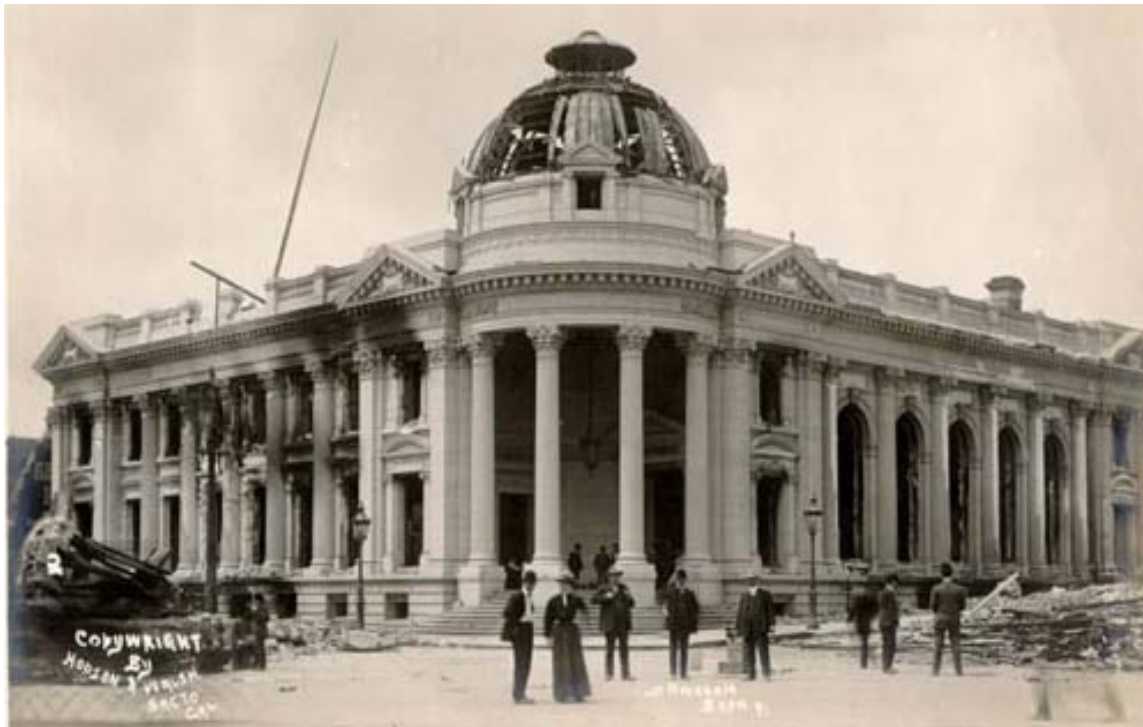
Item 17. Hibernia Bank Building, 1906. Note smoke damage at left dome beginning to be reconstructed. Source: San Francisco History Center, San Francisco Public Library.
