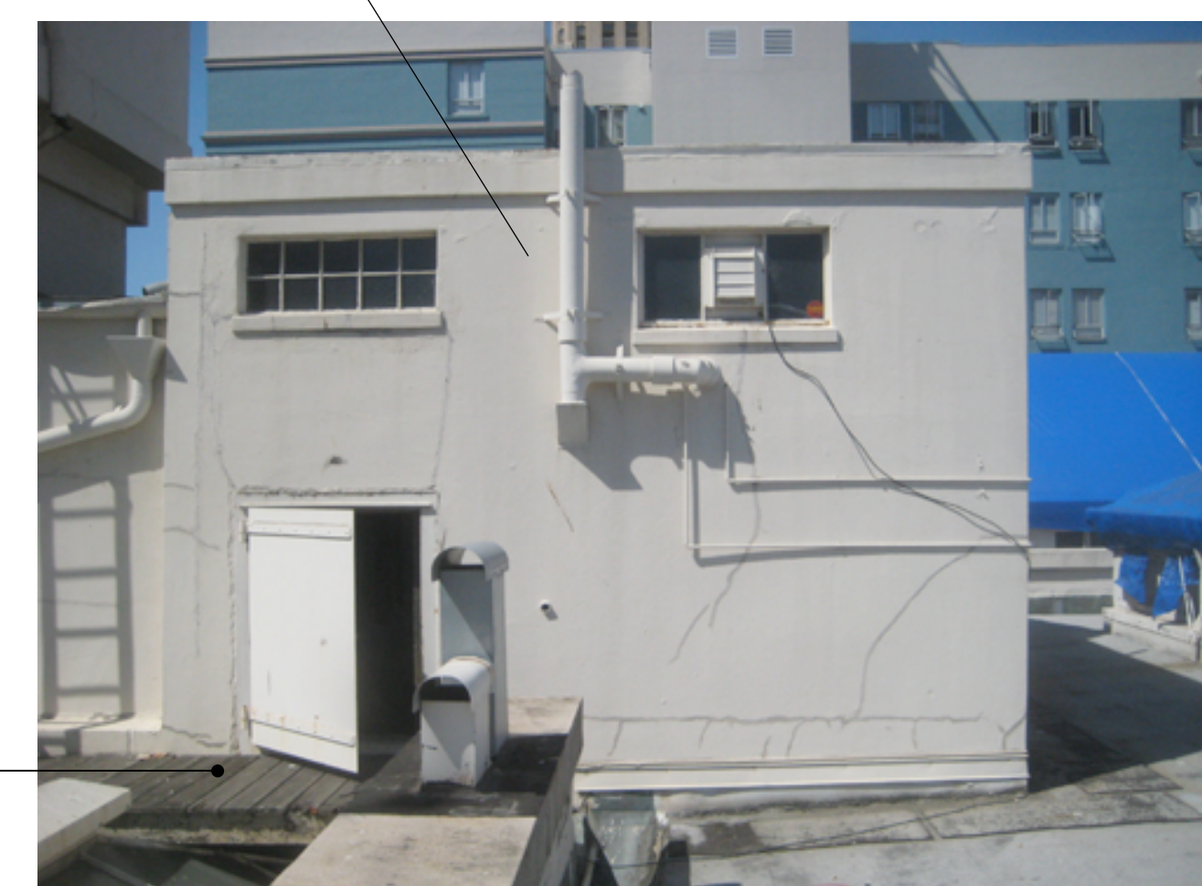
B: West side of penthouse
