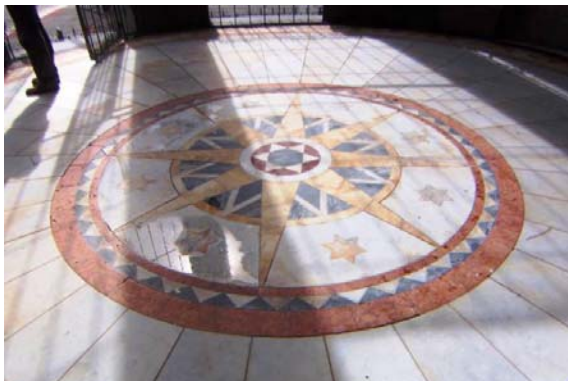
Figure 15 (l). Inlaid marble compass rose pattern on the floor of the interior of the rotunda. Source: KVP 2009.
