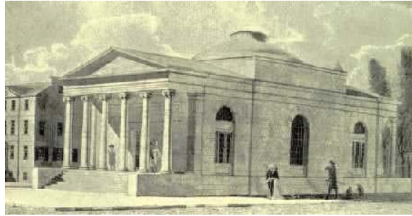
Figure 4. Benjamin Latrobe's Bank of Pennsylvania in Philadelphia.
