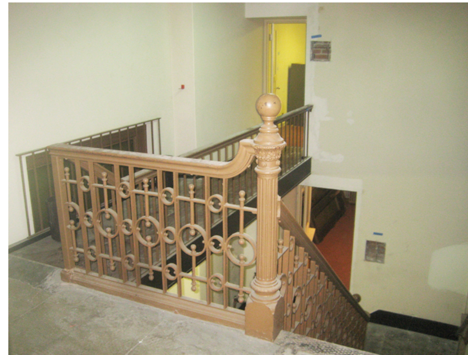
A: Walkway to Mezzanine storage to be removed and door to storage room to be infilled with new concrete shear wall.
