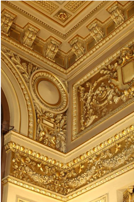
Figure 58. Detail of plaster decoration in Banking Hall (F-8). Source: KVP 2009.
