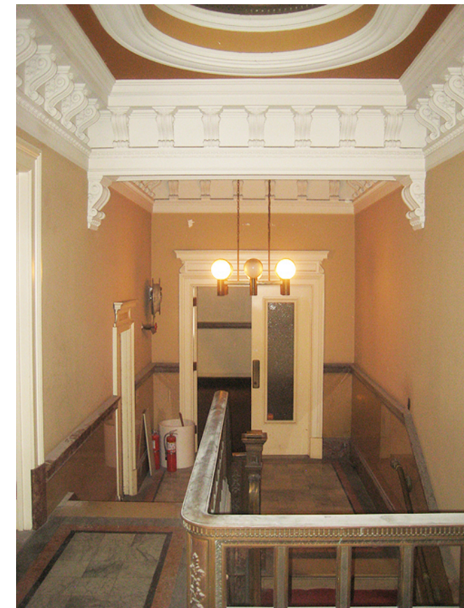
A: View of South stair hall looking at entry to 2nd floor office suite.
