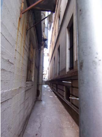
Figure 13. North facade. Source: KVP 2009.
