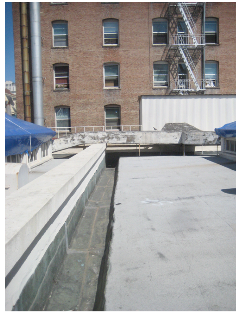
A: View across roof to mechanical penthouse. New metal walkway and north stair penthouse to be built in this location.
