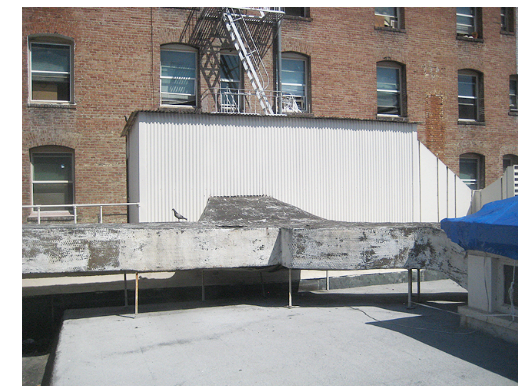
A: View of existing mechanical penthouse
