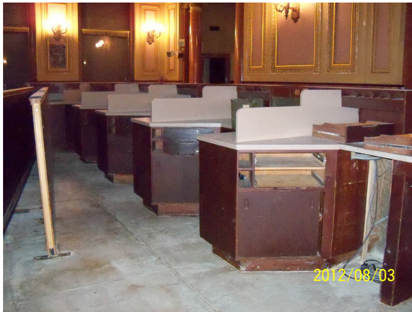
Figure 1. Plywood and Formica counter additions Source: Christopher VerPlanck
