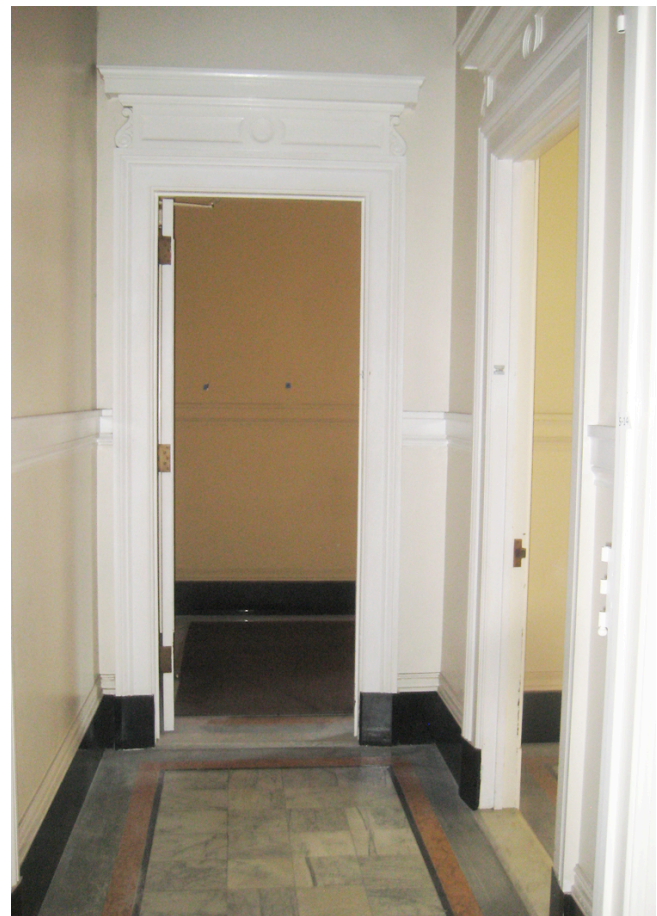
D: View of hallway to doorway in photo C.
