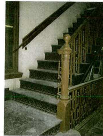
D: VIEW OF WINDOW TO BECOME WEST EXIT DOOR FROM NORTH STAIR HALL
