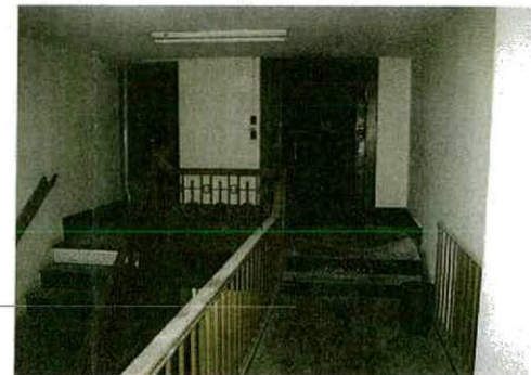
B: LANDING AT MEZZANINE LEVEL
