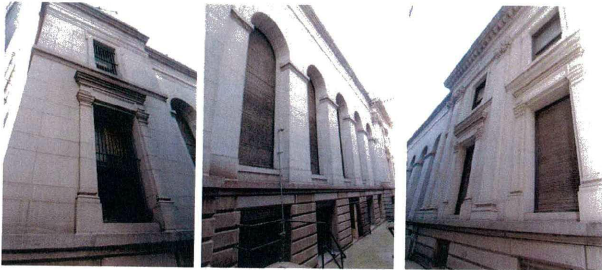
Figure 12. Details of west facade. From left to right: north bay, center bays and south bays.
