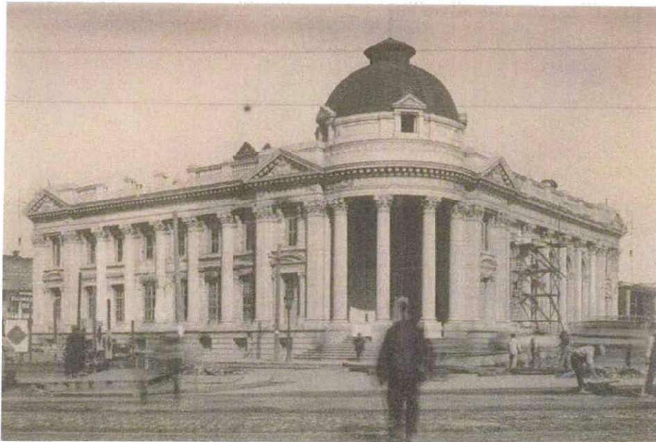
Item 19. Hibernia Bank Building during reconstruction, n.d. Source: Bancroft Library, University of California, Berkeley.
