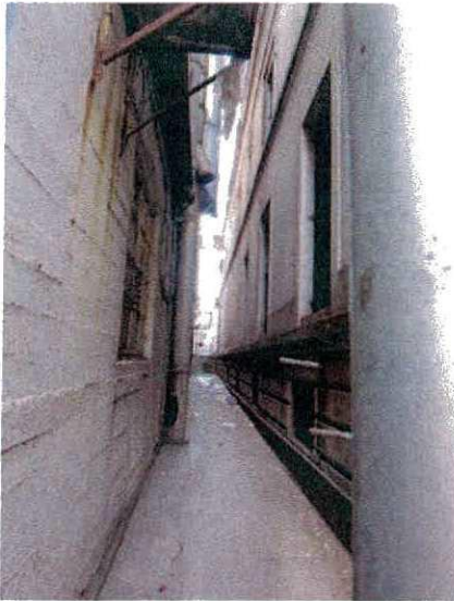
Figure 13. North facade. Source: KVP 2009.
