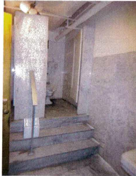
Figure 27. West Women's Toilet (B-29) located in the basement. Source: KVP 2009.
