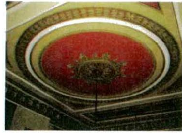
A: View of ceiling in SW Meeting Room.
