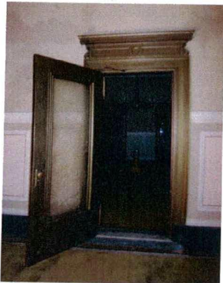
Figure 49. Typical partially glazed painted sheet metal door with painted sheet metal surround and cornice. Source: KVP 2009.
