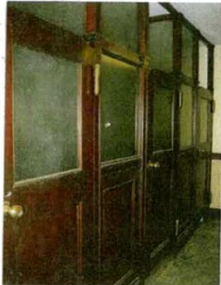
B: View of interior of historic safe deposit box viewing rooms.
