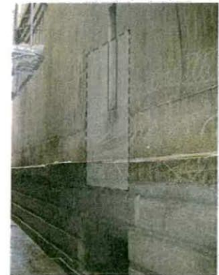
E: AREA OF MATERIAL TO BE CUT FOR NEW NORTH EXIT AT EAST SIDE OF STAIR HALL. MATERIAL TO BE RETAINED ON SITE FOR POSSIBLE REUSE. SEE PAGE 6 FOR STORAGE LOCATION. UPPER AREA OF LANCET WINDOW TO BE INFILLED WITH GRANITE RETAINED FROM CUT OPENING.
