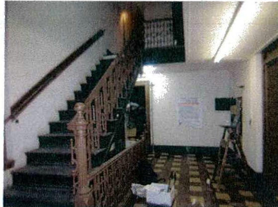
Figure 29. North Stair (F-3) located on the first floor. Source: KVP 2009.
