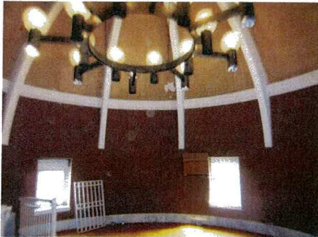
Figure 46. Dome Room (S-20) located at the penthouse level. Source: KVP 2009.
