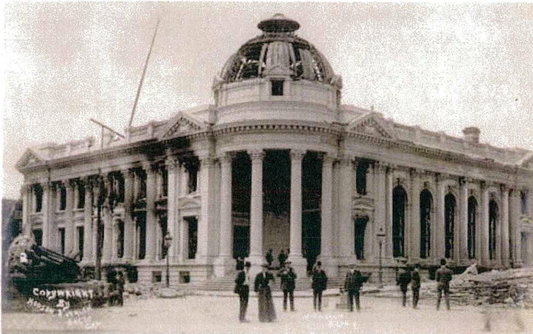
Item 17. Hibernia Bank Building, 1906. Note smoke damage at left dome beginning to be reconstructed. Source: San Francisco History Center, San Francisco Public Library.
