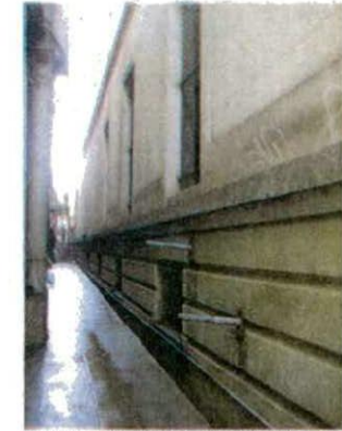
C: VIEW OF NORTH EXIT ALLEY INDICATING LOCATION OF EFFECTED AREA.
