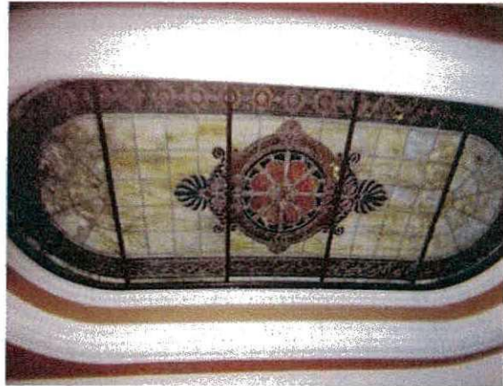
Figure 43. Detail of skylight in Stair Hall (S-10) located on the second floor south. Source: KVP 2009.
