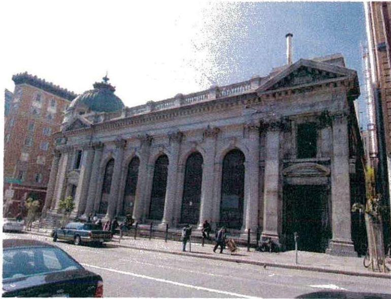
Figure 9. East facade facing Jones Street. Source: KVP 2009.
