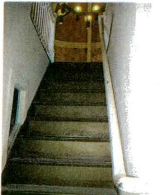
H: View of upper stair to Dome Room beyond. Access door at left reveals the granite and brick construction of the rotunda entry dome.
