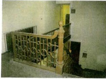
A: Walkway to Mezzanine storage to be removed and door to storage room to be infilled with new concrete shear wall.
