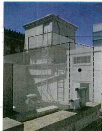
New elevator penthouse New east hall F: View of location of new east hall. Small skylight and vent to be removed. Elevator penthouse to be reconstructed.
