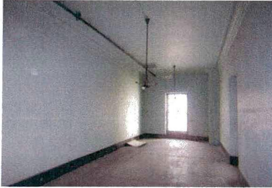
Figure 37. File Storage Room #1 (S-1) located on the second floor north. Source: KVP 2009.
