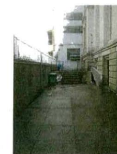
C: View of west exit alley
