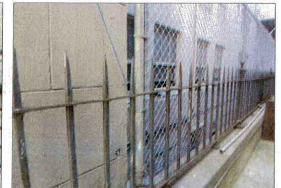
FENCE ALONG WEST PROPERTY LINE
