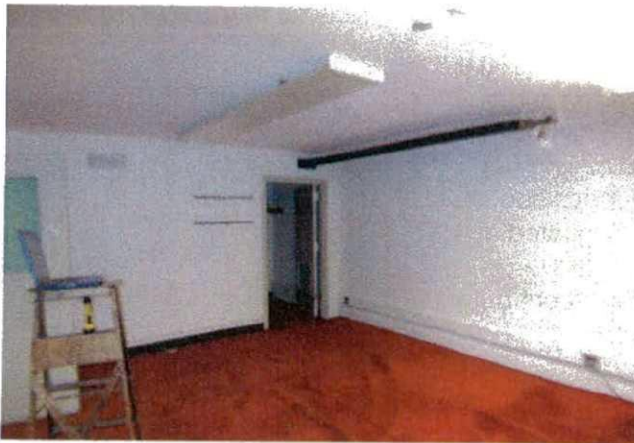
Figure 23. Office #2 (B-8) located in the basement. Source: KVP 2009.
