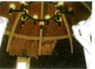
D: View of chandelier and ceiling of Dome Room. Renovations to room from 1977 to be removed.
