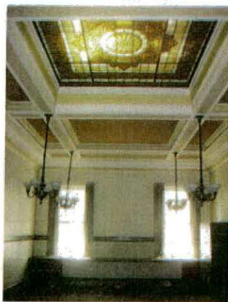
E: View of Waiting/Reception Room in 2nd Floor offices. This room will remain intact with the light fixtures to be retained.
