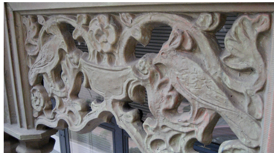
Decorative sheet metal below balconies
