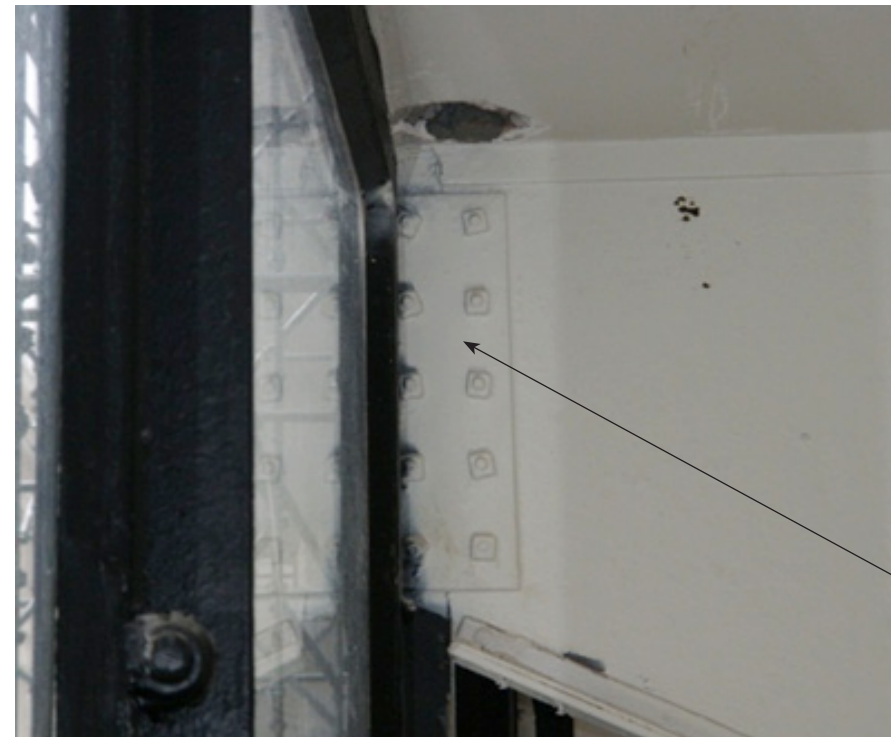
existing bolt plates connect T-mullion to outrigger plates; additional outriggers and bolt plates will match existing design
