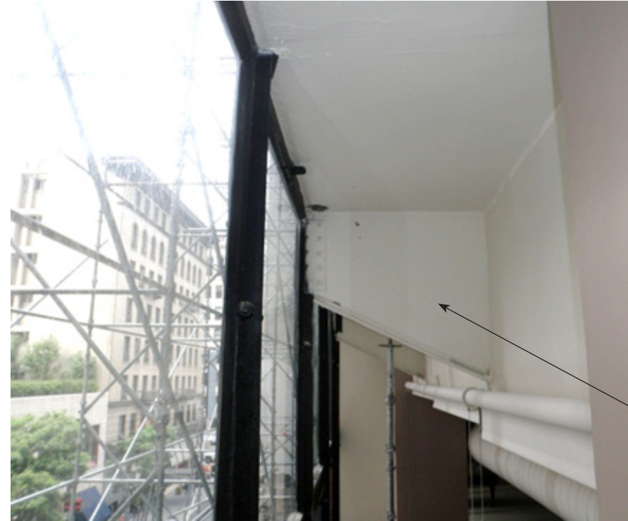
existing outriggers at non-balcony levels on 4th, 5th, and 6th floors; additional outriggers will be added for structural reinforcement of curtain wall
