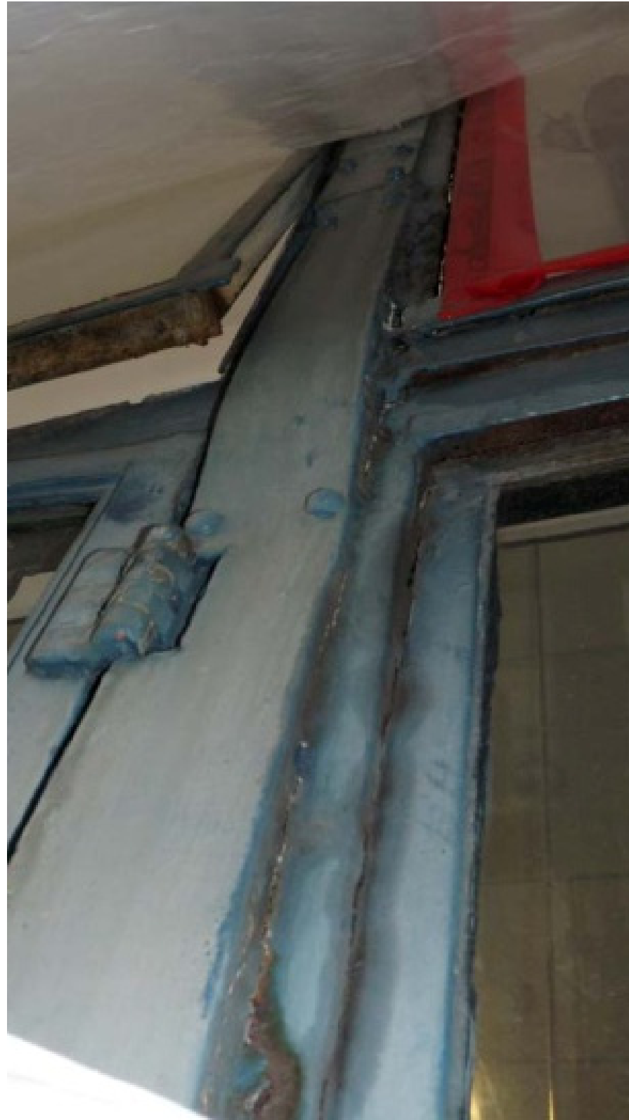
Vertical cover plate at curtain wall
