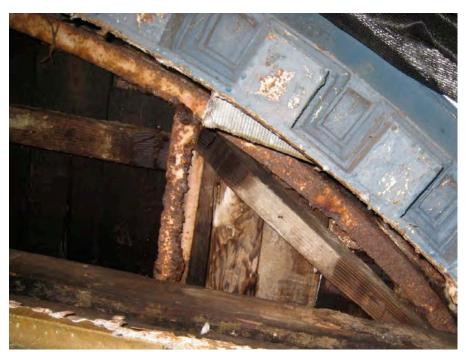
Deterioration at steel framework supporting a balcony
