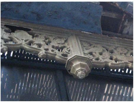
Deterioration at a frieze panel
