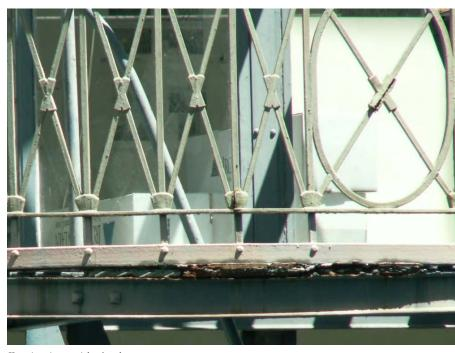
Deterioration at picket bracket
