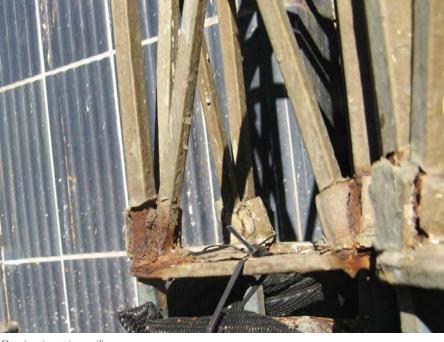
Deterioration at iron railings
