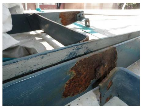
Deterioration at rung welded connections
