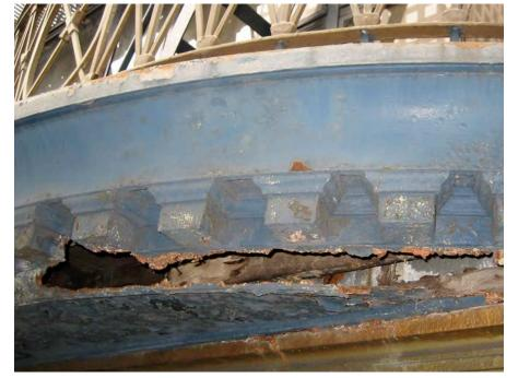
Deterioration at underside of balcony
