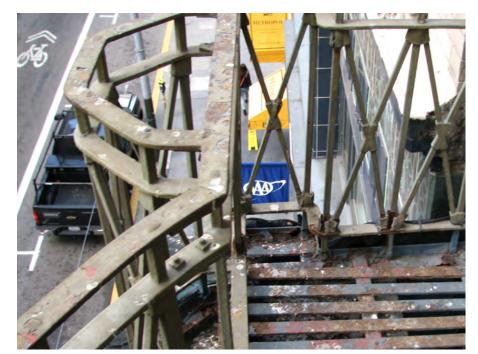
Deterioration at railings
