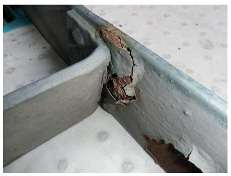
Deterioration at rung welded connections
