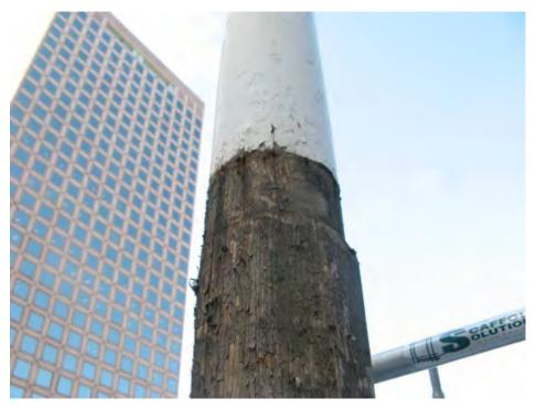
Figure 2: Detail of flagpole showing existing condition and color.
