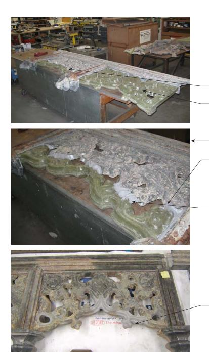
Panels that have between 5% and 50% panel deterioration will be repaired with a fiberglass patch. Two panels were mocked-up.
