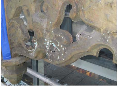
Deterioration at a frieze panel
