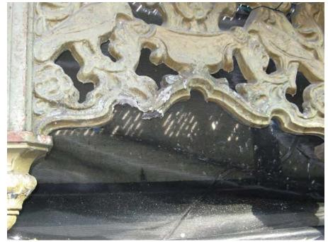
Deterioration at a frieze panel
