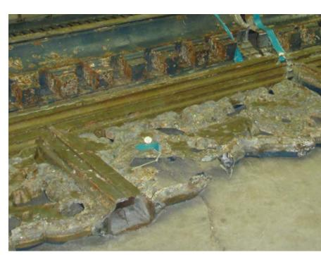
Deterioration at a frieze panel
