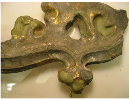
Figure 2: Section of tracery removed from lower (second story)cornice.
