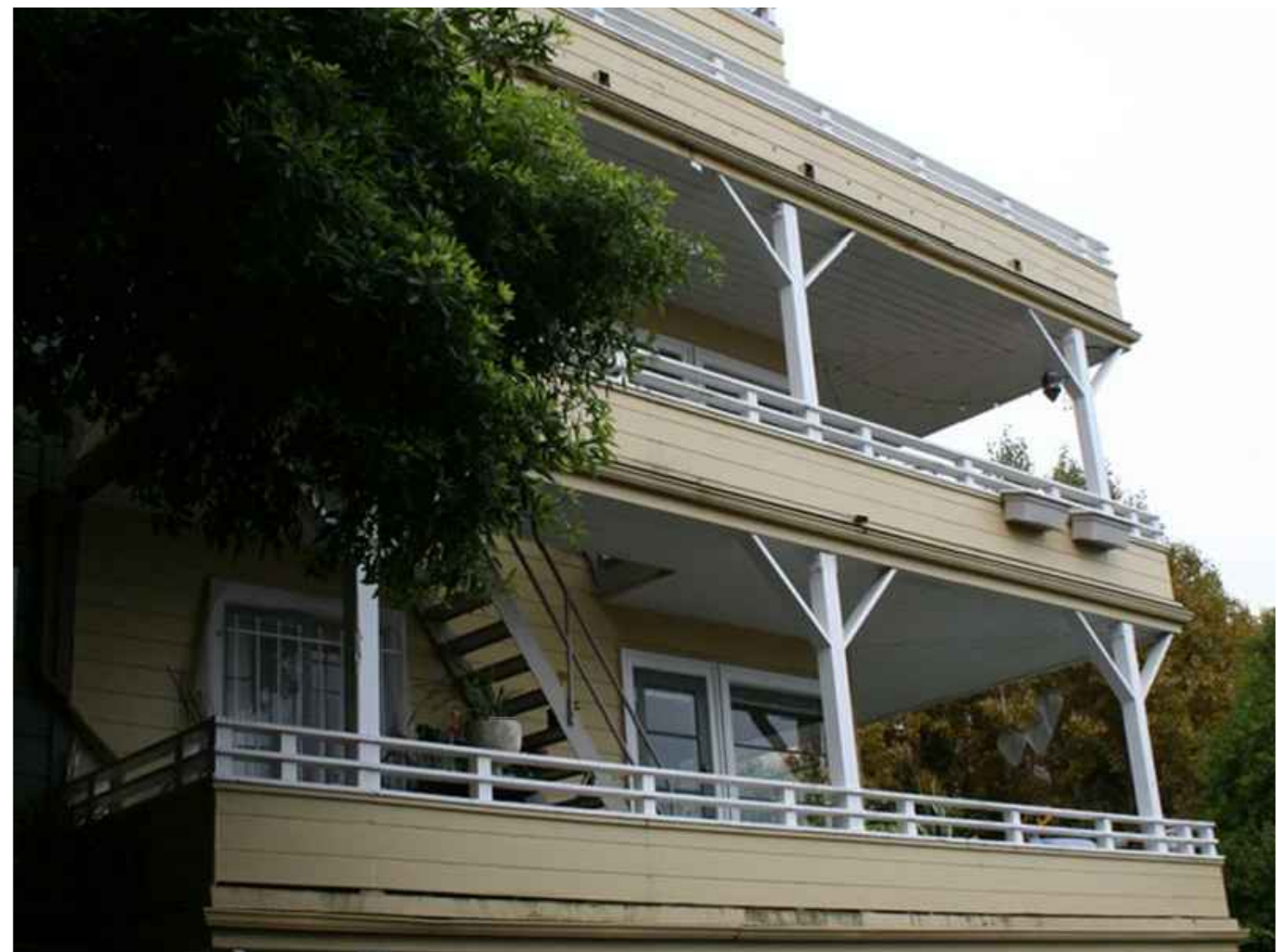
VIEW TOWARD ADJACENT BUILDING'S RAILING
