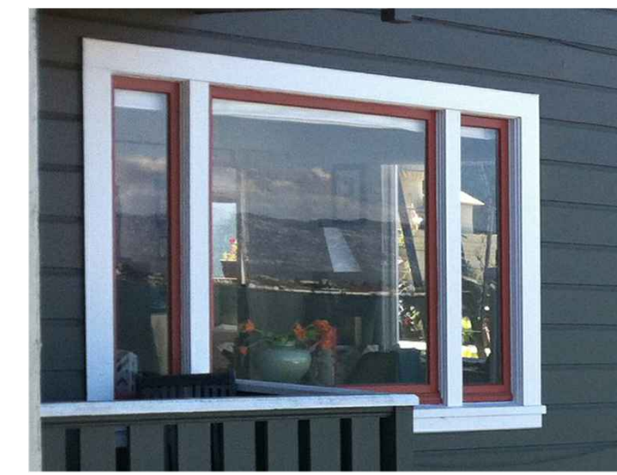
VIEW OF EXISTING WINDOW @ FOURTH FLOOR
