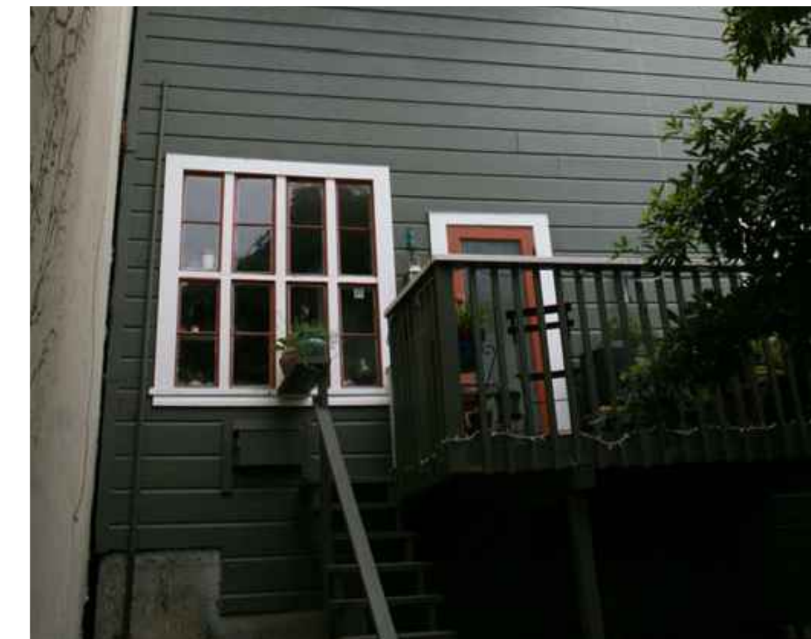
VIEW OF EXISTING SIDING
