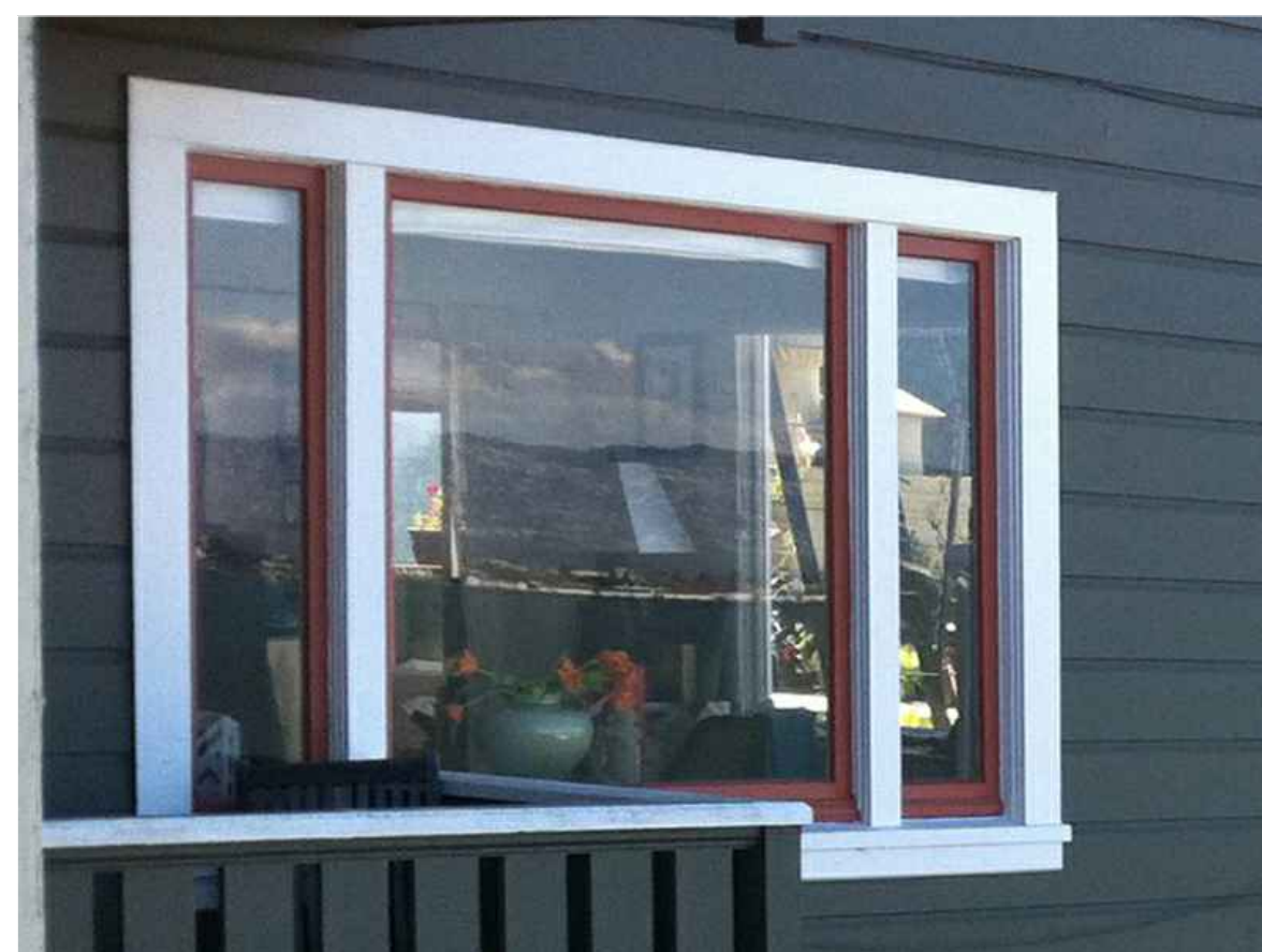
VIEW OF EXISTING WINDOW @ FOURTH FLOOR
