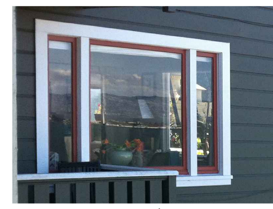
VIEW OF EXISTING WINDOW @ FOURTH FLOOR
