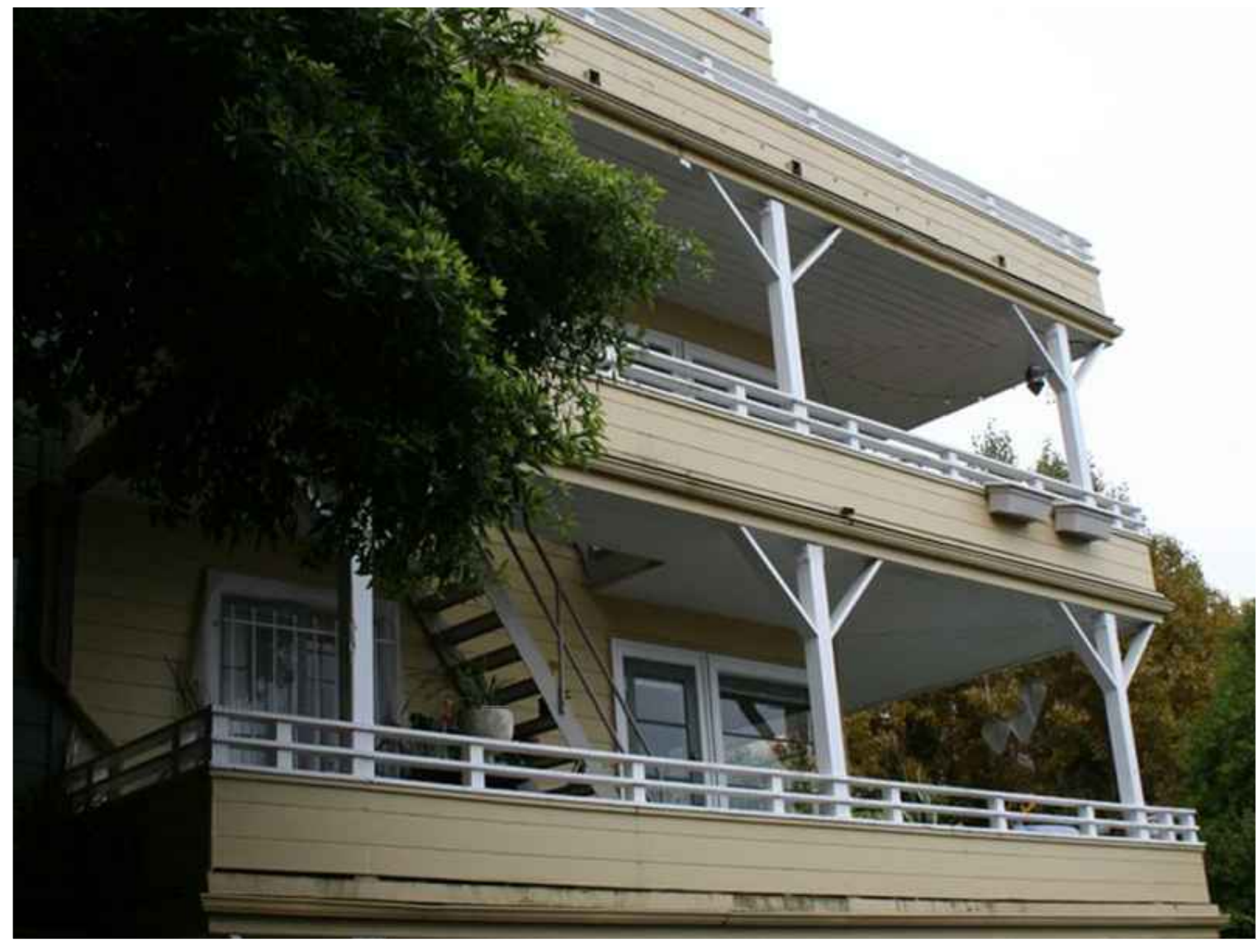
VIEW TOWARD ADJACENT BUILDING'S RAILING
