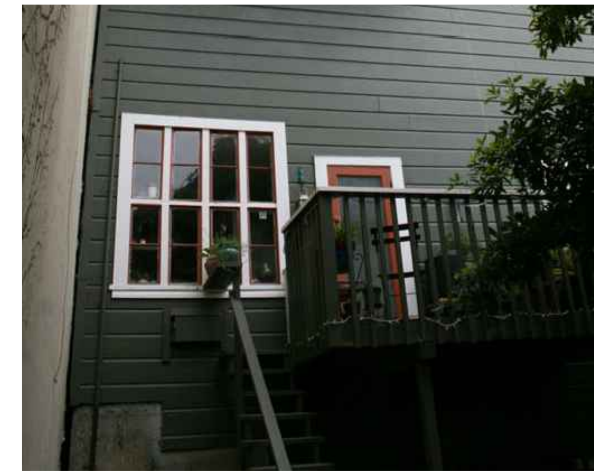
VIEW OF EXISTING SIDING
