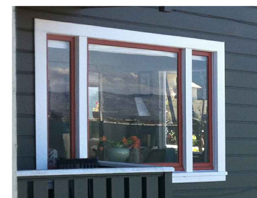
VIEW OF EXISTING WINDOW @ FOURTH FLOOR
