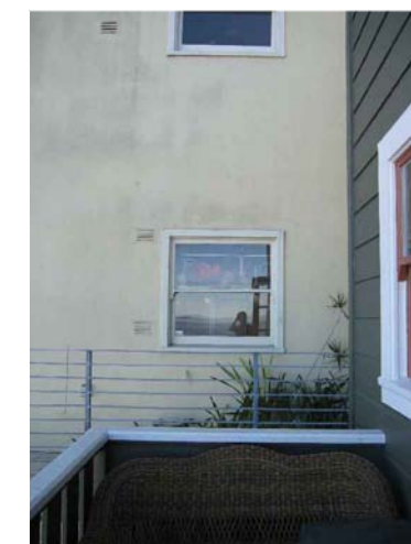
VIEW TOWARD ADJACENT BLD. (LOT 040/045) FROM FOURTH FLOOR
