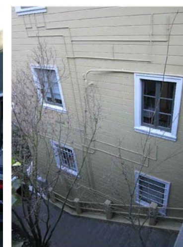
ADJACENT BUILDING VIEW FROM BRIDGE
