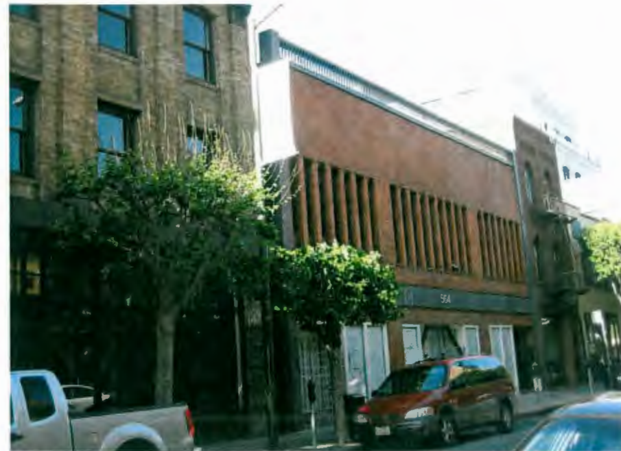
560-564 Pacific Avenue, looking northeast along Pacific Avenue
