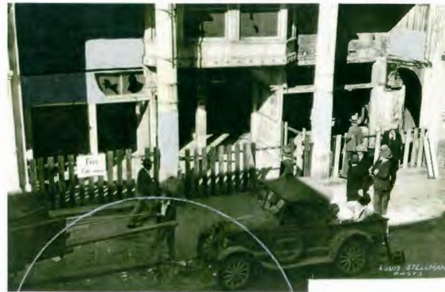
The Hippodrome reconstruction, 1934. Source: San Francisco Historical Photograph Collection
