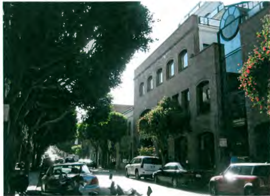
Infill construction on Pacific Avenue (north side) between Montgomery and Kearny streets.
