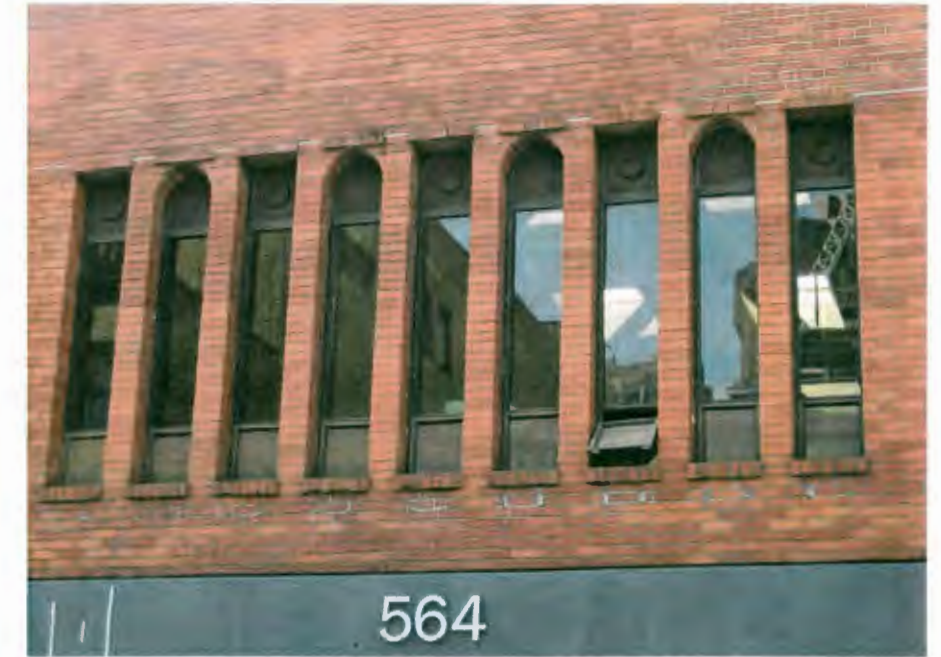
560-564 Pacific Avenue, detail of narrow second floor windows
