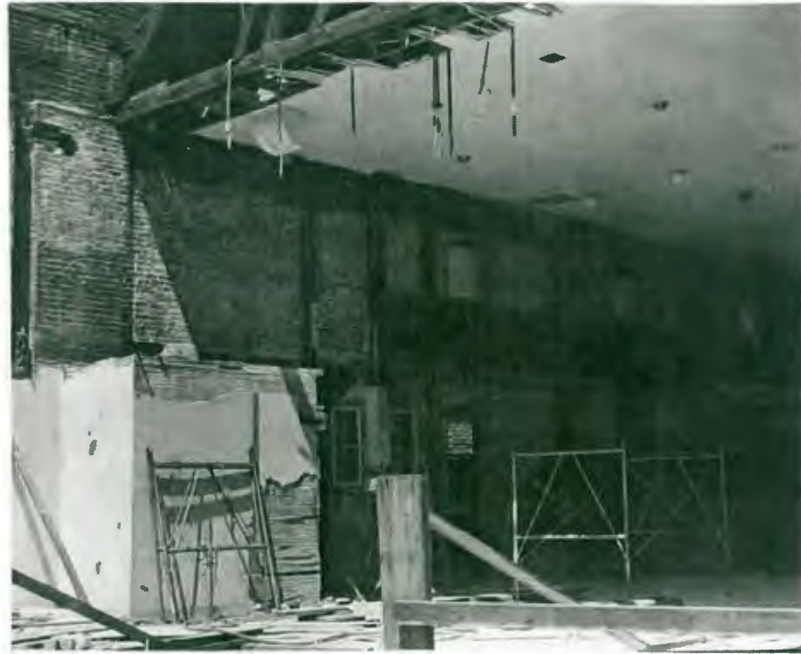
Demolition of facade, ca. 1965. Source: Beverly Willis, www.beverlywillis.com
