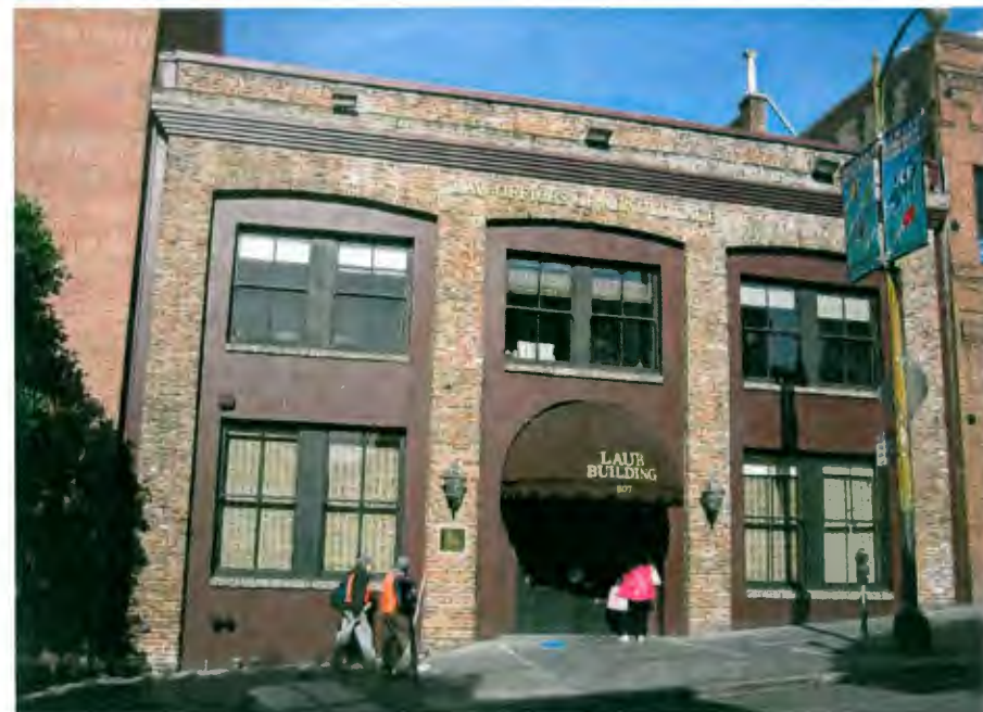
807 Montgomery Street, with stucco infill and compatible replacement windows
