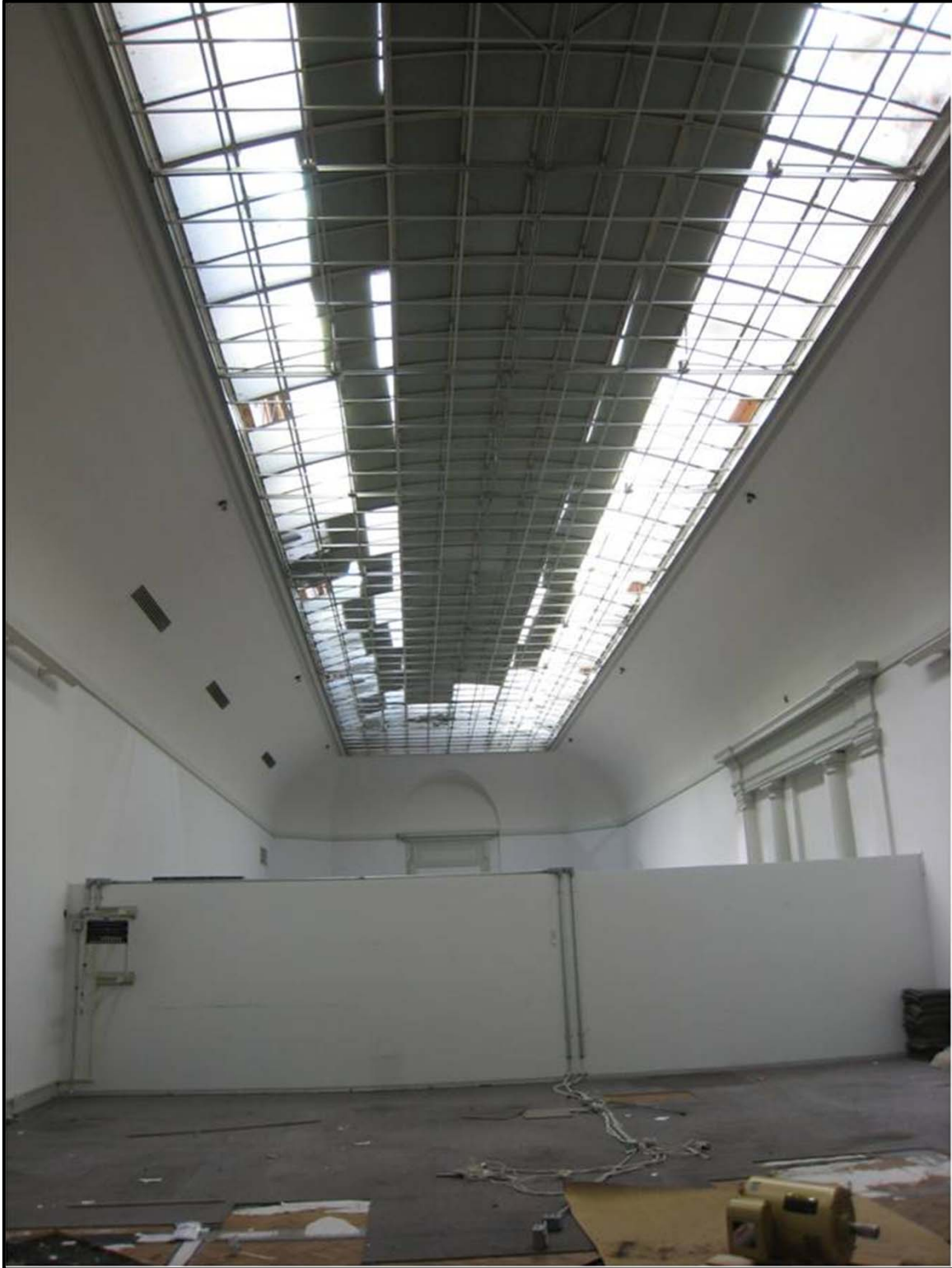
Veterans Building, 4 th Floor, View of Laylights
