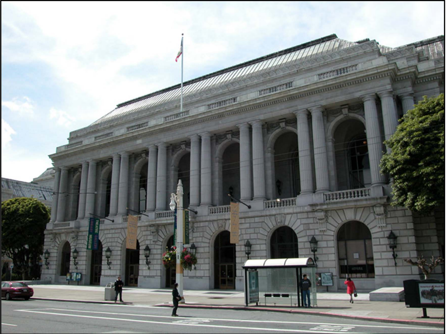
View of Veterans Building along Van Ness Avenue
