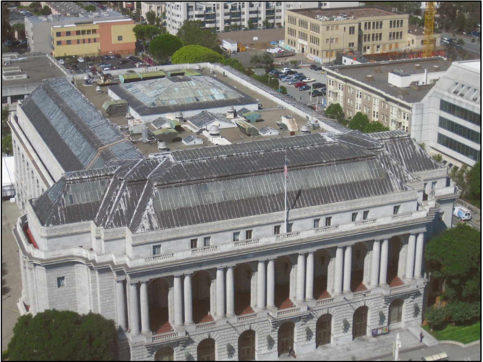
View of Veterans Building Roof
