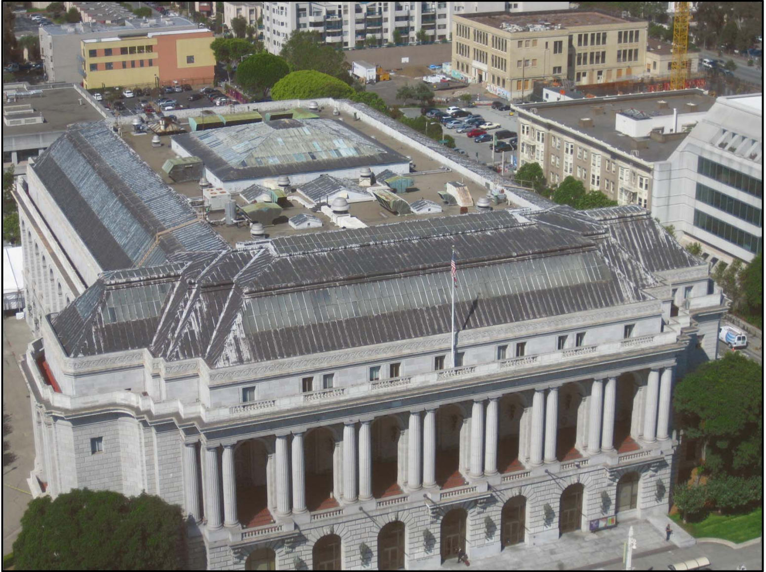
View of Veterans Building Roof
