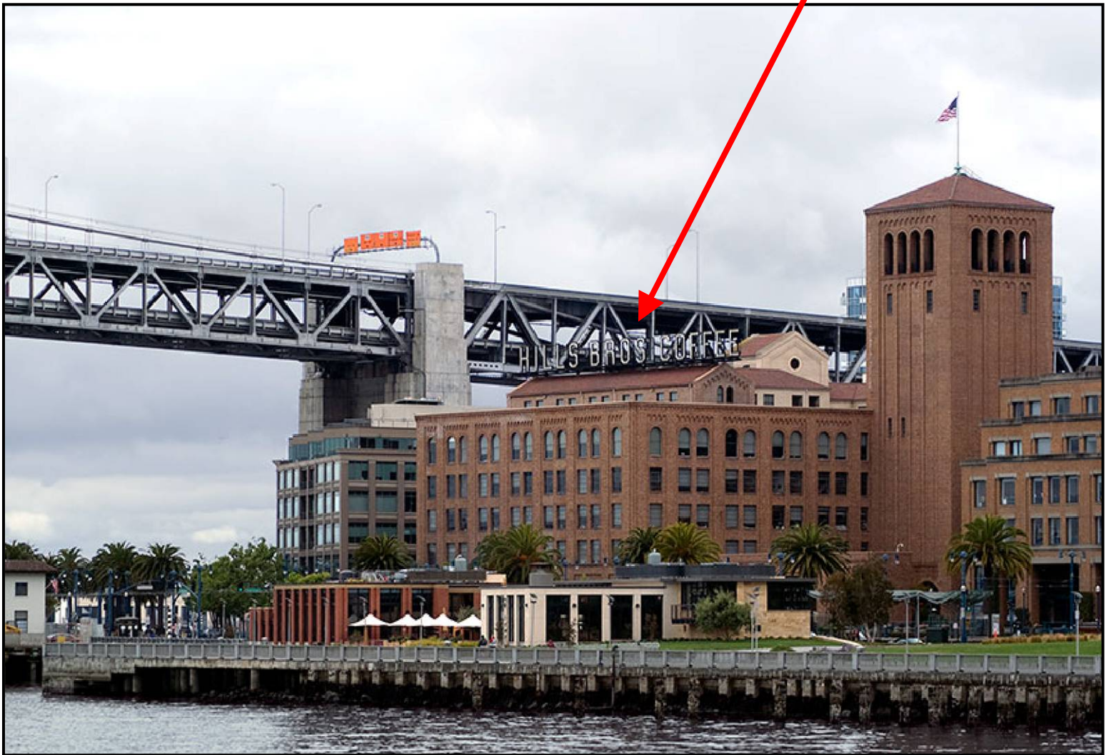
2 Harrison Street (View from Pier 14)
