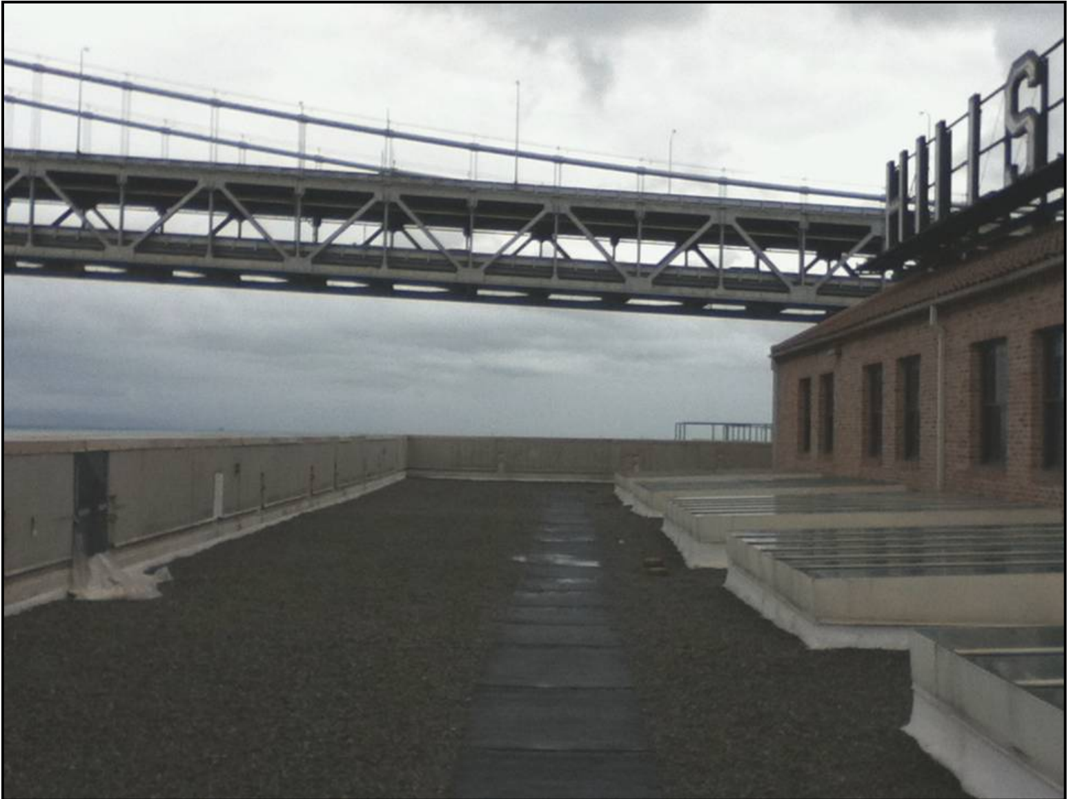
2 Harrison Street (Site of Future Roof Deck)
