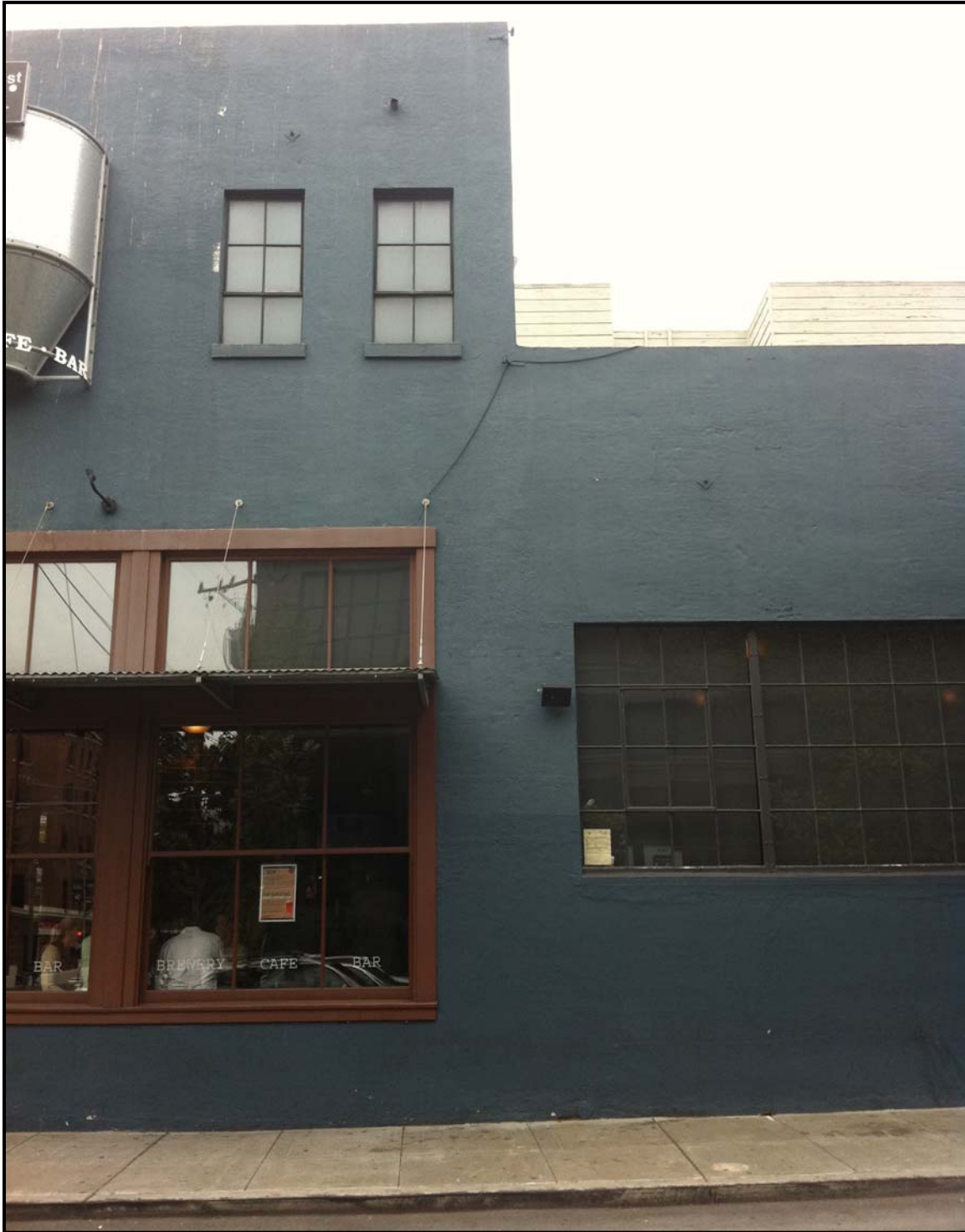
563 2 nd Street, DeBoom Street façade, Area of Work
