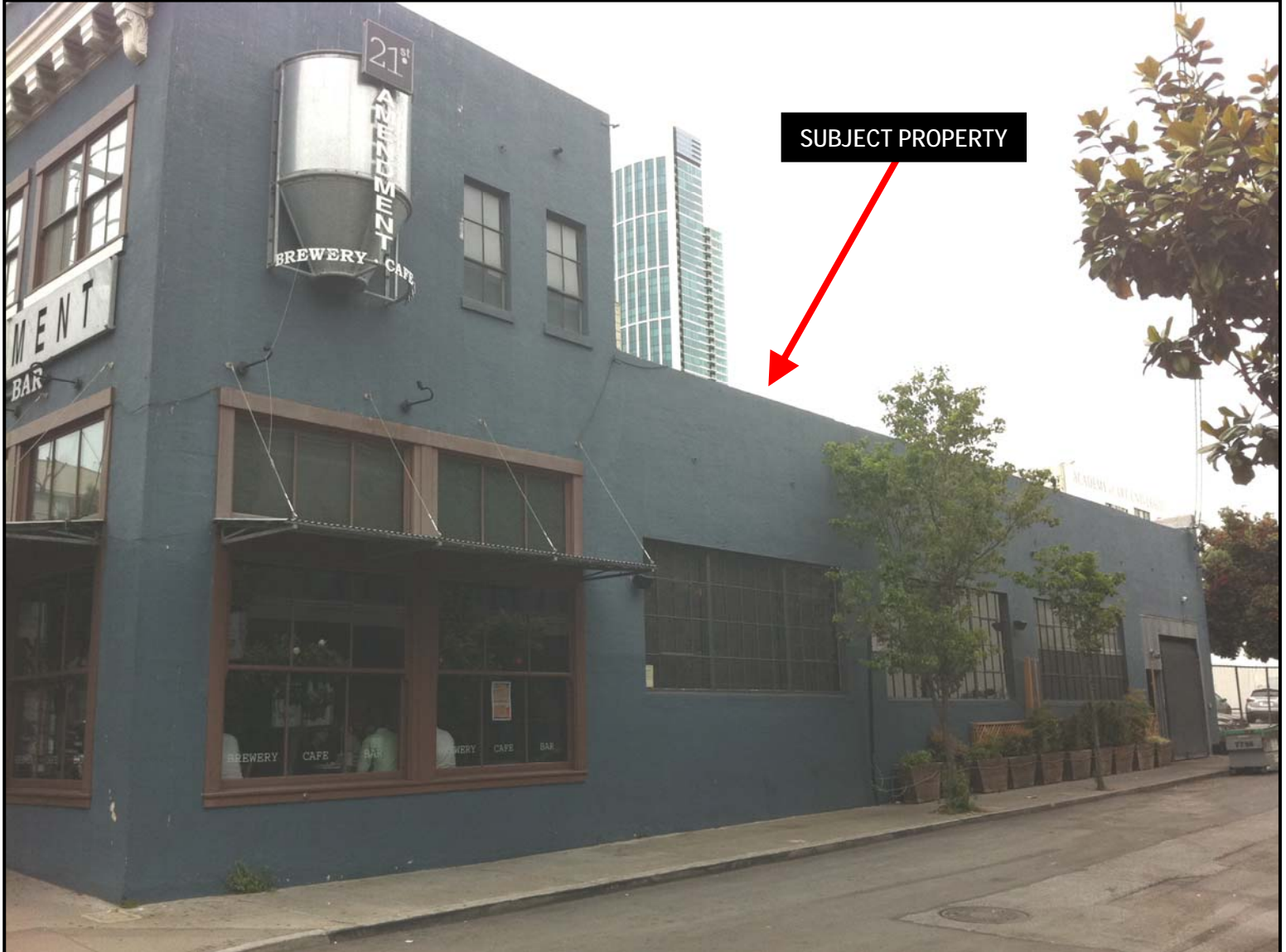
563 2 nd Street, DeBoom Street Facade
