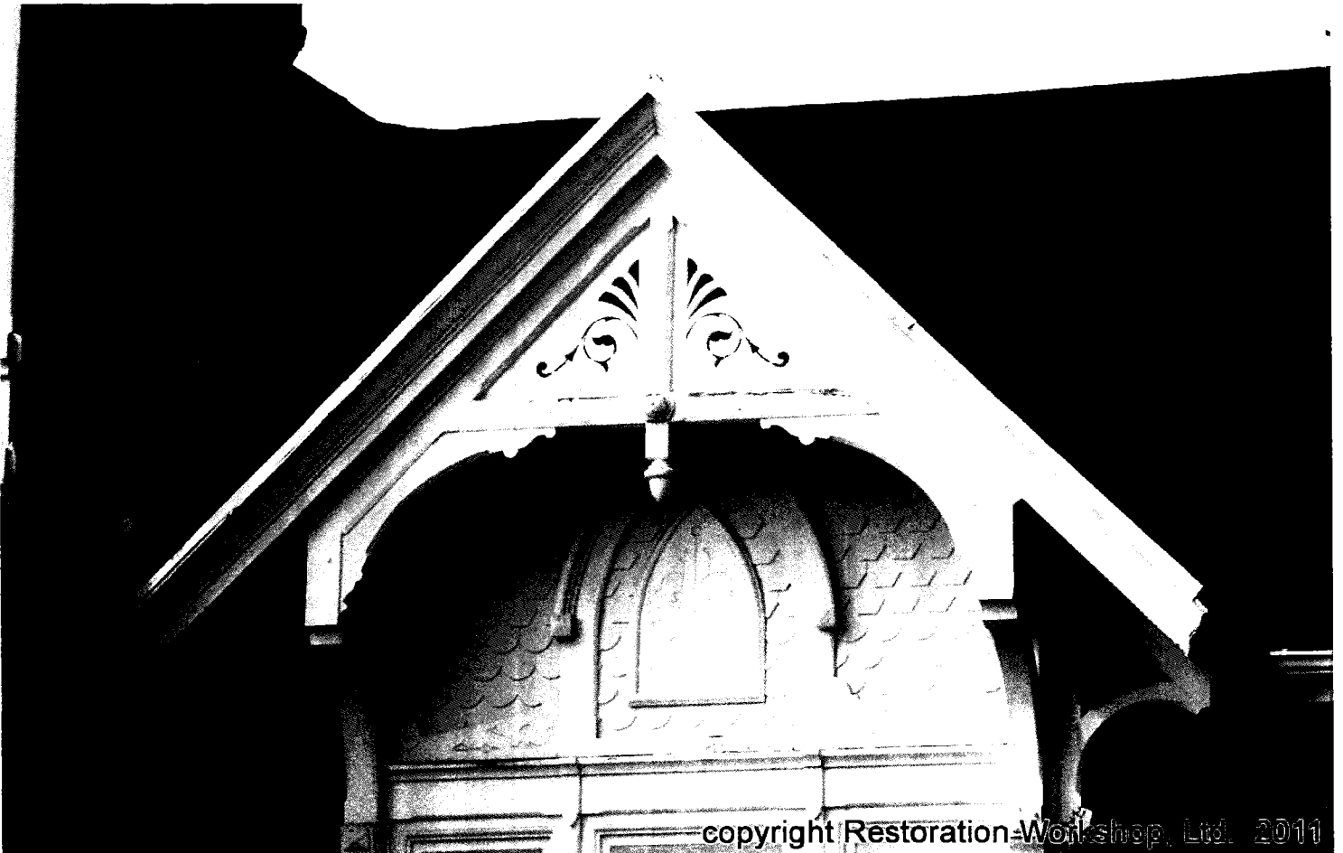
Gable over dining room bay (eastern facade)
