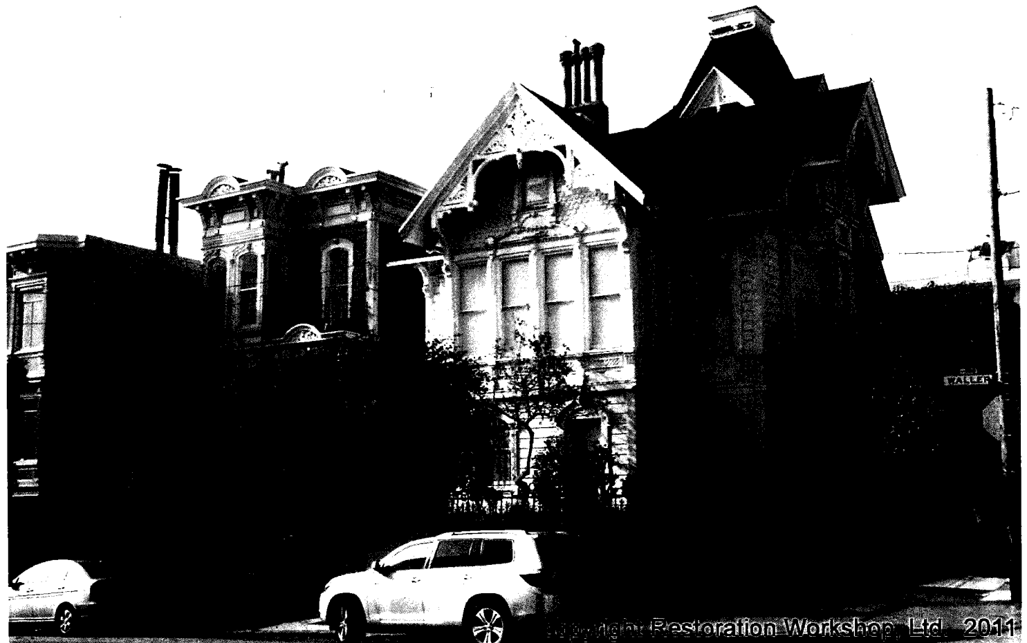
201 Buchanan: South Facade
