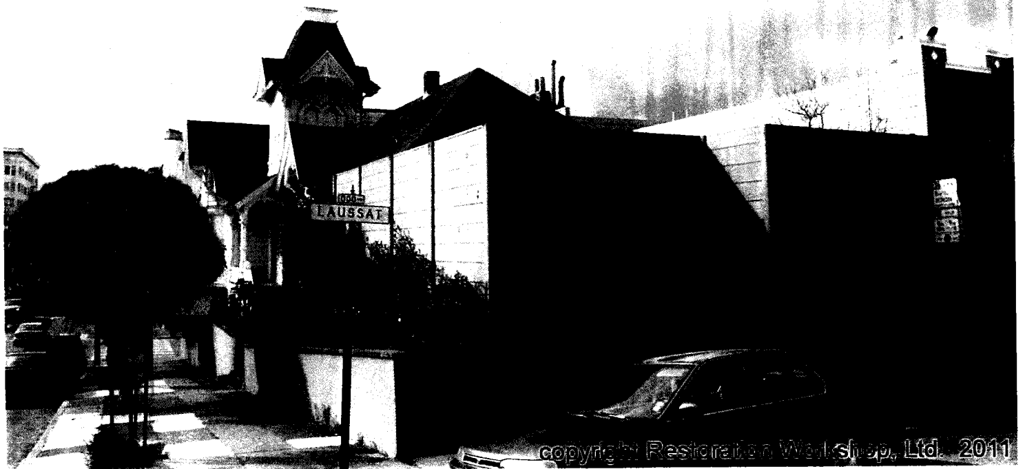
201 Buchanan: South Elevation, Non-historic addition and rear fence.
