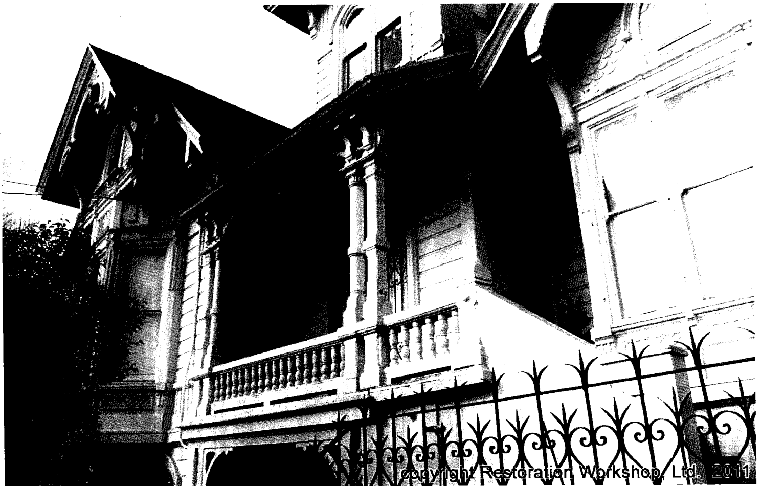
Eastern facade: Porch and main entrance.
