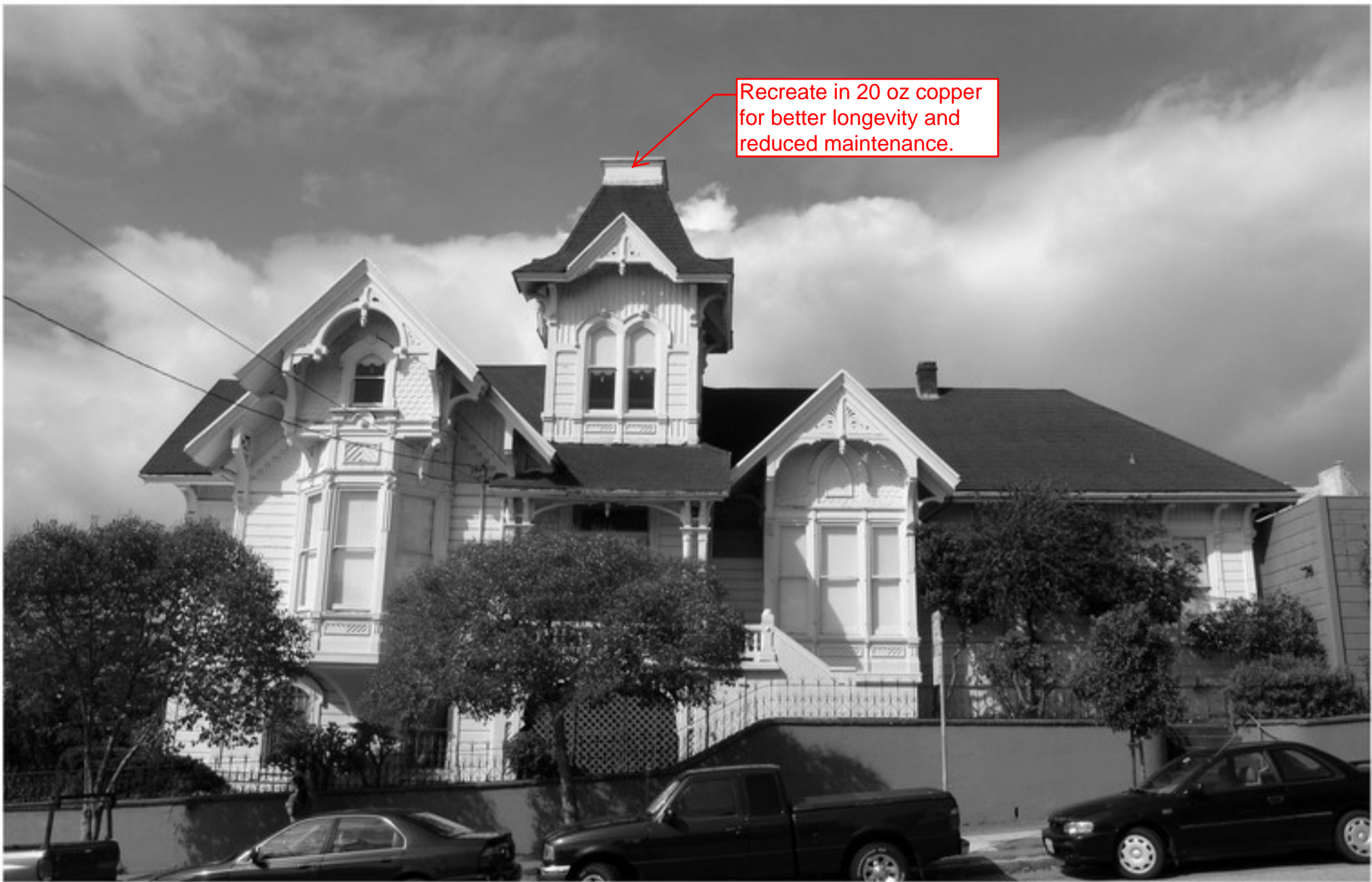
201 Buchanan Street: Eastern facade
