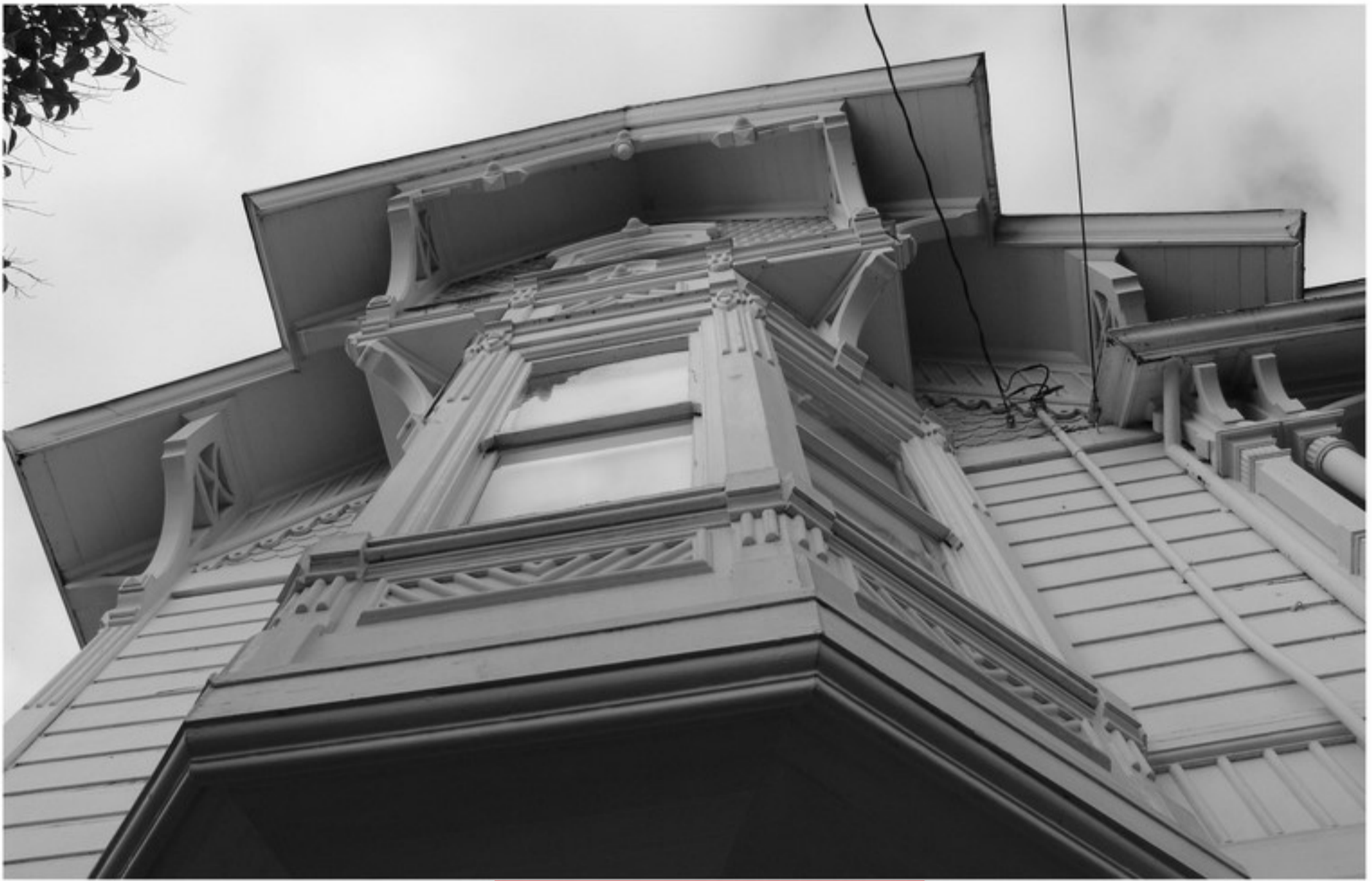
Front parlor bay and gable (eastern facade)
