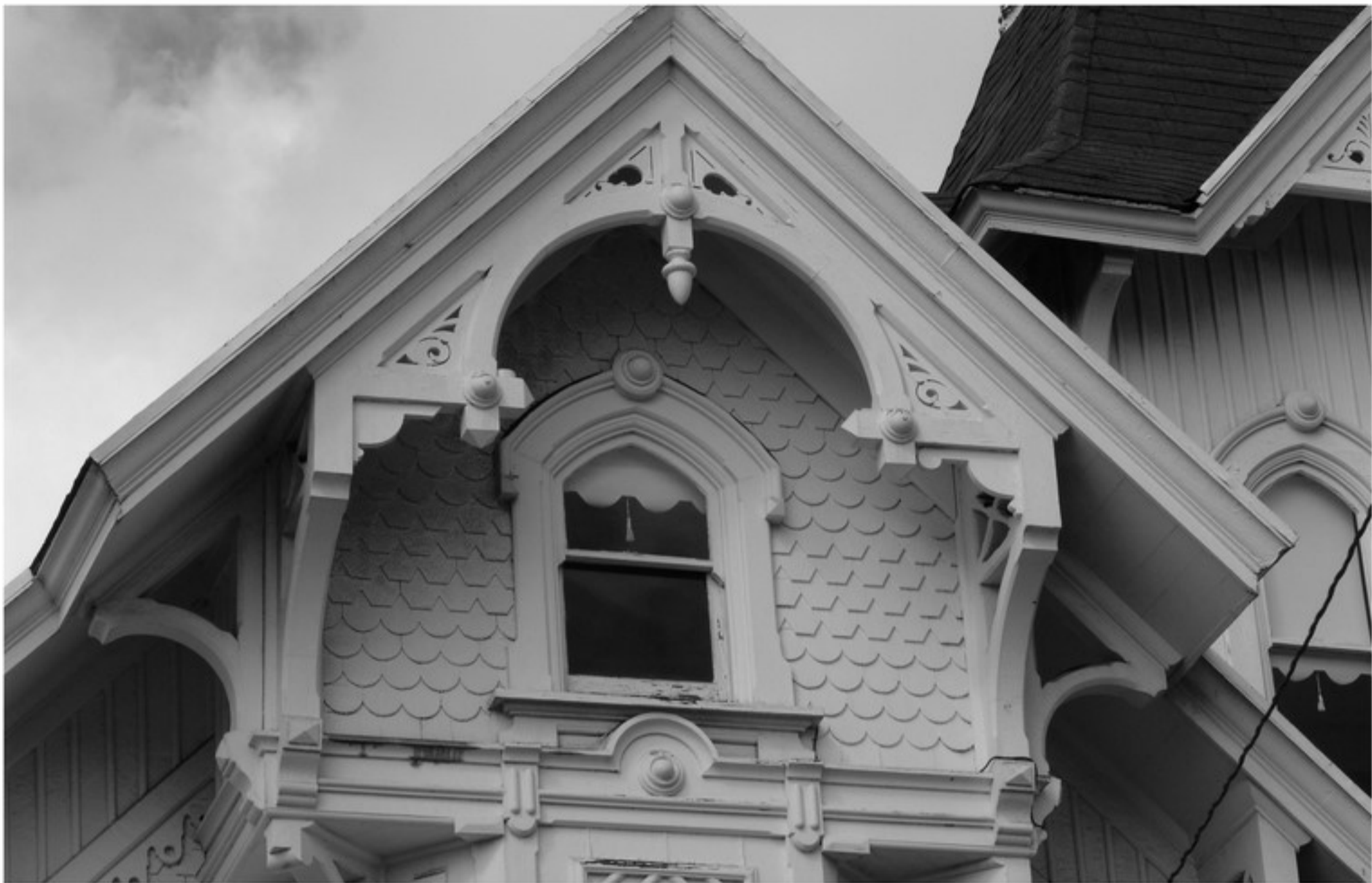
Gable over front parlor Bay (eastern facade)
