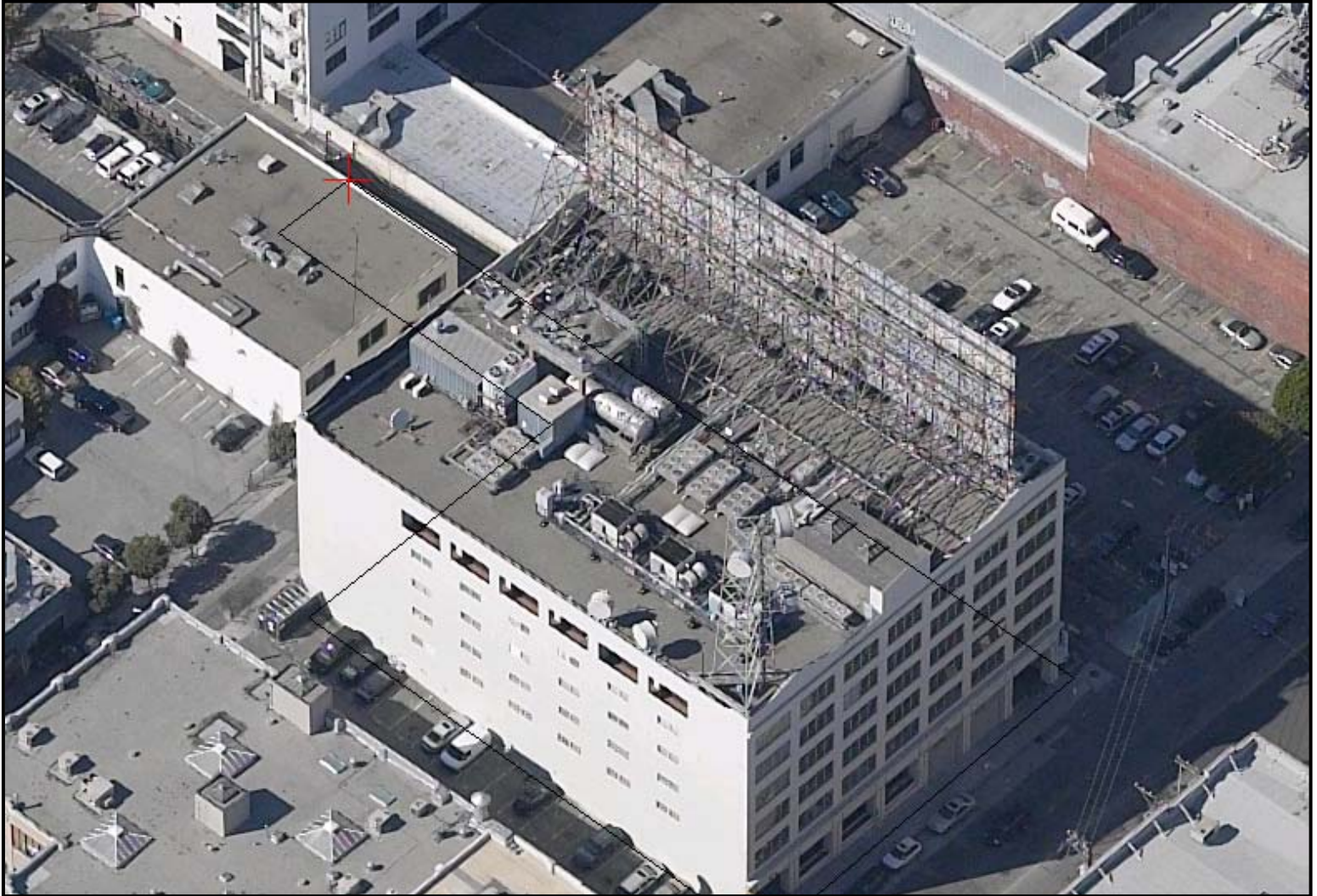
Detail of 274 Brannan Street Roof
