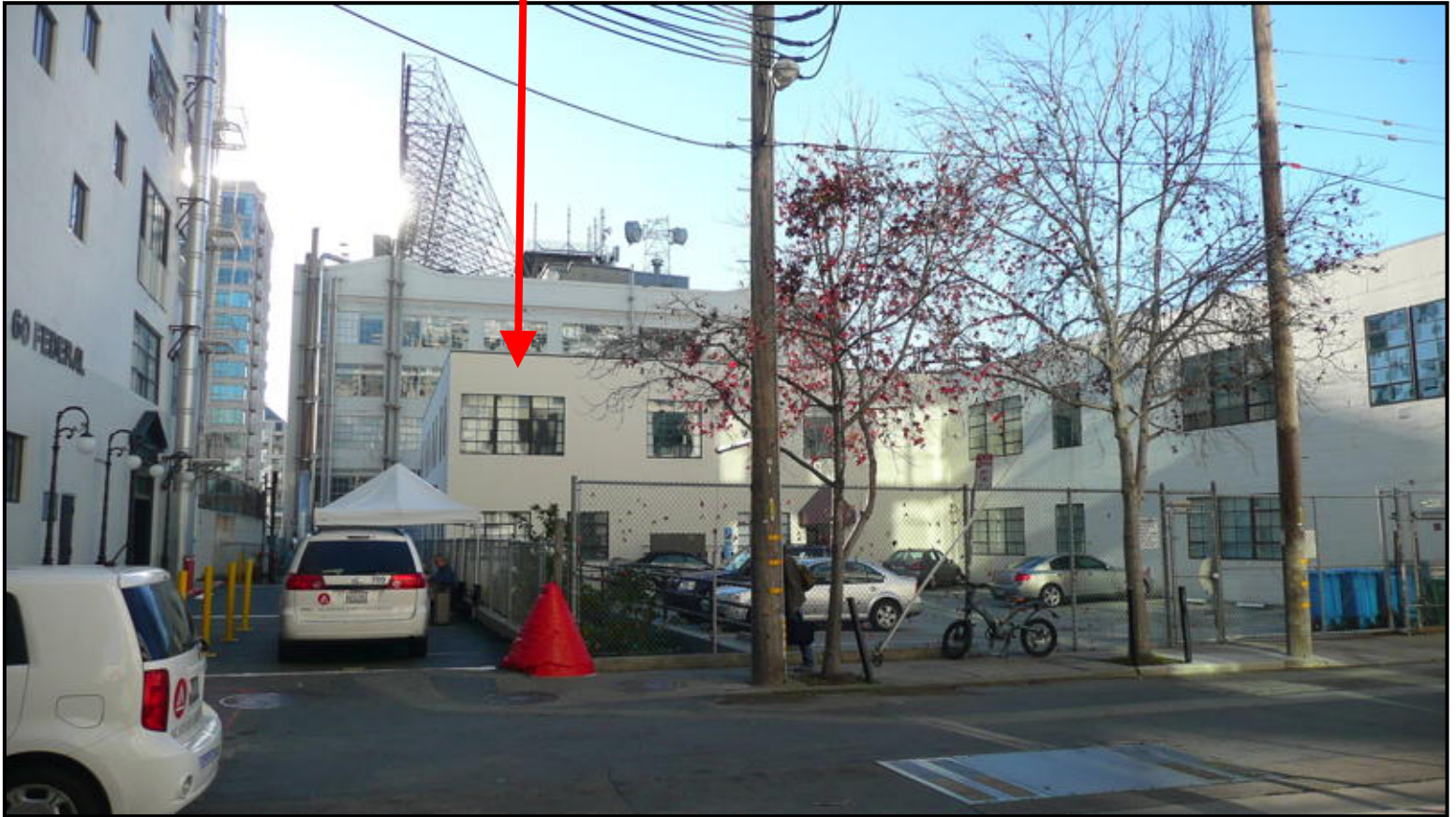
75 Federal Street, North Facade
