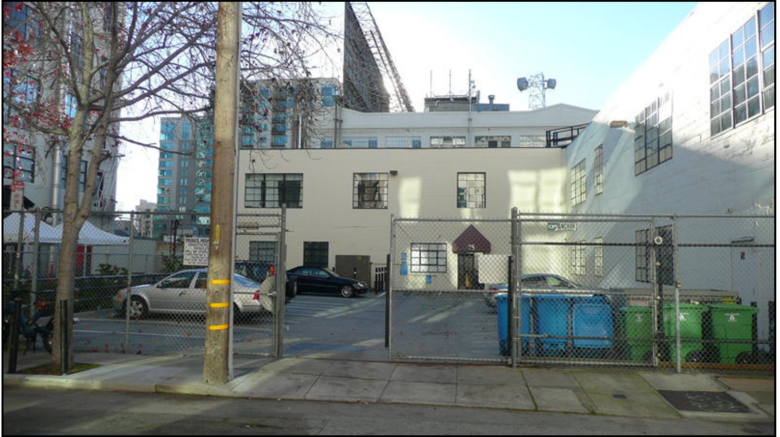
75 Federal Street, North Facade
