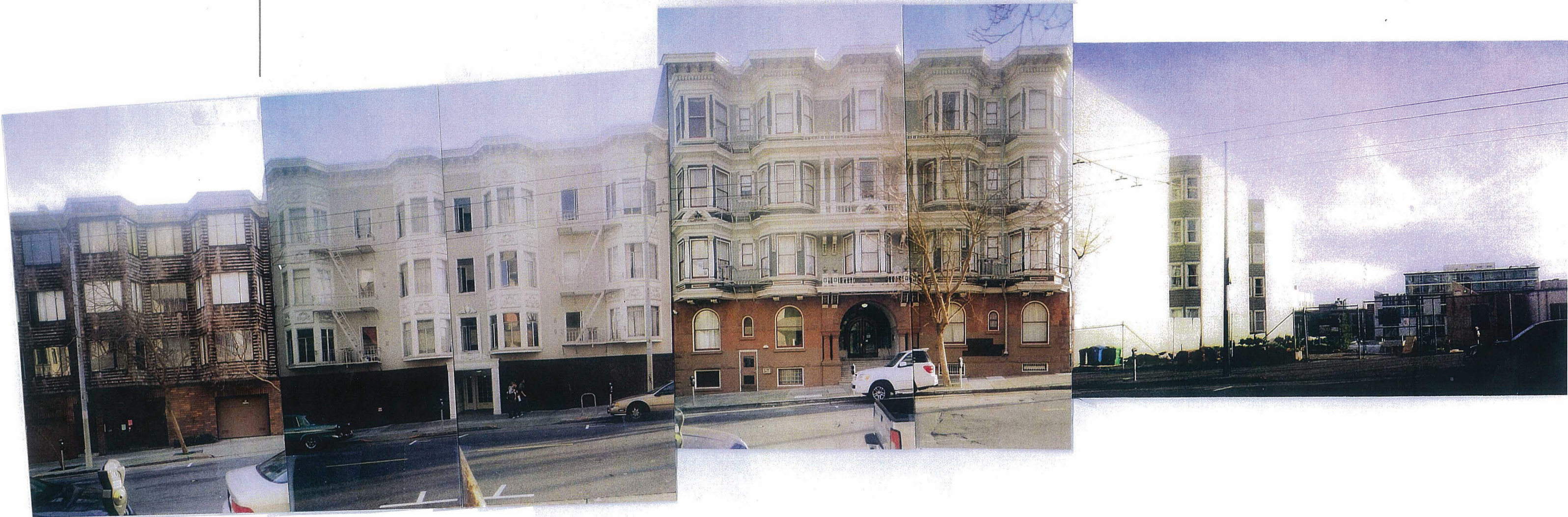
NORTH FACADES OF EDDY STREET BUILDINGS
