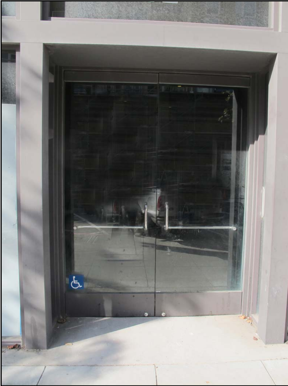
72 Townsend Street, Area of Work (Door Sign)
