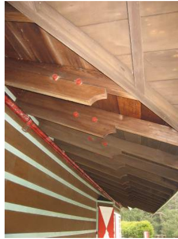
Left: Interior view of the boat room looking northeast. Right: Exterior view of sculpted rafter tails and overhanging eaves.
