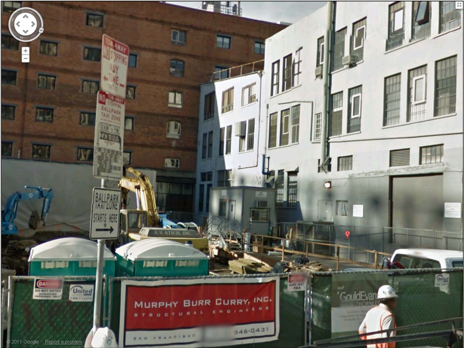
111 Townsend Street, View of Rear Façade
