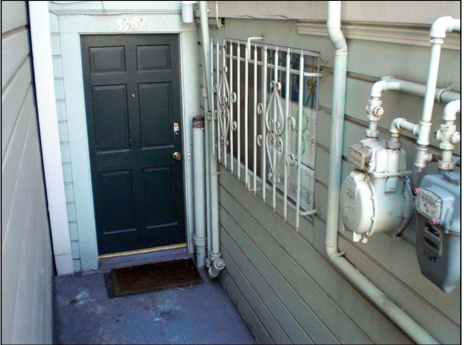
Subject Property, Site of Window Insertion on Side (East) Facade
