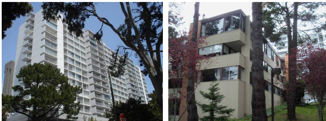
Left: 66 Cleary Court residential tower designed by Jones & Emmons (1964). Right: Across the street, at 85 Cleary Court, is a complex of six three-story, 12-unit buildings designed by Claude Oakland (1963). Common alterations include the enclosing and glazing of both the low-rise buildings and the tower. The middle-unit (right) retains its original open-air balcony. Photos: Aisha Rahimi; Mary Brown, San Francisco Planning Department
