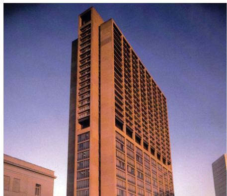
Fox Plaza Tower, 1390 Market. Photo courtesy of Cahill Contractors.
