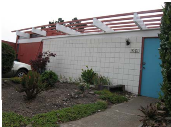
1021 Duncan Street. This block features a grouping of Claude Oakland designed Eichler houses. Photo: Mary Brown, San Francisco Planning Department
