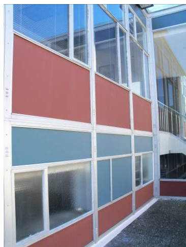
San Francisco Modern architect Francis Joseph McCarthy incorporated colored "Spandrelite" spandrel panels in the curtain wall of the (1956) International Brotherhood of Electrical Workers Local 6 building at 55 Fillmore Street. Photo: Mary Brown, San Francisco Planning Department.
