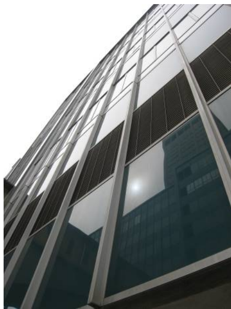
Detail of projecting mullions that vertically divide the massing of the (1968) California State Automobile Assoc. office building on Hayes Street. Photo: Mary Brown, San Francisco Planning Department
