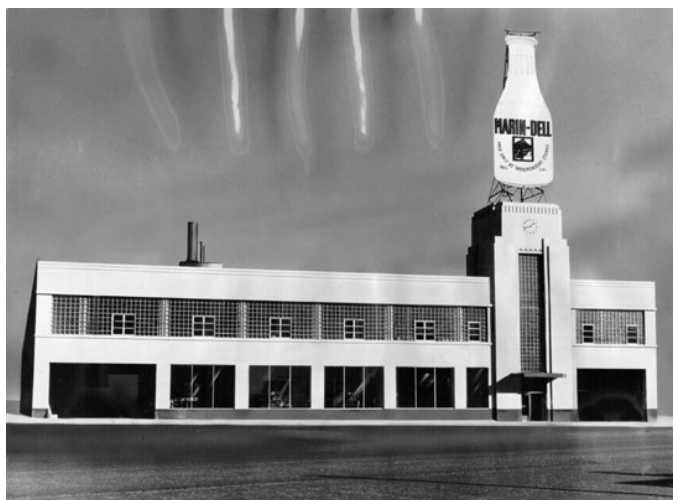
LEFT: The Marin Dairyman's Milk Company building incorporates key characteristics of the Moderne style including glass block walls, rounded overhang, banding at the roofline, and a stepped tower. Although the bottle sign was removed, the building retains physical integrity.
