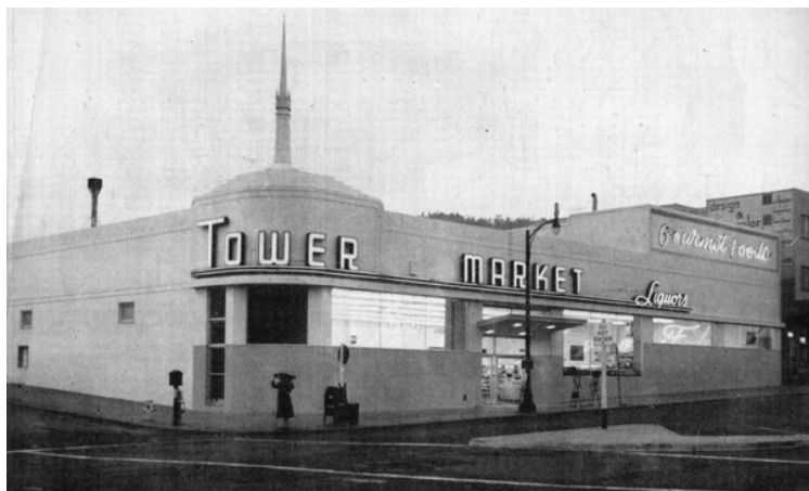
Left: Constructed in 1942 and remodeled in 1958 (pictured), the Tower Market anchored and grew a several-block retail strip in the Miraloma neighborhood. (Source: mtdavidson.org)
