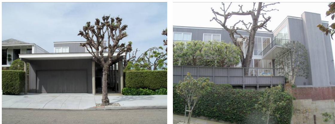
ABOVE. The Goldman House, 3700 Washington Street, designed by Joseph Esherick (1951). The L-shaped, box-like house is perched on a steep slope near Presidio Heights. Photos: Mary Brown, San Francisco Planning Department
