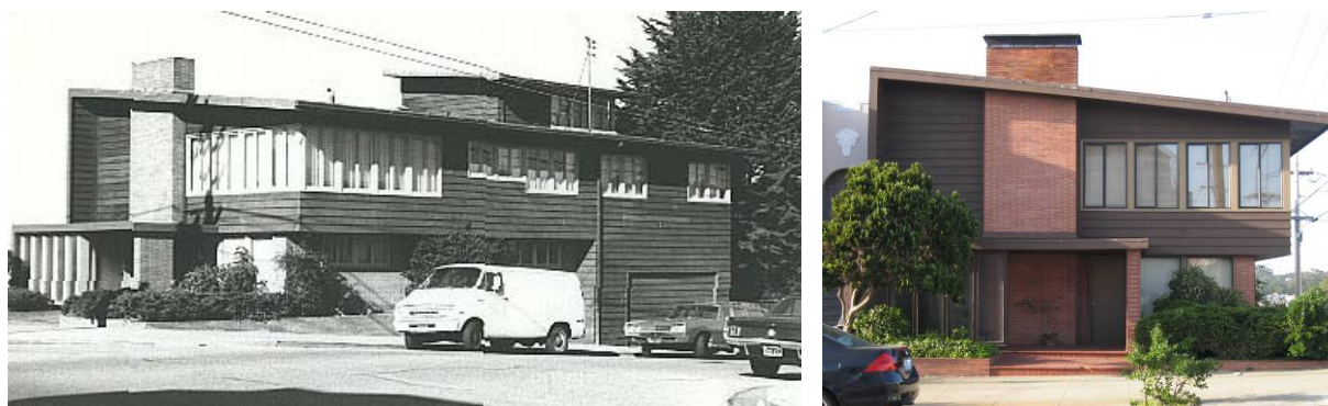
ABOVE: 2000 Kirkham Street is an unusual example of a Second Bay Tradition residence located in the Sunset District. It also features Midcentury Modern design elements, illustrative of the occasionally blurred distinction between Second Bay Tradition and Midcentury Modern design – many buildings reflect a hybridization of the two styles. The house was built in 1950 and designed by little-known architect Albert Richards. Aside from window replacement the building retains high levels of physical integrity. Photographs: 1976 Architectural Survey and Matt Weintraub, 2009
