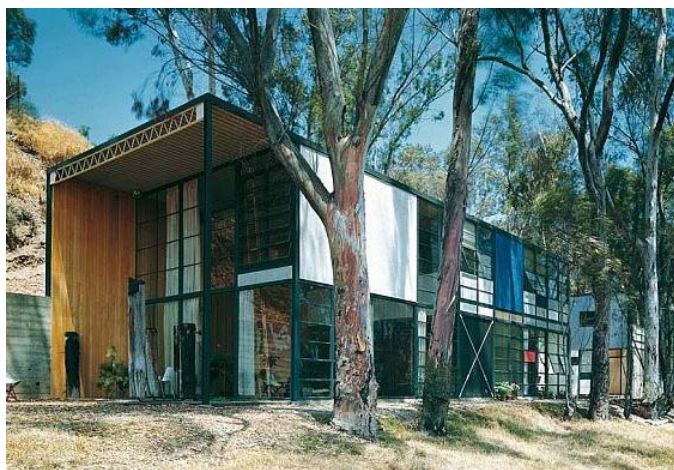
Left: One of the most celebrated of the Case Study Houses, Charles & Ray Eames' House #8 in Pacific Palisades was designed by the couple as a personal residence and studio. Based on a modular system, it is built entirely of prefabricated components including steel, glass, asbestos, and Cemesto board. Craig Ellwood, Pierre Koenig, and Raphael Soriano also designed iconic steel and glass Case Study Houses. Steel and glass houses are less common in San Francisco, although local architect David (Beverly) Thorne's is known for his steel and glass House #26 (1962-1963) in San Rafael, California and the Dave Brubeck House in the Oakland Hills (1954). Photo: www.prefabs2009.org/casestudy/earlyprefabs/files
