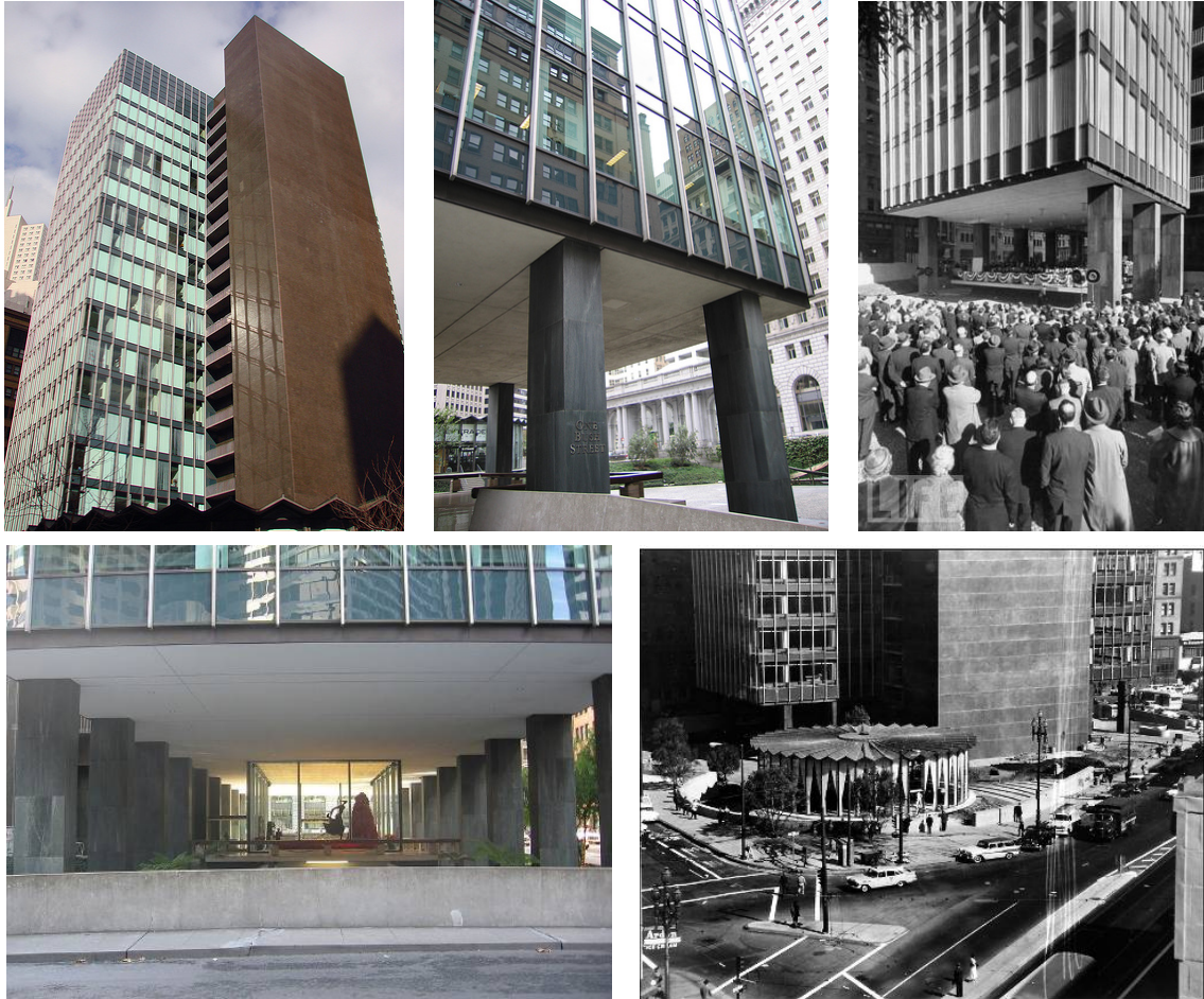
Views of the Crown Zellerbach Building and its ancillary circular bank building. Top right: Opening day celebration. Above left: Perched on pilotis, the building appears to float above the transparent lobby. Photo credits: Life Magazine, Flickr users, and http://blog.wellsfargo.com/GuidedByHistory
