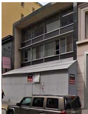
Left: The California Savings Bank, at 46 Geary Street, in 1956 and 2010. Designed in 1956 by architect Ward Thomas, the bank featured a visual open front, open-plan interior, opaque spandrel panels; a projecting box overhang; blade sign; and ‘floated lighting ceilings’ comprised of 50’ plastic fixtures fitted with fluorescent tubes. It reflects the influence of Skidmore Owings and Merrill’s iconic (1954) Modern bank in Midtown Manhattan. Photos: San Francisco History Center, San Francisco Public Library; www.mapjack.com
