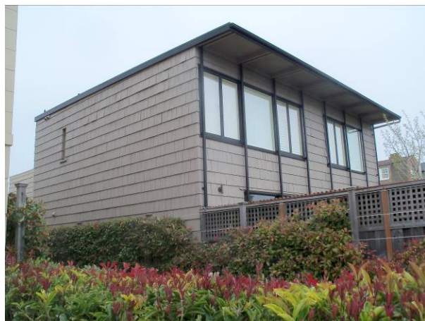
3074 Pacific Avenue, designed by Joseph Esherick (1953). The block features several buildings designed by Esherick and William Wurster. Photo: Mary Brown, San Francisco Planning Department
