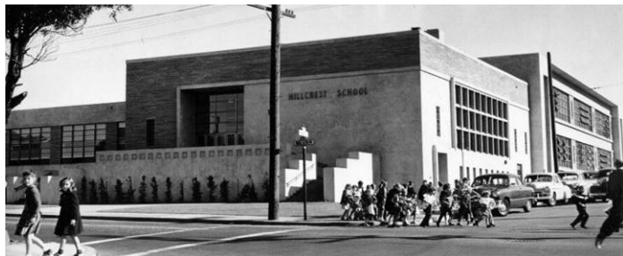
LEFT: Hillcrest Elementary School (1951) on Silver Avenue.
