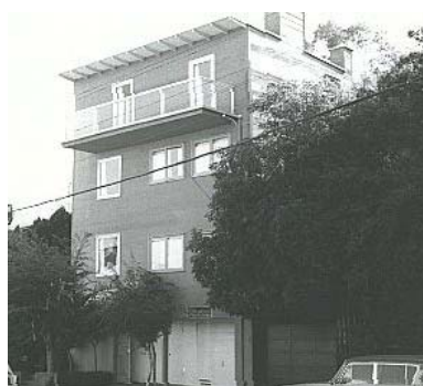
Left: The Harley-Stevens House (1940, William Wurster) at 1641 Green Street.
