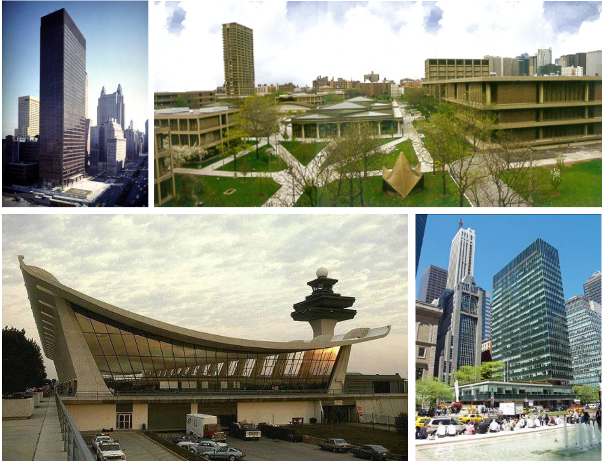
Top left: Mies van der Rohe's Seagram Building (left), a 38-story office skyscraper constructed in New York City (1954-58), Mies utilized a steel frame clad with a taut curtain wall of amber-tinted glass and bronze mullions to create an external expression of the building's structure. The Seagram building is fronted by a large, open urban plaza, one that inspired downtown NYC (and later, San Francisco) to enact Downtown open-space requirements. Photo: www.greatbuildings.com
