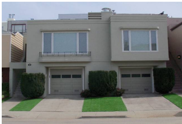
LEFT: Constructed in 1948, this late Streamline Moderne single-family residence is located in the Anza Vista neighborhood, a builder-developed residential tract. The somewhat restrained design includes key character-defining features such as rounded corners, speed lines, balconette, original window configuration, rounded projecting overhangs, and an asymmetrical façade. Aside from the replacement garage doors, the building retains integrity of design, materials and feeling and may qualify for local and state listing as a district contributor under Criteria C/3. Photo: Mary Brown, San Francisco Planning Department
