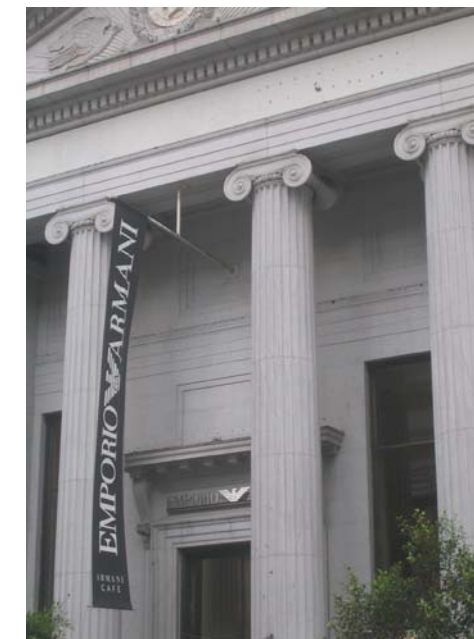
Existing banner at Grant Ave to be replaced. Source: Page & Turnbull
