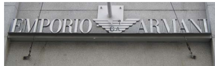
Existing signage at O'Farrell Street entrance to be replaced, with similar signage except text and metal to be gloss black colored. Source: Page & Turnbull
