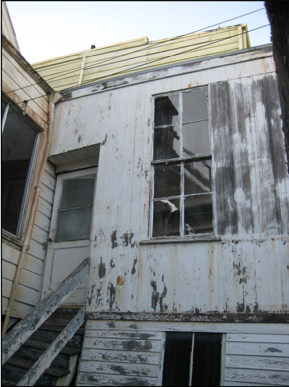
Subject Property, Detail of Rear Facade
