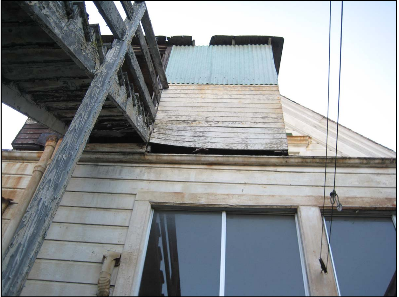
Subject Property, Detail of Rear Facade
