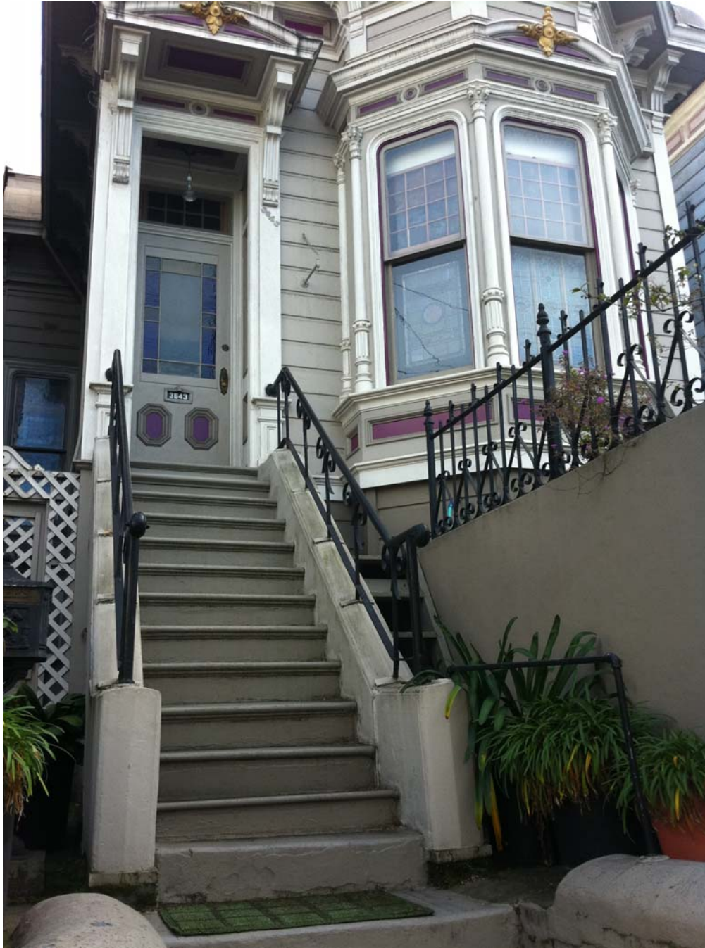
Historic Handrail Example, 3643 20th Street
