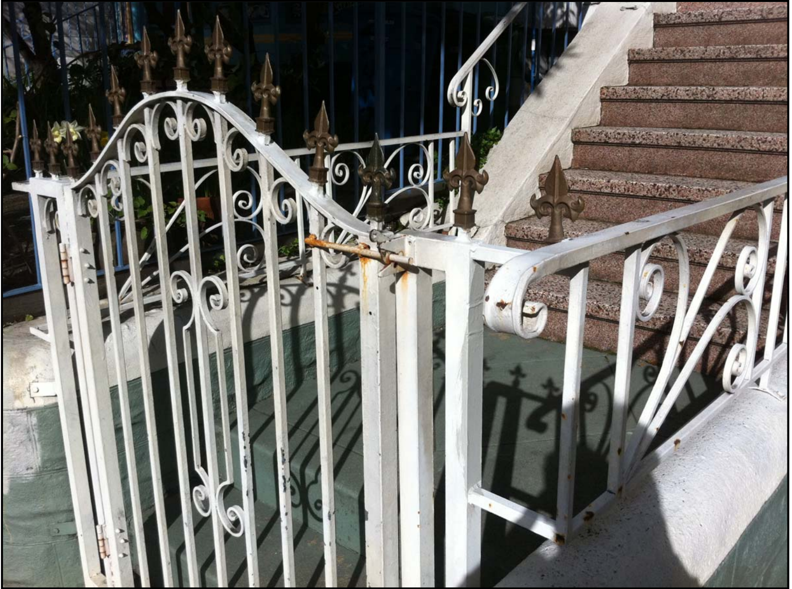
Non-Historic, Compatible, Handrail Example, 959-61 Valencia Street
