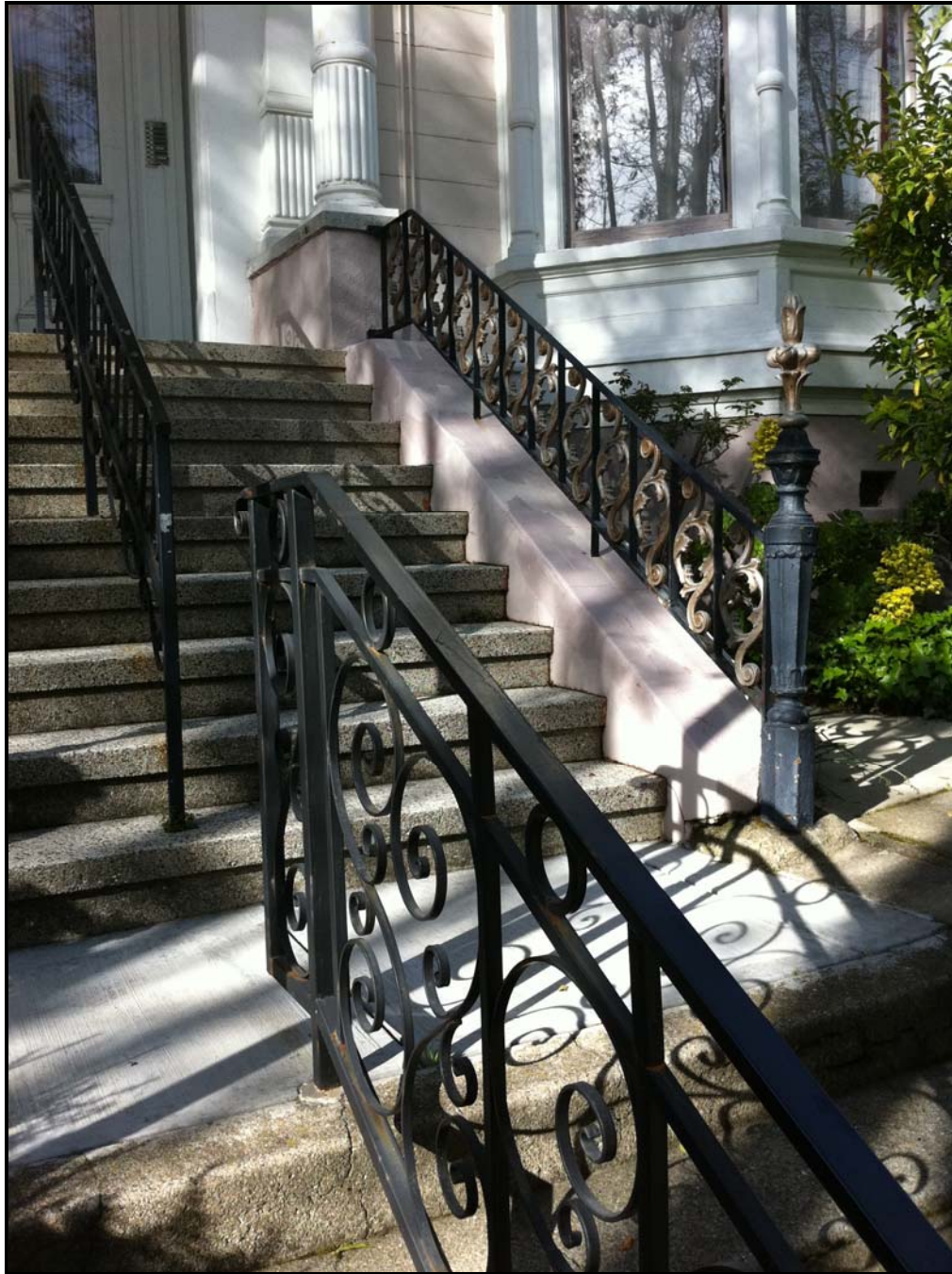
Compatible Alteration, Handrail Example, 58 Liberty Street
