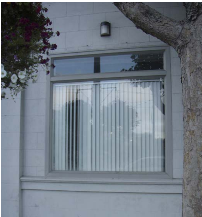
17. Existing windows & lighting
