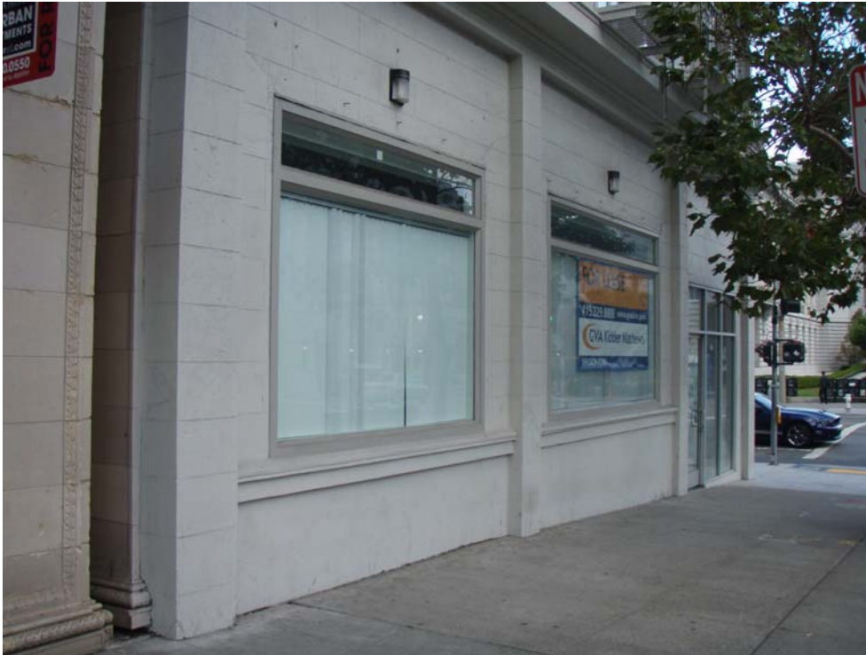
16. Detail of windows along Van Ness
