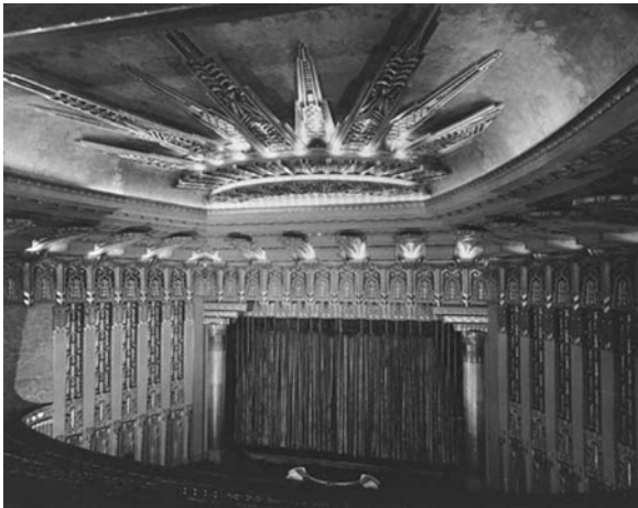
Figure 46. Wiltern Theater (1931), Los Angeles. Source: Los Angeles Public Library, in Cinema Treasures, www.cinematreasures.org (accessed 15 October 2007).
