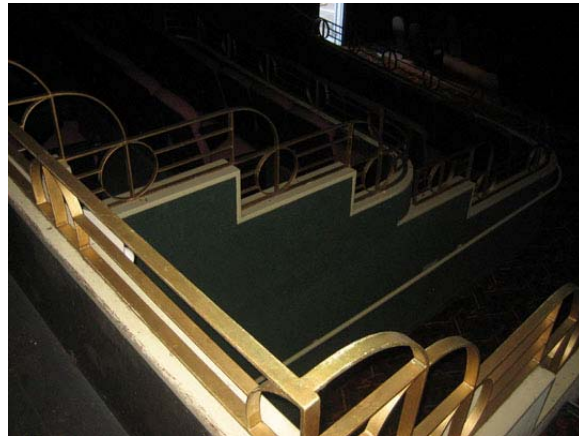
Figure 13. Art Deco balustrades on loggia. Note: Illustrated are a combination of original 1941 balustrades and matching 1998 replacements. Source: Page & Turnbull, Oct 2007.
