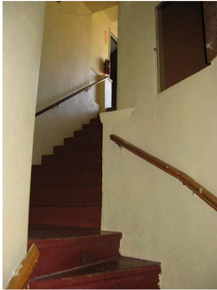
Figure 18. Staircase. View northwest from first floor lobby. Source: Page & Turnbull, Oct 2007.
