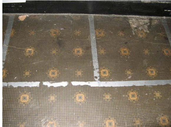
Figure 21. Mosaic flooring, second floor hallway. Source: Page & Turnbull, Oct 2007.
