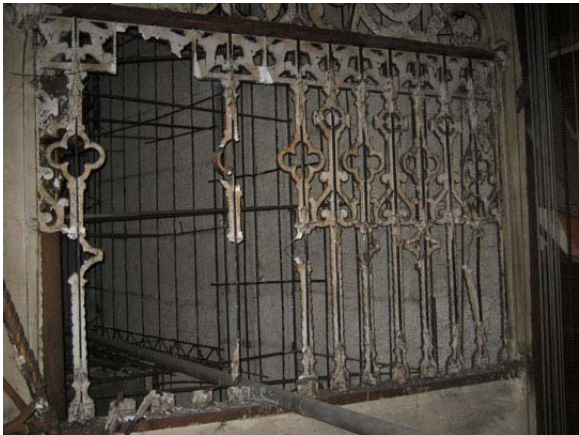
Figure 16. Original (1924) organ grille work behind modern screen. Source: Page & Turnbull, Oct 2007.
