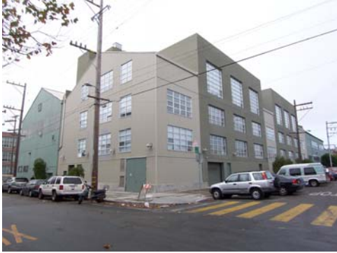
100_5515.JPG, 11/19/2007, view to NW, new portion
