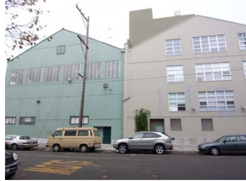
100_5516.JPG, 11/19/2007, view to N
