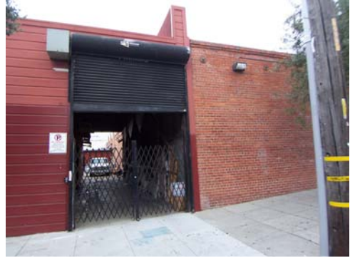
100_5205.JPG, 11/16/07, view to N, eastern building
