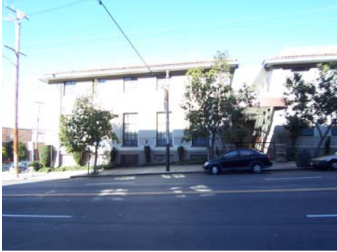
100_6186.JPG, 11/23/07, view to N
