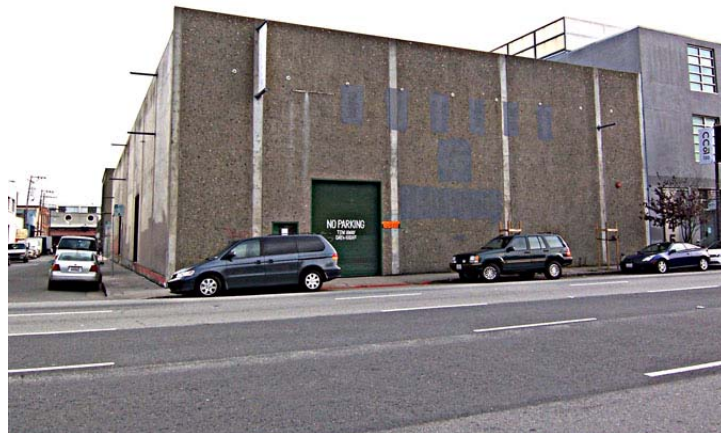
Figure 51. 925 Bryant St. Source: KVP Consulting
