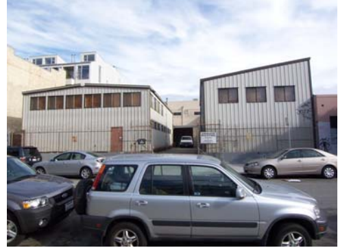
100_5529.JPG, 11/19/07, view to E, Alabama St. elevation
