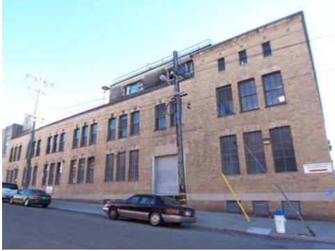
100_6268.JPG, 11/23/2007, view to S, Alameda St elevation
