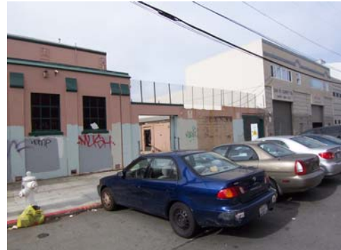
100_5243.JPG, 11/16/07, view to W, building 4 behind wall
