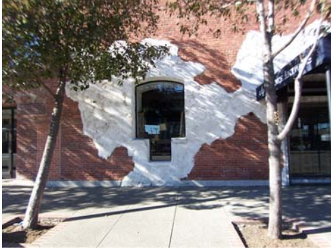
100_6064.JPG, 11/23/07, detail east elevation
