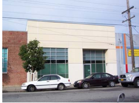
100_1920.JPG, 11/16/07, view to N, eastern building
