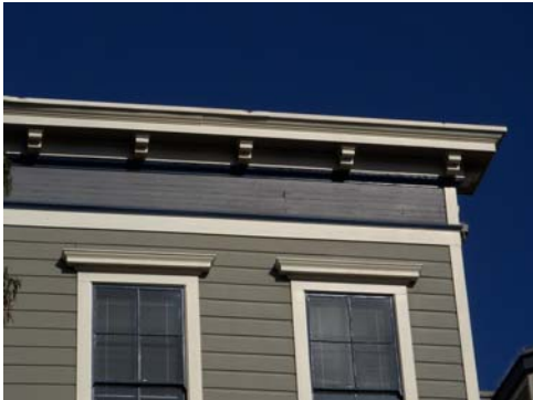
100_5764.JPG, 11/21/07, view to N, cornice detail
