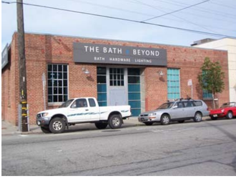
100_1919.JPG, 11/16/07, view to N, western building
