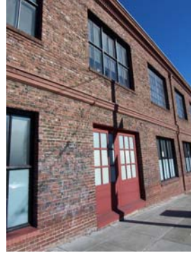
100_6030.JPG, 11/23/07, detail south elevation
