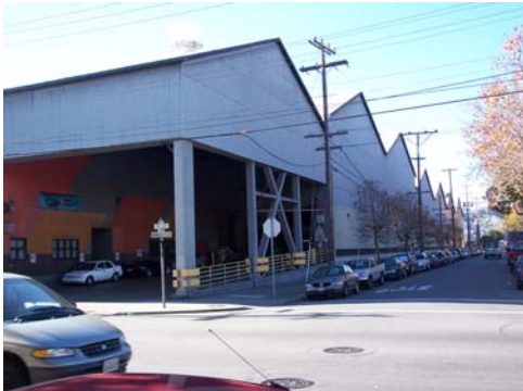
100_5867.JPG, 11/21/07, view to W, north elevation
