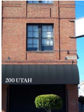
100_6048.JPG, 11/23/07, detail NE corner
