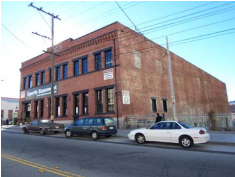
100_62531.JPG, 11/23/07, Florida St. elevation
