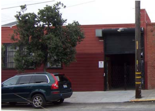
100_5206-1, 11/16/07, view to N, eastern building
