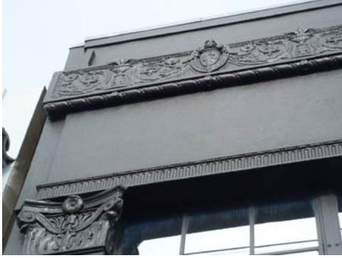
100_6536.JPG, 12/4/07, view to N, cornice & capital detail
