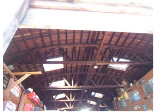
100_6421.JPG, 11/28/07, view to N, interior eastern building
