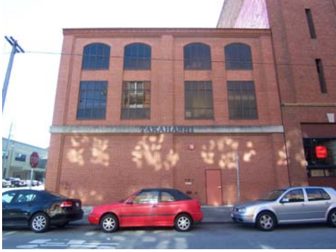
100_2229.JPG, 11/21/07, north elevation
