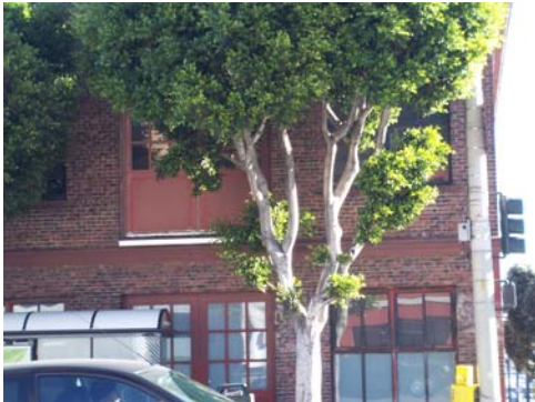
100_6029.JPG, 11/23/07, detail west elevation
