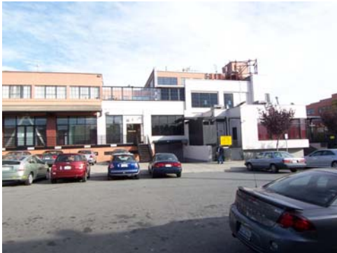
100_5609.JPG, 11/19/07, view to E, annex
