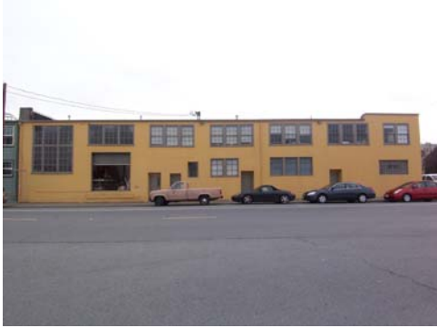
100_1950.JPG. 11/16/07, view to S
