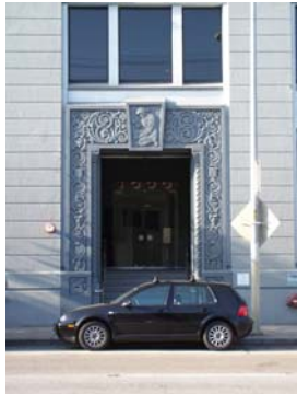
100_2622.JPG, detail main entrance, 11/27/2007
