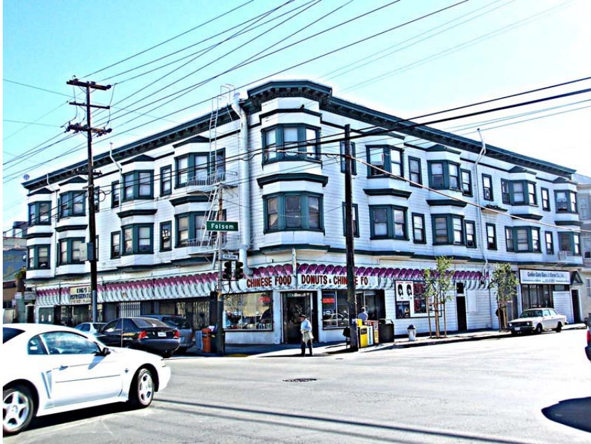
Figure 65. Wagner Hotel, 2011 Folsom Street Source: KVP Consulting
