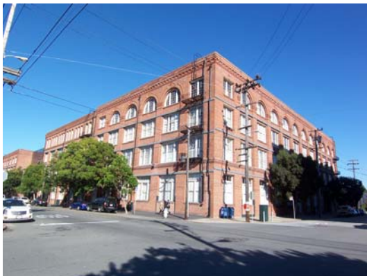
Figure 6. Kansas Street warehouses Source: KVP Consulting
