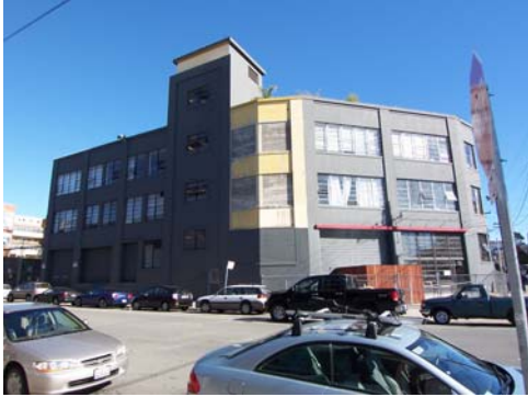
100_5714.JPG, 11/20/07, view to NE
