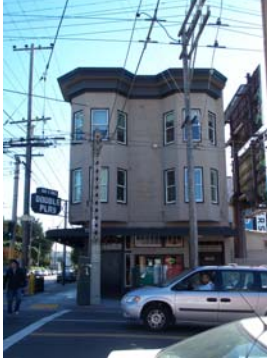
100_5952.JPG, 11/21/2007, view to S
