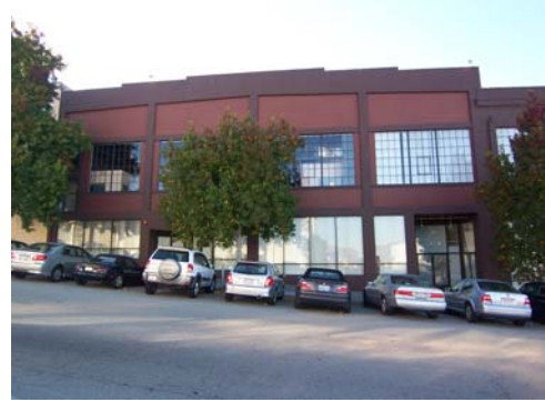
100_2145.JPG, 11/20/07, view to W, concrete addition
