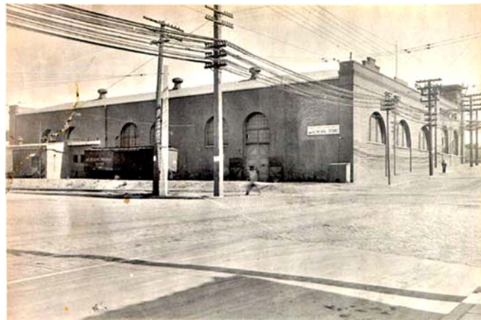
Figure 9. Market Street Railway Powerhouse, n.d. Source: San Francisco Public Library
