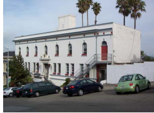
View toward northeast, 11.16.07, 100_1901.JPG
