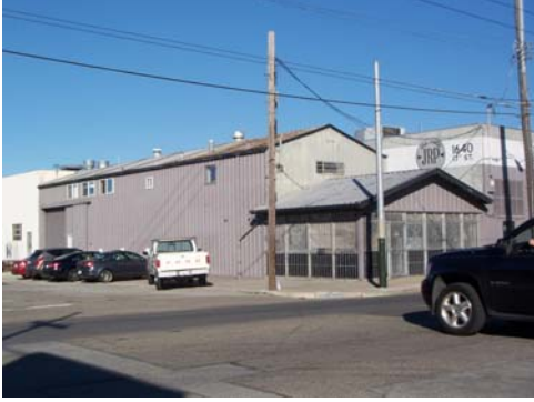
100_2107.JPG, 11/20/07, view to NE
