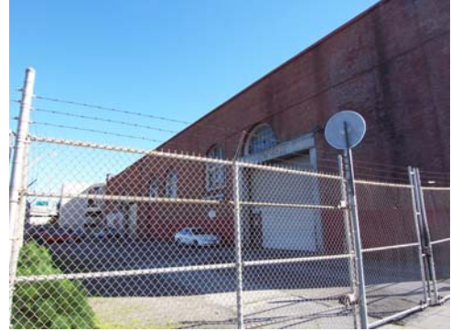
North facade, 11.23.07, 100_6217.JPG
