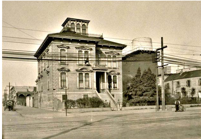
Figure 18. John Center House and Water Works, 1925 Source: Bancroft Library
