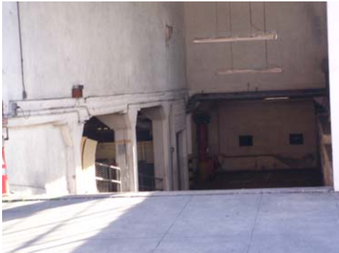
100_6240.JPG, 11/23/2007, detail, 15th St. vehicular entrance
