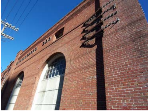
Detail window & brickwork, 11.23.07, 100_6216.JPG,
