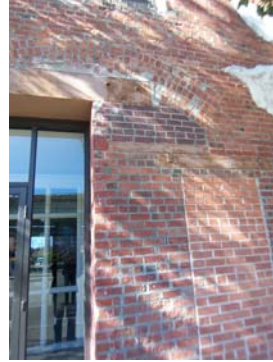
100_6068.JPG, 11/23/07, detail brickwork & window
