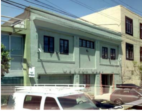
100_5487_2.JPG, 11/19/2007, east elevation
