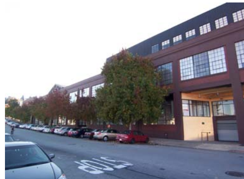
100_2142.JPG, 11/20/07, south elevation
