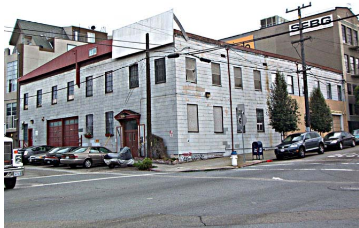
Figure 13. Berger & Carter warehouse Source: KVP Consulting, LLC
