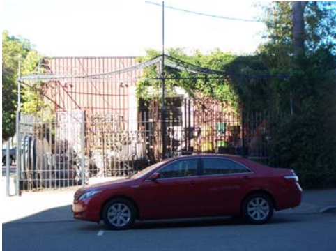
100_2342.JPG, 11/26/07, view to N, corrugated metal section
