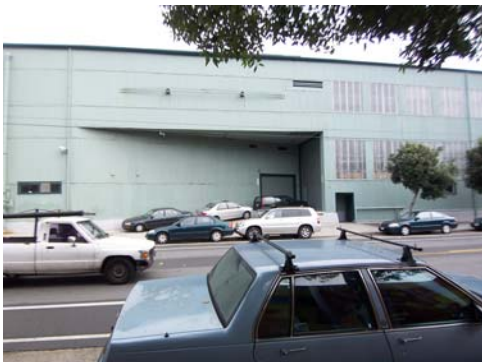
100_5520.JPG, 11/19/2007, west elevation rail car entrance
