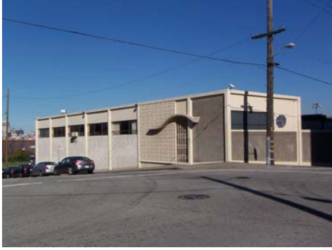
View to NE, 11/20/07, 100_2070.JPG
