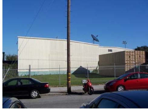
100_2074.JPG, 11/20/07, view to E, steel building
