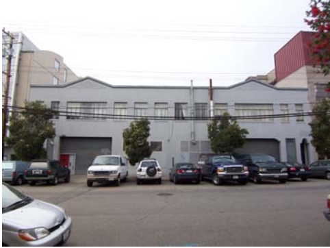
100_5155.JPG, 11/16/2007, view to W, east elevation
