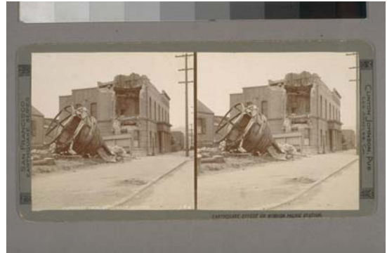
1906, showing earthquake damage
