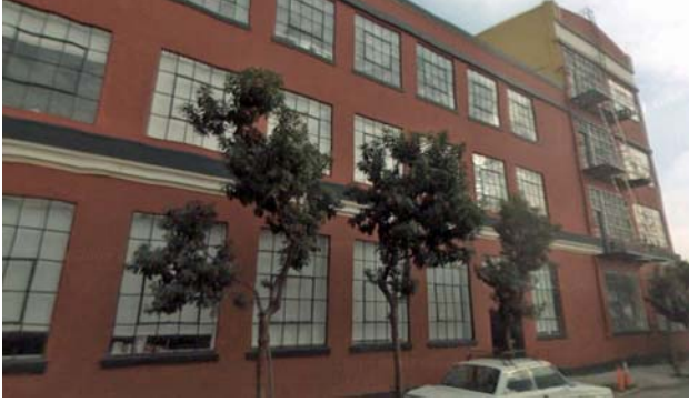
100_5339.T.JPG, 11/16/2007, view to E, Treat St elevation
