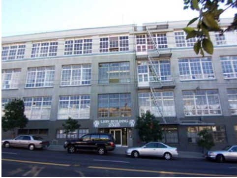
100_5934.JPG, 11/21/2007, view to S
