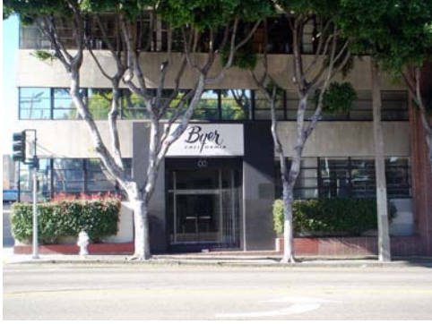
100_6110.JPG, 11/23/07, east elevation
