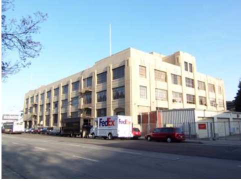
View toward east, 11.27.07, 100_2665.JPG
