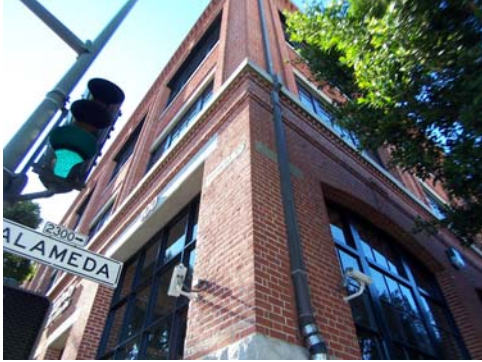
100_6122.JPG, 11/23/07, detail NE corner
