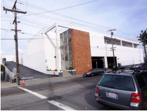
100_5274.JPG, 11/16/07, view to NE
