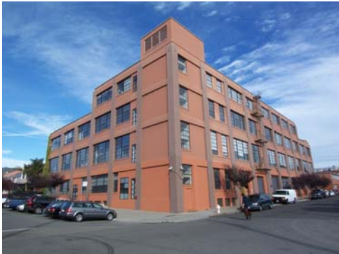
100_5596.JPG, 11/19/07, view to NE
