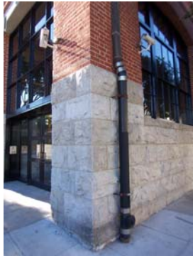
100_6123.JPG, 11/23/07, detail NE corner, base
