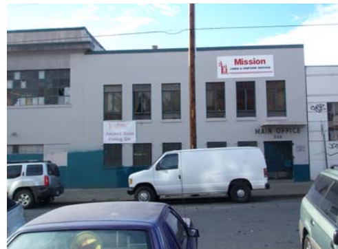
100_5623.JPG, 11/19/2007, office entrance
