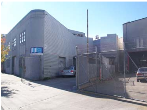
100_5857.JPG, 11/21/07, detail NE corner
