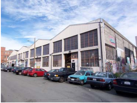
100_5563.JPG, 11/19/2007, Florida St. elevation
