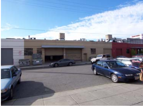
100_5618.JPG, 11/19/07, view to E, Florida elevation
