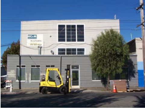
South elevation, entrance, 11/20/07, 100_2084.JPG
