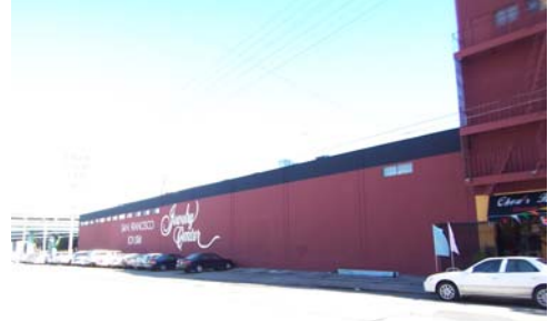
100_6080.JPG, 11/23/07, view to NE
