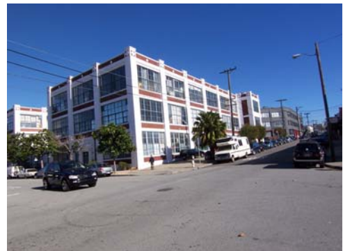
100_5730.JPG, 11/20/2007, view to NE
