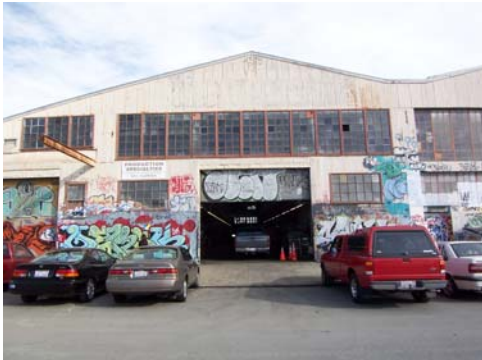
100_5568.JPG, 11/19/2007, addition (left)
