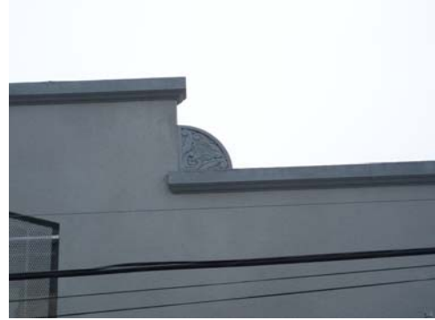
100_5171.JPG, 11/16/2007, parapet detail
