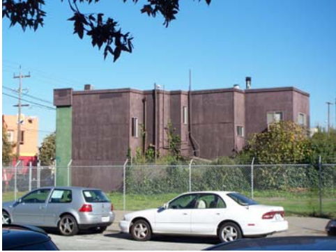
100_2073.JPG, 11/20/07, view to E, frame building
