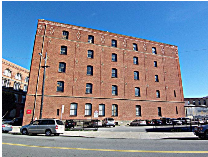
Figure 23. J.I. Case Threshing Co. Building, 200 Rhode Island St. Source: KVP Consulting
