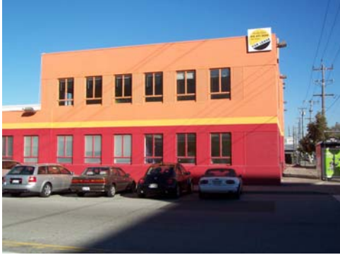
100_2116.JPG, 11/20/07, view to E
