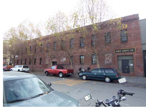
100_5551.JPG, 11/19/07, view to S
