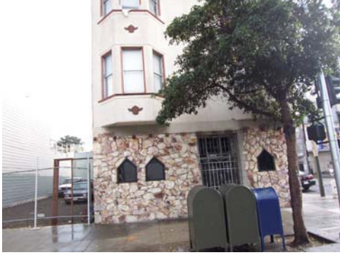
100_6522.JPG, 12/4/07, view to E
