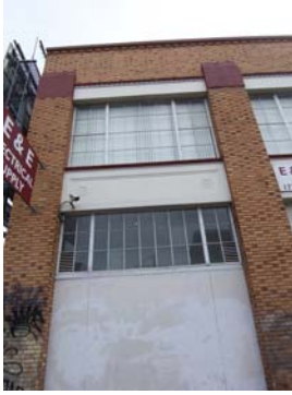
100_6518.JPG, 12/4/07, view to E, detail
