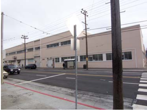
100_5359.JPG, view to NE
