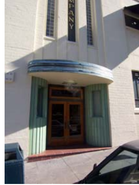
100_2039.JPG, 11/20/07, entrance detail
