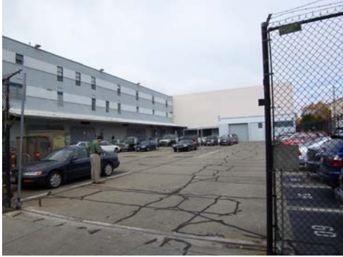
100_5247.JPG, 11/16/07, view to NW, ancillary building at rear
