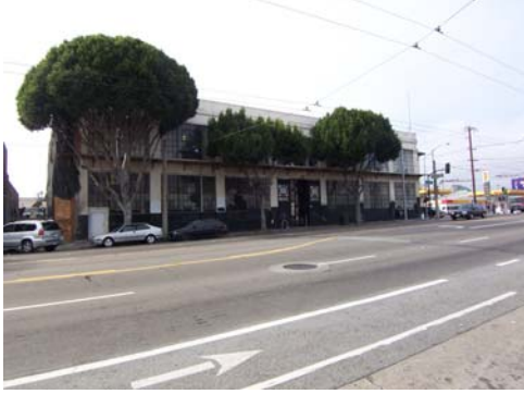
100_5305.JPG, 11/16/07, Potrero Ave. elevation
