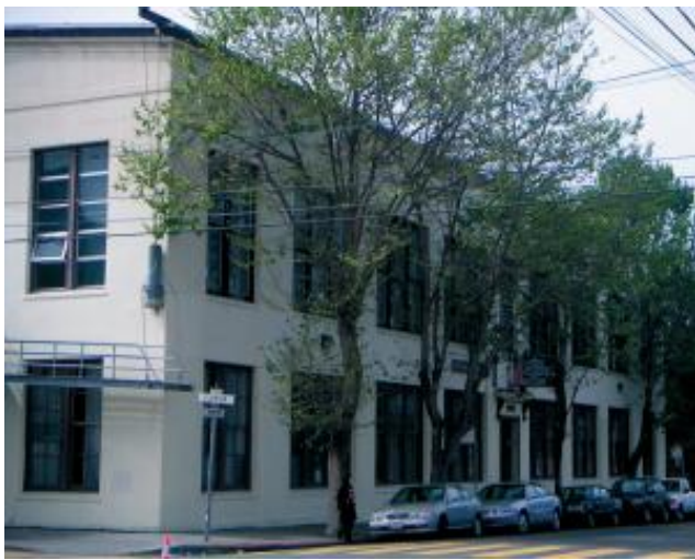
Photo: 2929 19 th St. Pelton Factory. Production type plant.
