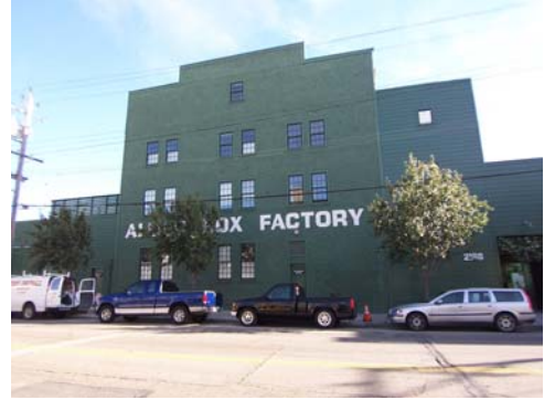
100_5750.JPG, 11/21/07, view to E, central building
