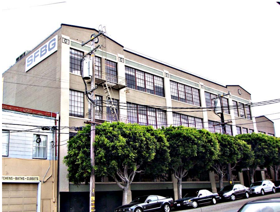
Figure 68. Berger & Carter Warehouse, 135 Mississippi Street Source: KVP Consulting
