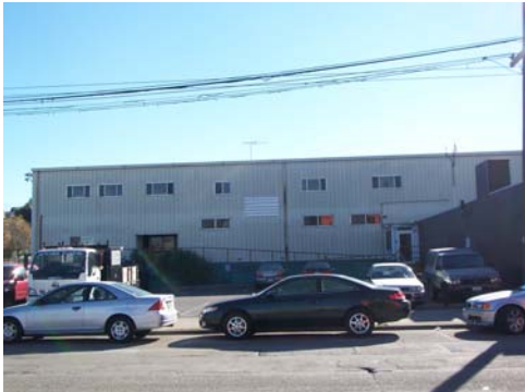
100_2076.JPG, 11/20/07, view to S, steel building
