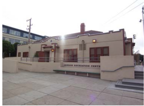
View toward south, 11.16.07, 100_1962.JPG
