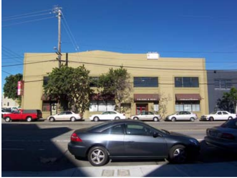
100_2255.JPG, south elevation, 11/21/2007
