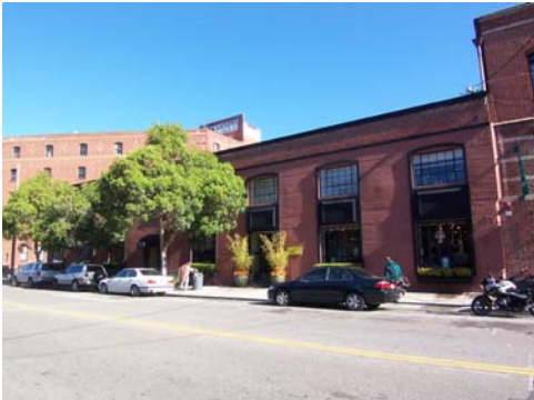
100_2246.JPG, 11/21/07, view to E
