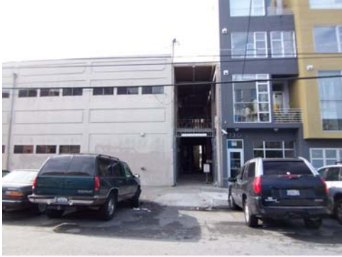
100_5530.JPG, 11/19/07, view to W, pass through
