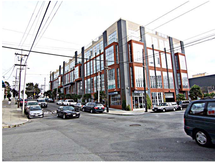
Figure 54. 1800 Bryant St. Source: KVP Consulting
