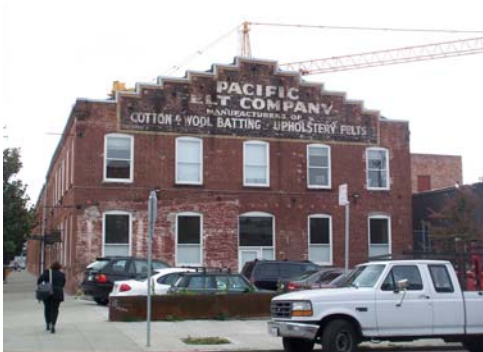
North elevation, 11/16/07, 100_5213.JPG
