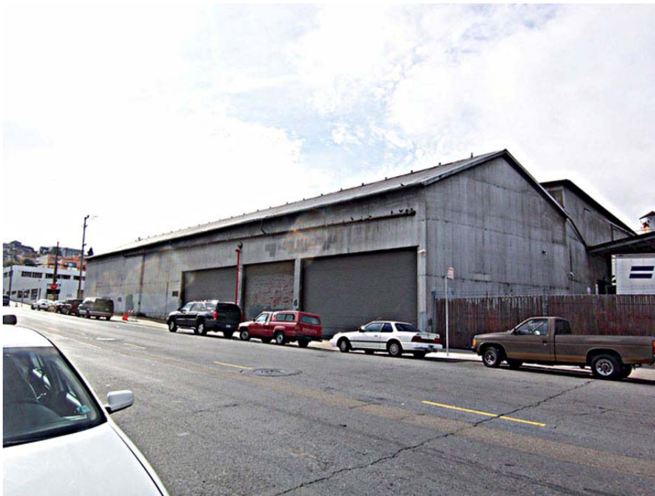
Figure 71. Pacific Rolling Mills warehouse, 1200 17 th St. Source: KVP Consulting
