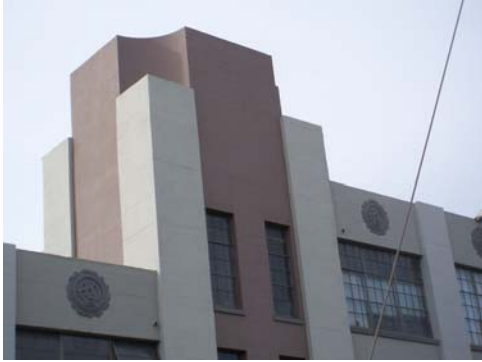
100_5325.JPG, 11/16/2007, tower detail
