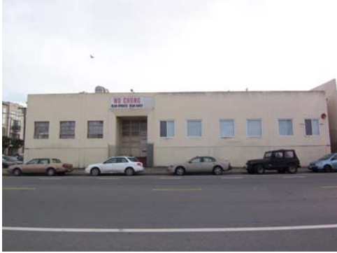
16th Street elevation, 11/16/07, 100_1928.JPG
