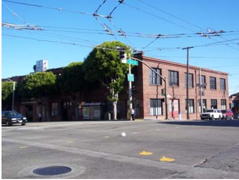
100_6026.JPG, 11/23/07, view to NE
