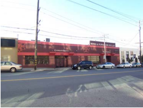
View to west, both buildings, 11/20/07, 100_2169.JPG
