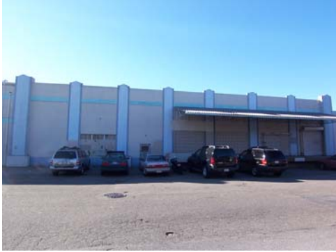
100_2346.JPG, 11/26/07, view to W, 2 story section
