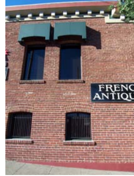
100_6018.JPG, 11/23/07, detail east elevation
