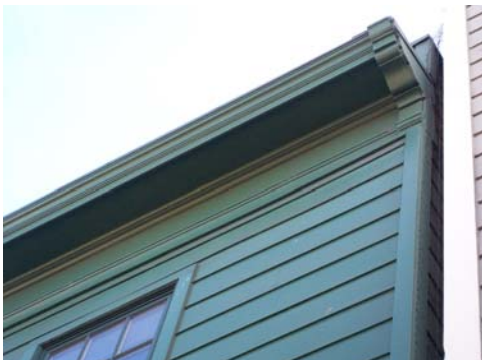
100_5758.JPG, 11/21/07, cornice detail
