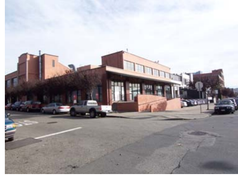
100_5607.JPG, 11/19/07, view to SE, western building
