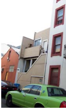
100_2585A.JPG, view to SW, 11/26/07, Kate St. elevation
