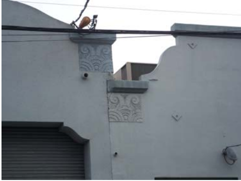
100_5170.JPG, 11/16/2007, parapet detail
