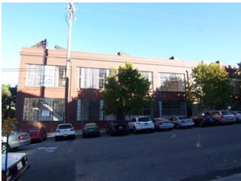
100_2154.JPG, 11/20/07, view to E
