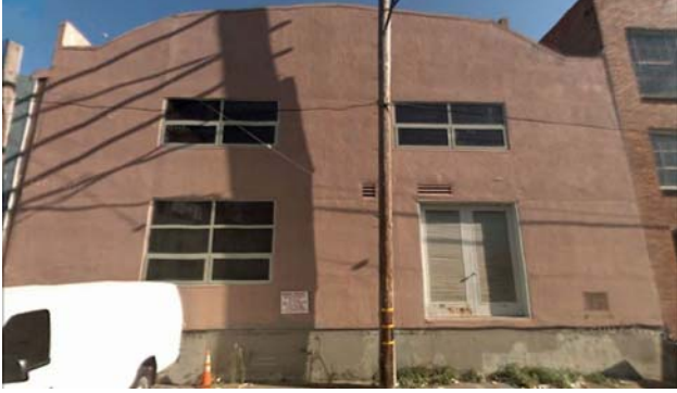
100_2534.2.JPG, view to E, 11/26/07, Langton St. elevation
