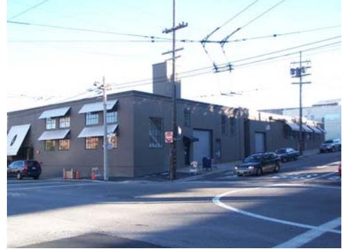
View to SE, Vermont elevation, 11/21/07, 100_2162.JPG
