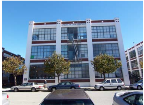
100_5726.JPG, 11/20/2007, view to E
