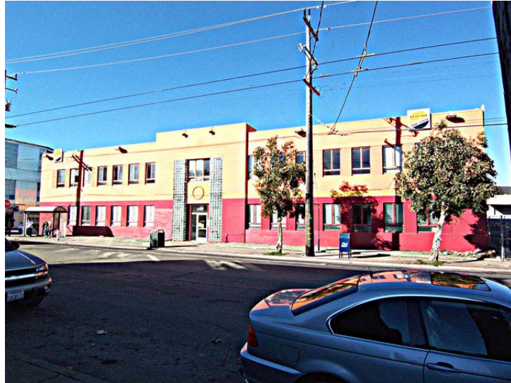
Figure 43. John A. Roebling & Sons Wire Rope Co., 1740 17 th St. Source: KVP Consulting
