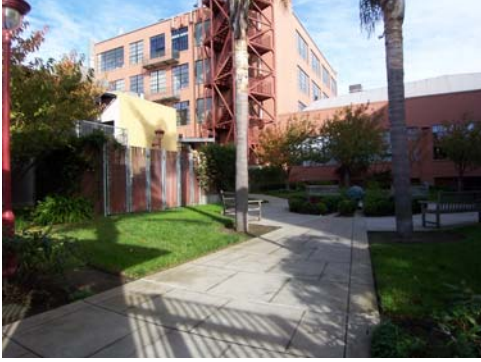
100_5614, 11/19/07, view to NE, south & west elevations
