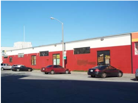
100_2118.JPG, 11/20/07, view to NE
