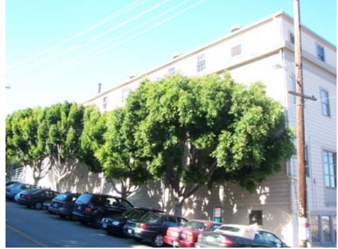
100_2048.JPG, 10/20/07, 18th St. south elevation
