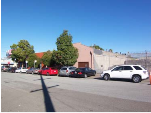
West elevation, 11/21/07, 100_2090.JPG
