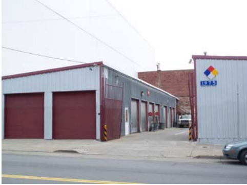
100_5177.JPG, 11/16/07, view to NE
