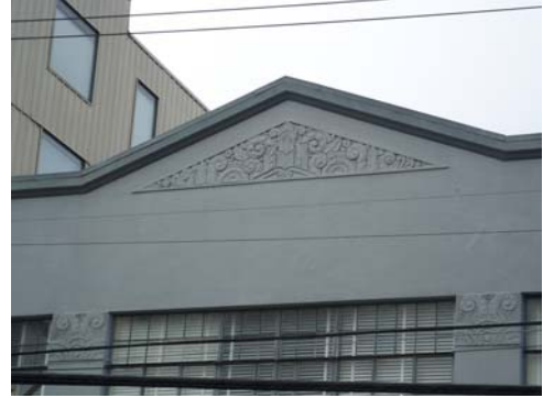
100_5156.JPG, 11/16/2007, parapet detail
