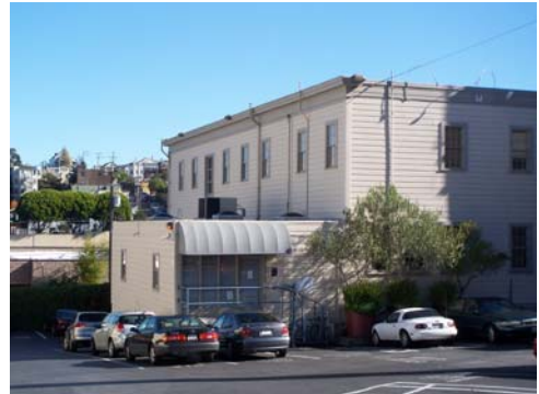
100_2056.JPG, 10/20/07, north elevation
