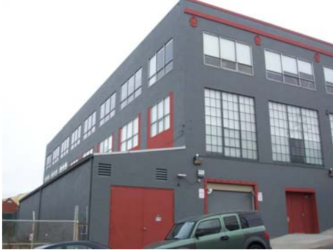
100_5139.JPG, 11/16/2007, view to NE
