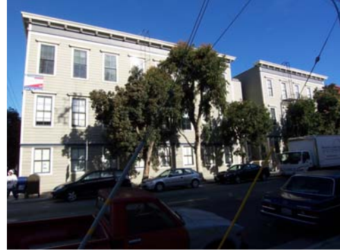
100_5762.JPG, 11/21/07, view to N, two buildings & connector
