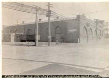
Sub Station & Storehouse - Bryant & Alameda. M.S.R.R. 1901
