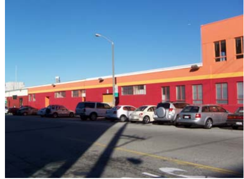
100_2117.JPG, 11/20/07, view to NE
