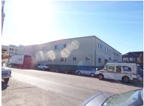
100_2077.JPG, 11/20/07, view to SW, steel building
