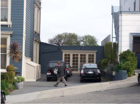
Addition at rear, 11.16.07, 100_1898.JPG
