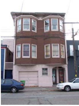
View toward south, 11.16.07, 100_1934.jpg
