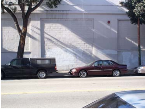
100_6457.JPG, 11/29/07, detail east elevation
