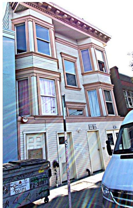
Figure 64. 1771 Folsom Street Source: KVP Consulting
