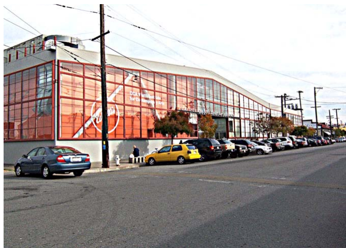
Figure 49. Greyhound garage, 450 Irwin St. Source: KVP Consulting
