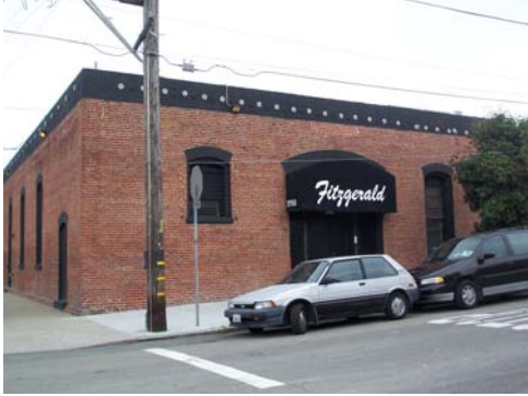
100_5203.JPG, 11/16/07, view to N, main building
