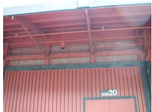
Ssq_005.JPG, 11/12/08, detail, W elevation
