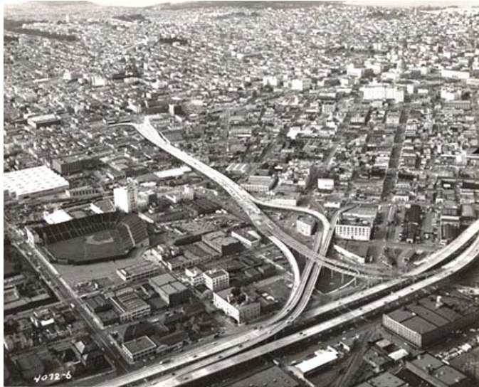
Figure 47. Aerial view of the Bayshore and Central freeways in the survey area, looking northwest Source: San Francisco Public Library
