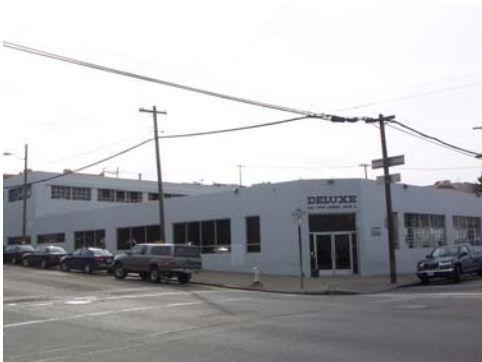
100_1888.JPG, 11/16/07, Texas & 17th street elevations
