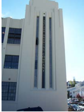
100_2036.JPG, 11/20/07, tower detail
