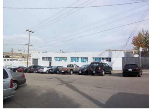
100_1884.JPG, 11/16/07, view to NE
