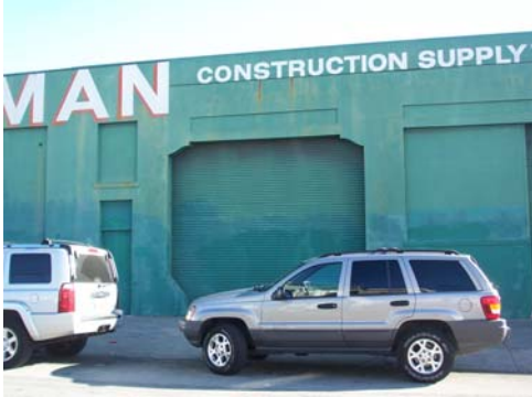
100_6307.JPG, 11/28/07, detail west elevation
