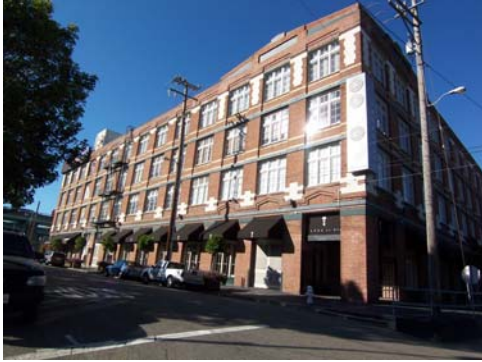
View toward northwest, 11.21.07, 100_2340.JPG
