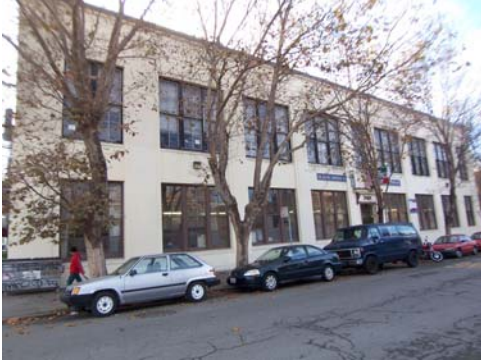
100_5540.JPG, 11/19/2007, view to S
