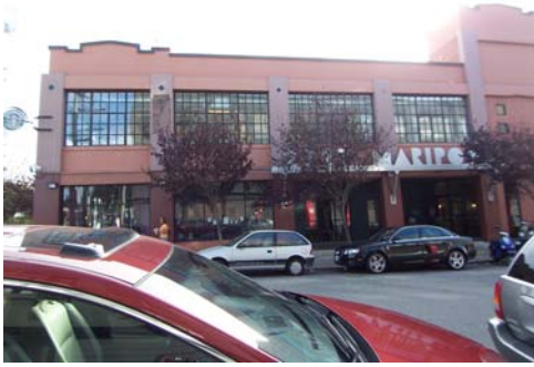
100_5606.JPG, 11/19/07, view to S
