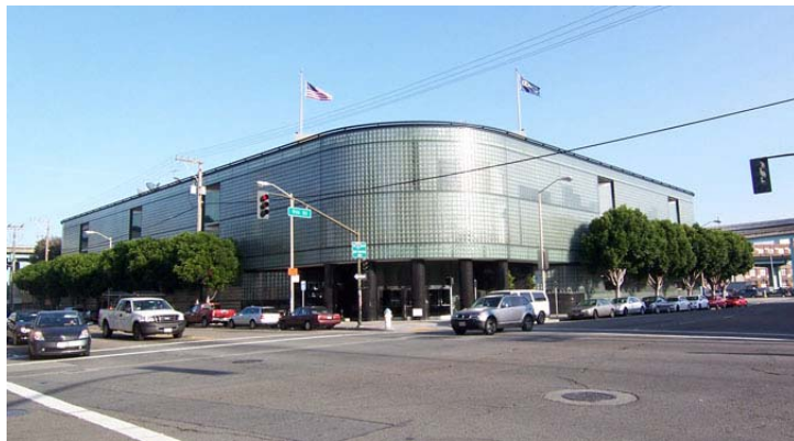
Figure 53. Data Center, 999 Brannan St. Source: KVP Consulting
