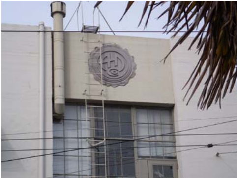
100_5328.JPG, 11/16/2007, parapet detail
