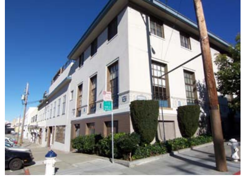
100_6192.JPG, 11/23/07, view to NE
