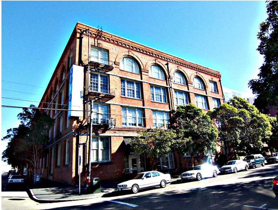
Figure 67. John Hoey & Co. warehouse, 101 Henry Adams Street Source: KVP Consulting
