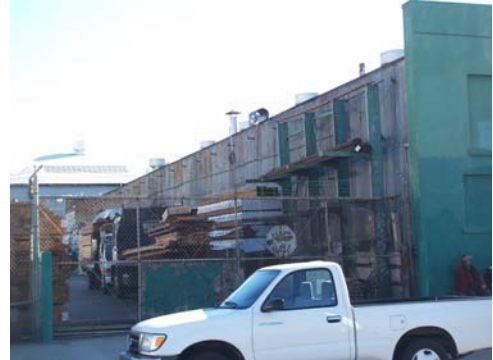
100_6310.JPG, 11/28/07, north elevation
