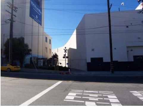
100_6210.JPG, view W, north elevation (left)
