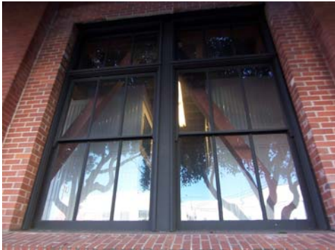
100_5800.JPG, 11/21/07, window detail
