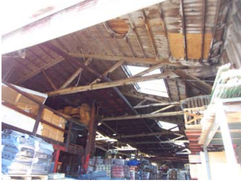
100_6422.JPG, 11/28/07, view to N, interior western building
