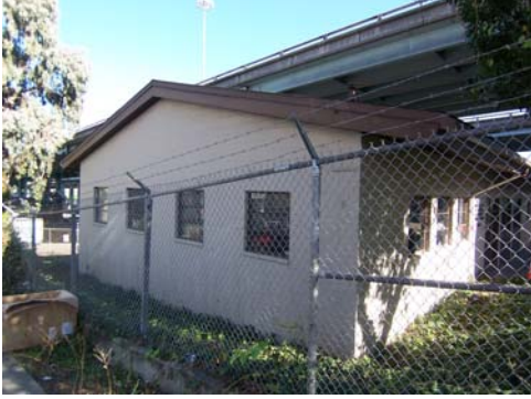
100_2200.JPG, 11/21/07, concrete block utility building
