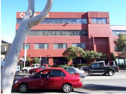
100_6380.JPG, 11/28/07, view to E
