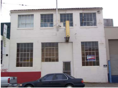
100_1914.JPG, 11/16/07, view to S
