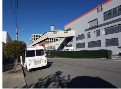
100_6236.JPG, 11/23/2007, view to NE, enclosed bridge on Florida St.
