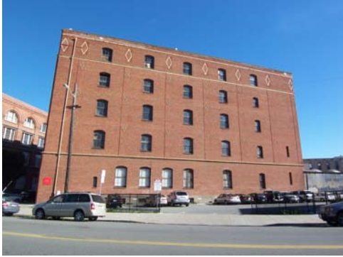
100_2224.JPG, 11/21/07, view to S
