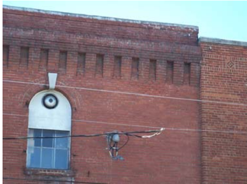
100_5920.JPG, cornice detail
