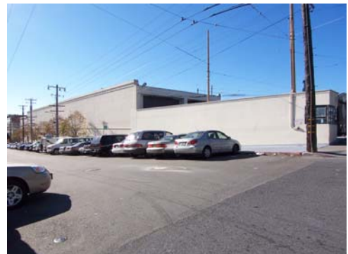
100_5687.JPG, 11/20/2007, view to W, Hampshire St. elevation
