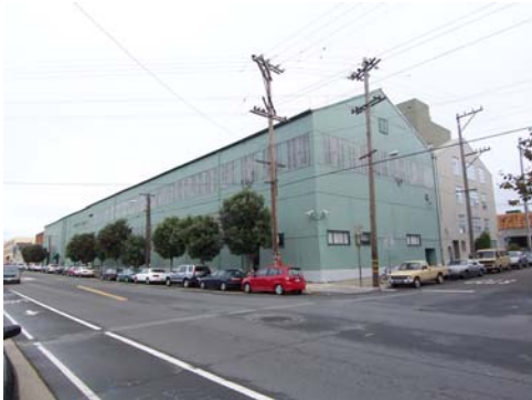
100_5517.JPG, 11/19/2007, view to NE
