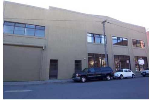
100_2250.JPG, north elevation, 11/21/2007
