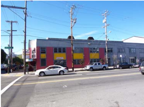
100_5855.JPG, 11/21/07, view to W, east elevation
