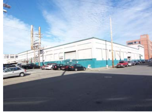
100_5631.JPG, 11/19/2007, view to NE
