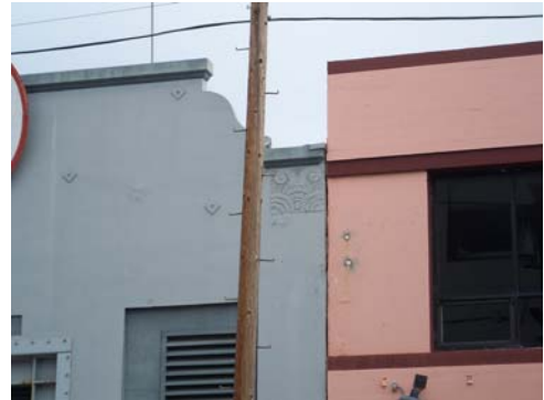
100_5152.JPG, 11/16/2007, parapet detail, west elevation
