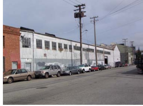
View toward northeast, 11.16.07, 100_1865.JPG
