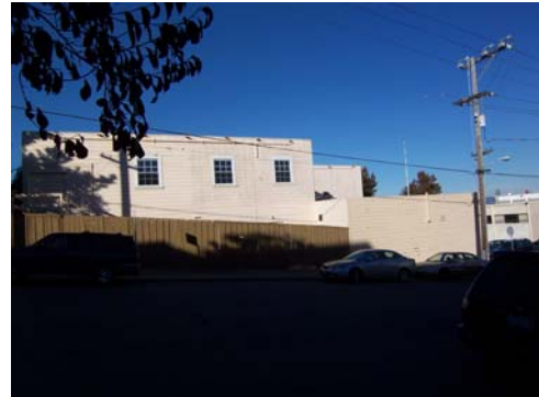
100_2148.JPG, 11/20/07, view to N, frame addition
