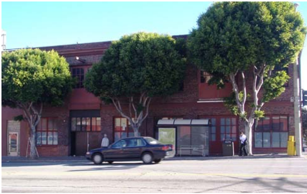
Figure 14. Forderer Cornice Co. building Source: KVP Consulting
