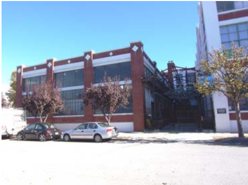
100_5725.JPG, 11/20/2007, view to E
