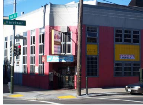
100_5854.JPG, 11/21/07, corner and window detail
