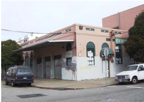
100_5246-1.JPG, 11/16/07, view to NE, building 3
