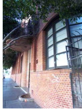
100_5797.JPG, 11/21/07, north elevation, detail
