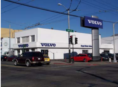
100_6432.JPG, 11/28/07, view to NE
