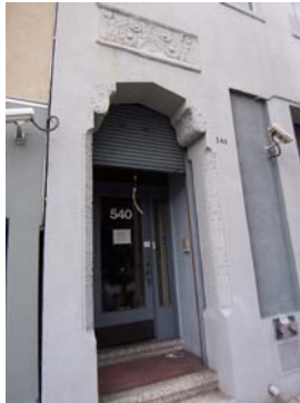
100_5154.JPG, 11/16/07, entrance detail, east elevation
