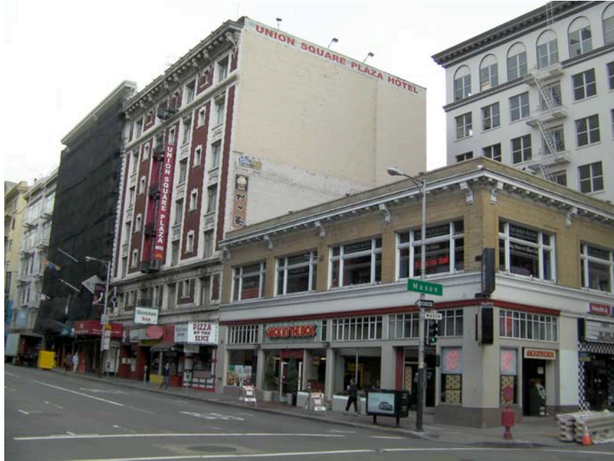
View North West on Geary from Mason and Geary
