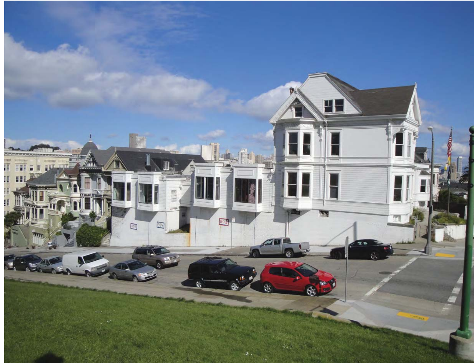
EXISTING CORNER OF STEINER & GROVE
