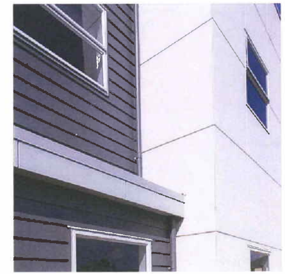
6. EXTERIOR SMOOTH PANEL MATERIAL
