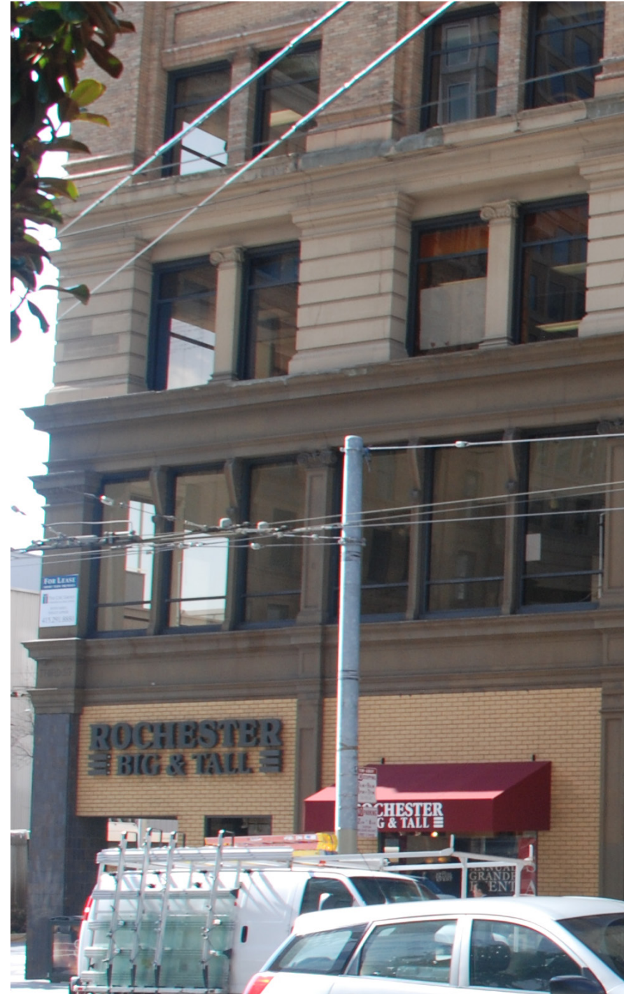
Typical Existing Windows
