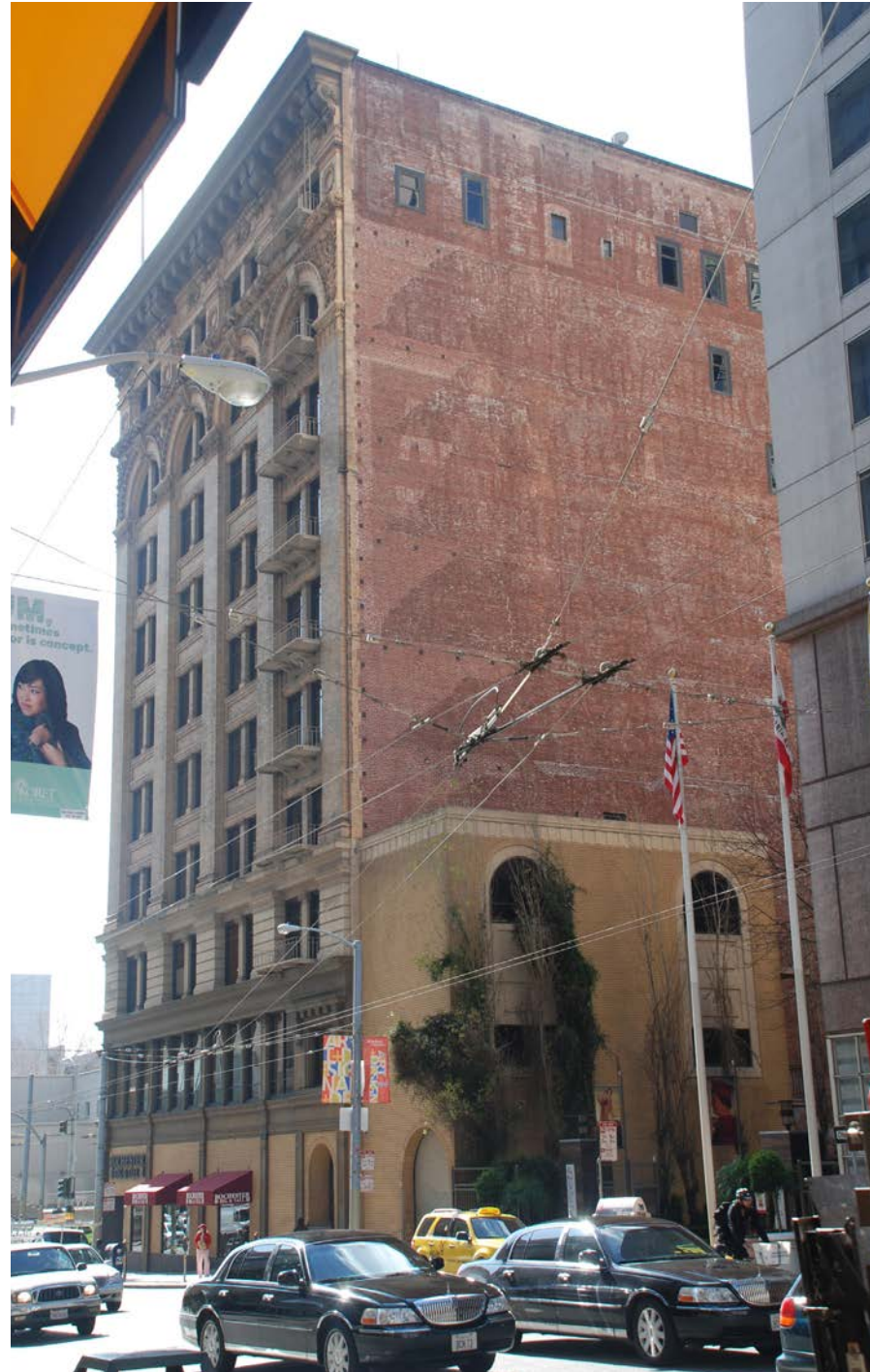
View looking southwest from Third Street
