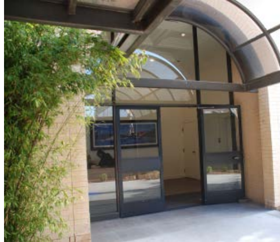
Figure 31. Southwest façade, primary entrance.
