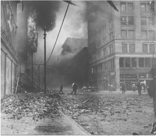
Figure 10. During and after the 1906 Earthquake and Fire. The Aronson Building is located on the right. Source: California Historical Society
