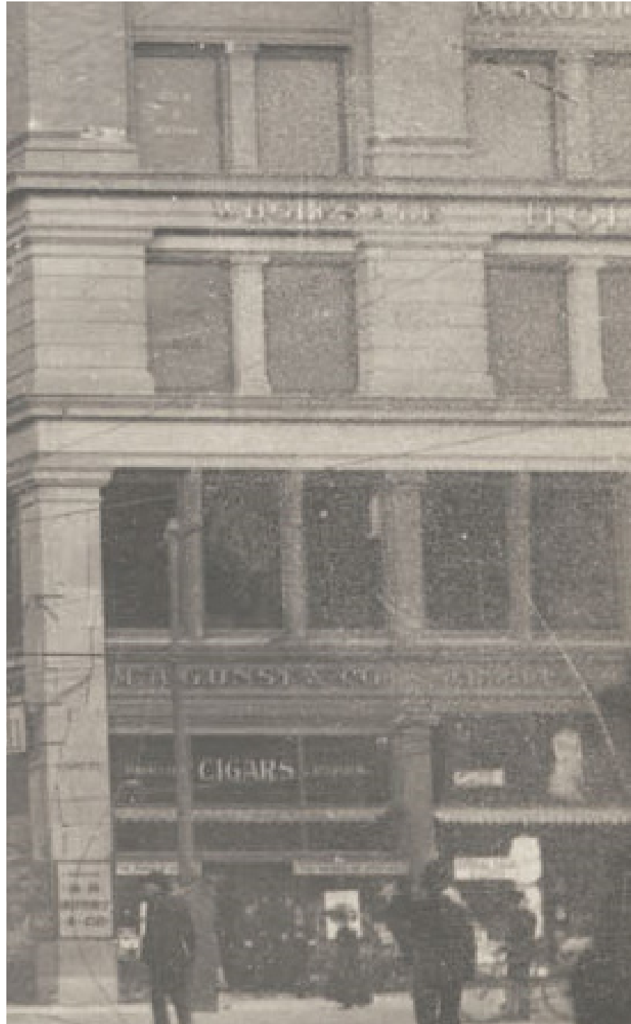
Original windows were simple single lite wood windows
