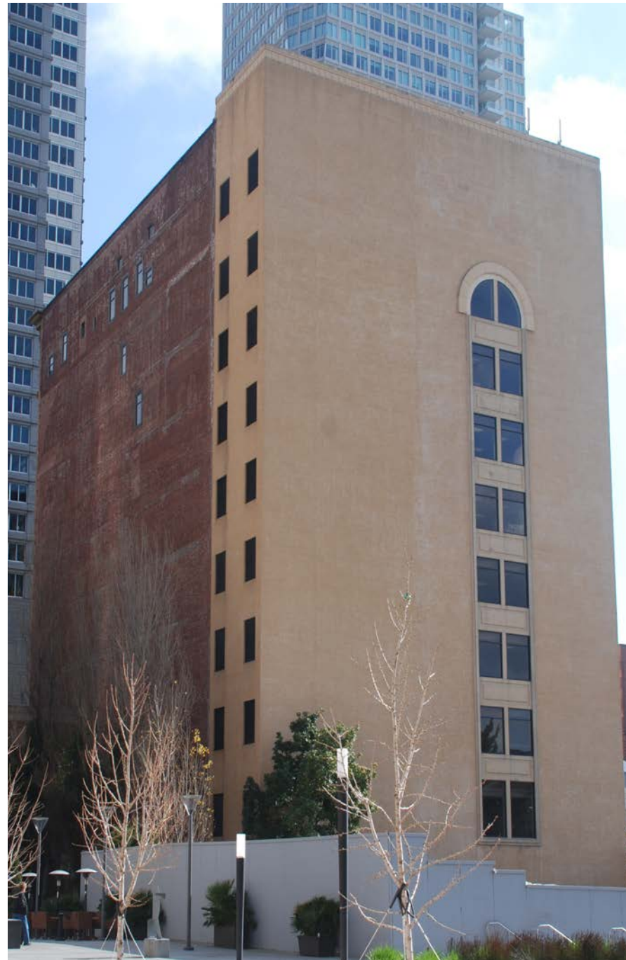
Non-historic addition at west facade, view from northwest
