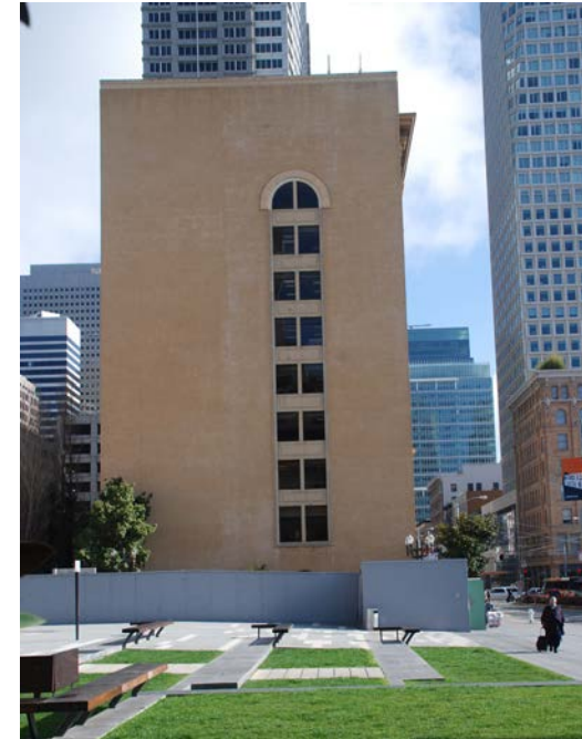
View of Aronson Building from west, Jessie Square in foreground. (Page & Turnbull)
