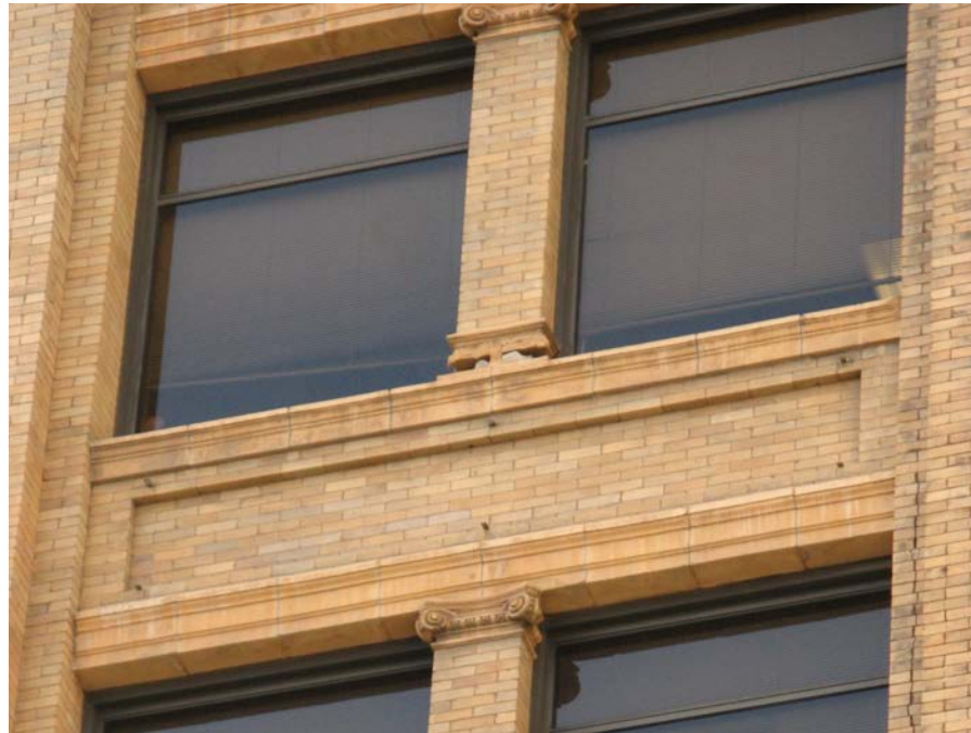
View of brick area to be repaired
