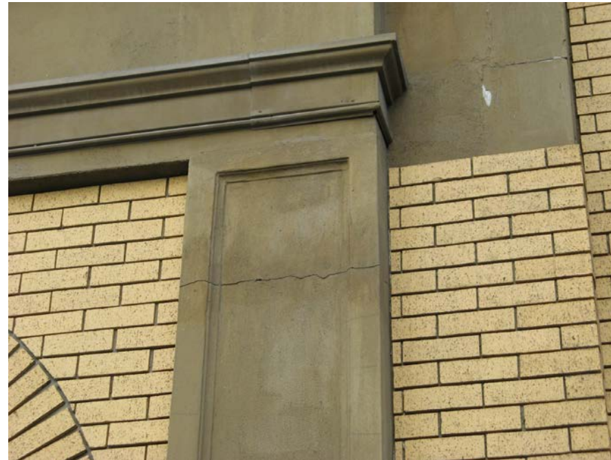
View of pilaster to be repaired
