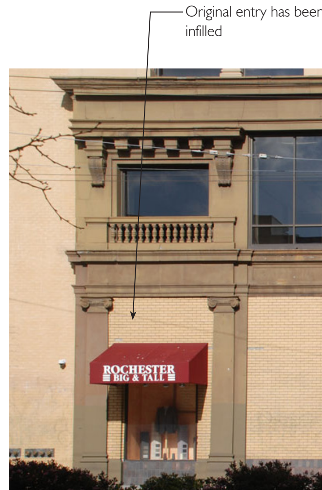
Existing bay where arched entry was located
