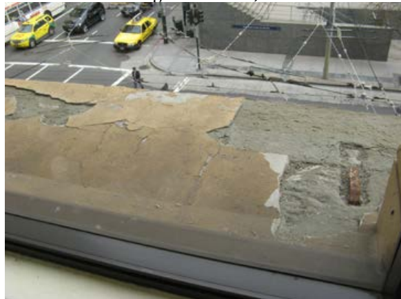
Figure 42. Exfoliation of crust. Source: Page & Turnbull, March 2010.
