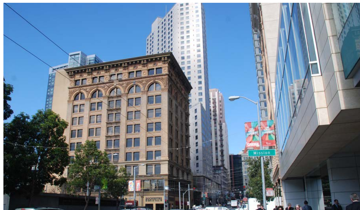
View of Aronson Building from south, Westin Hotel in background. (Page & Turnbull)
