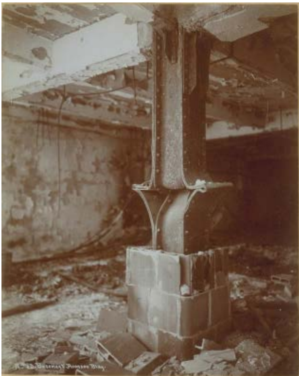
Figure 13. Buckled I-beam encased in failed hollow tiles in the basement, 1906. Source: Bancroft Library.
