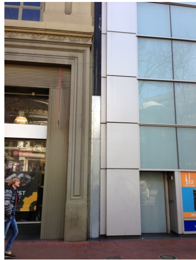
Close-up view of the seismic joint at 735 Market Street
