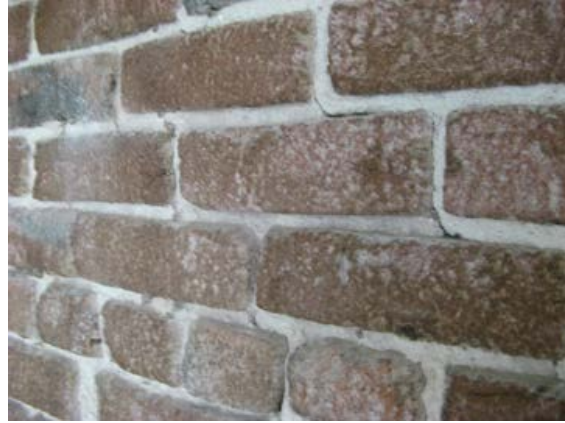
Figure 38. Interior brick face. Source: Page & Turnbull, March 2010.
