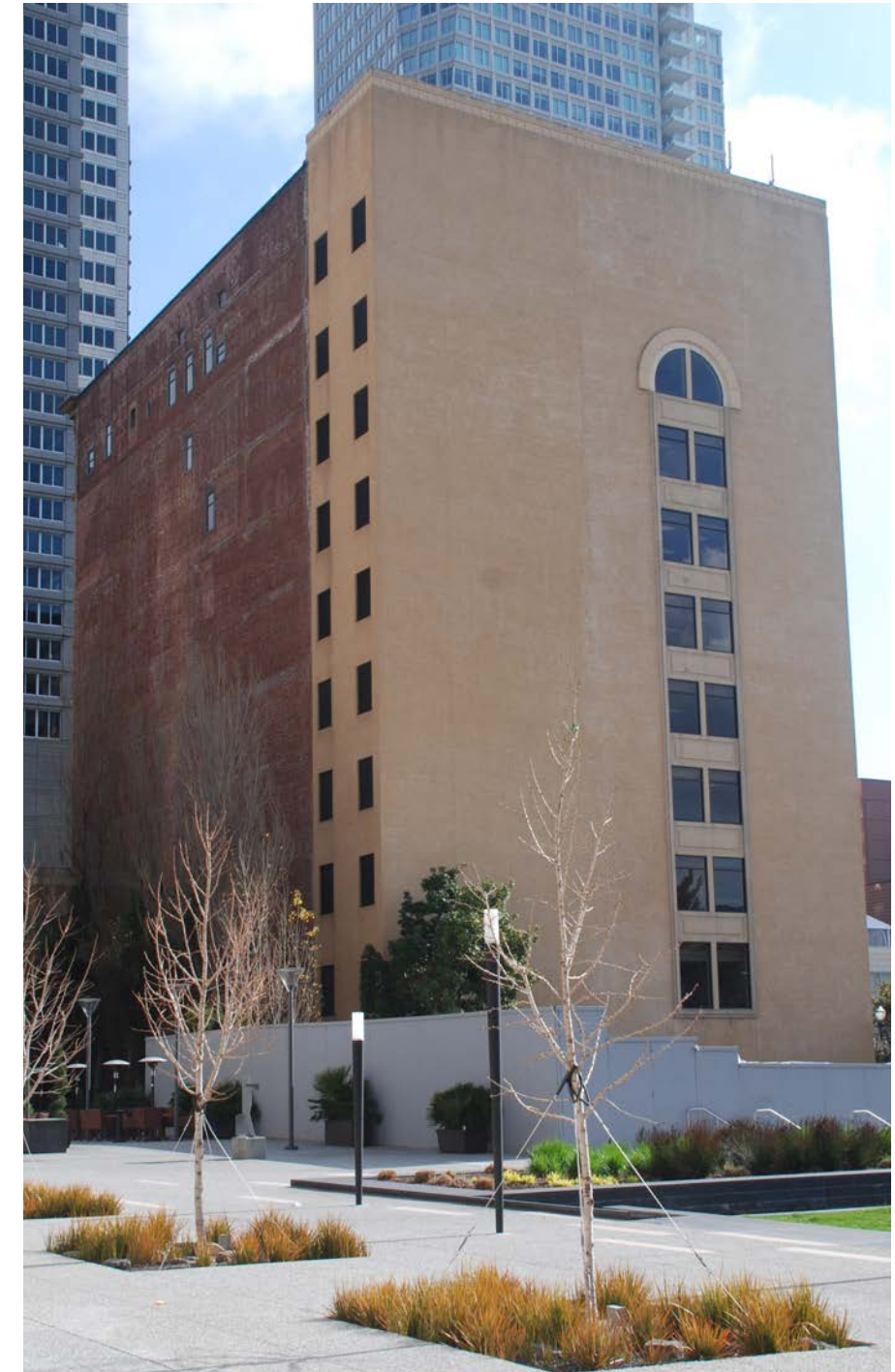
View of building from northwest. (Page & Turnbull)
