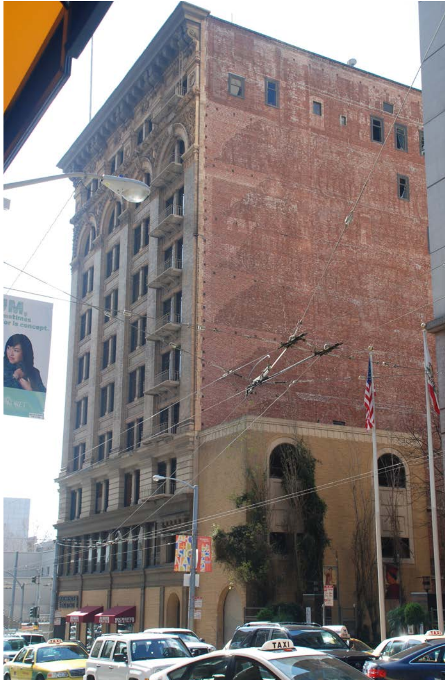
Existing north facade
