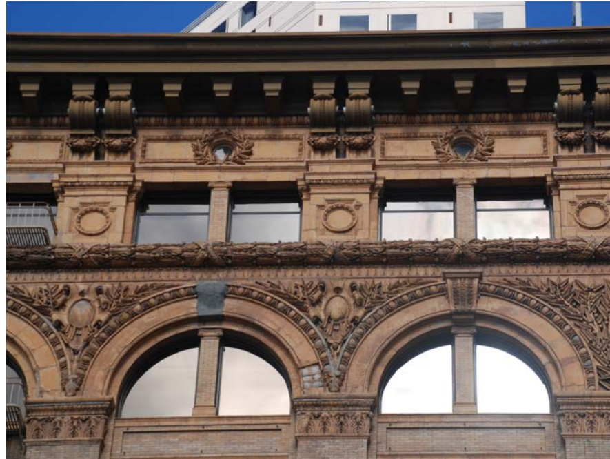
Terra cotta ornamentation at 9th and 10th floors
