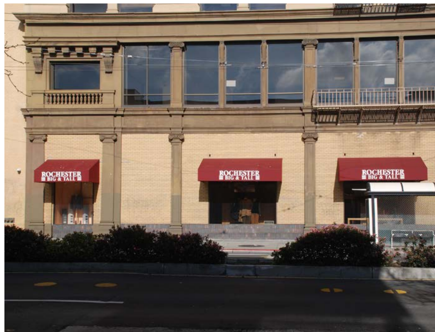
Brick infill at first floor
