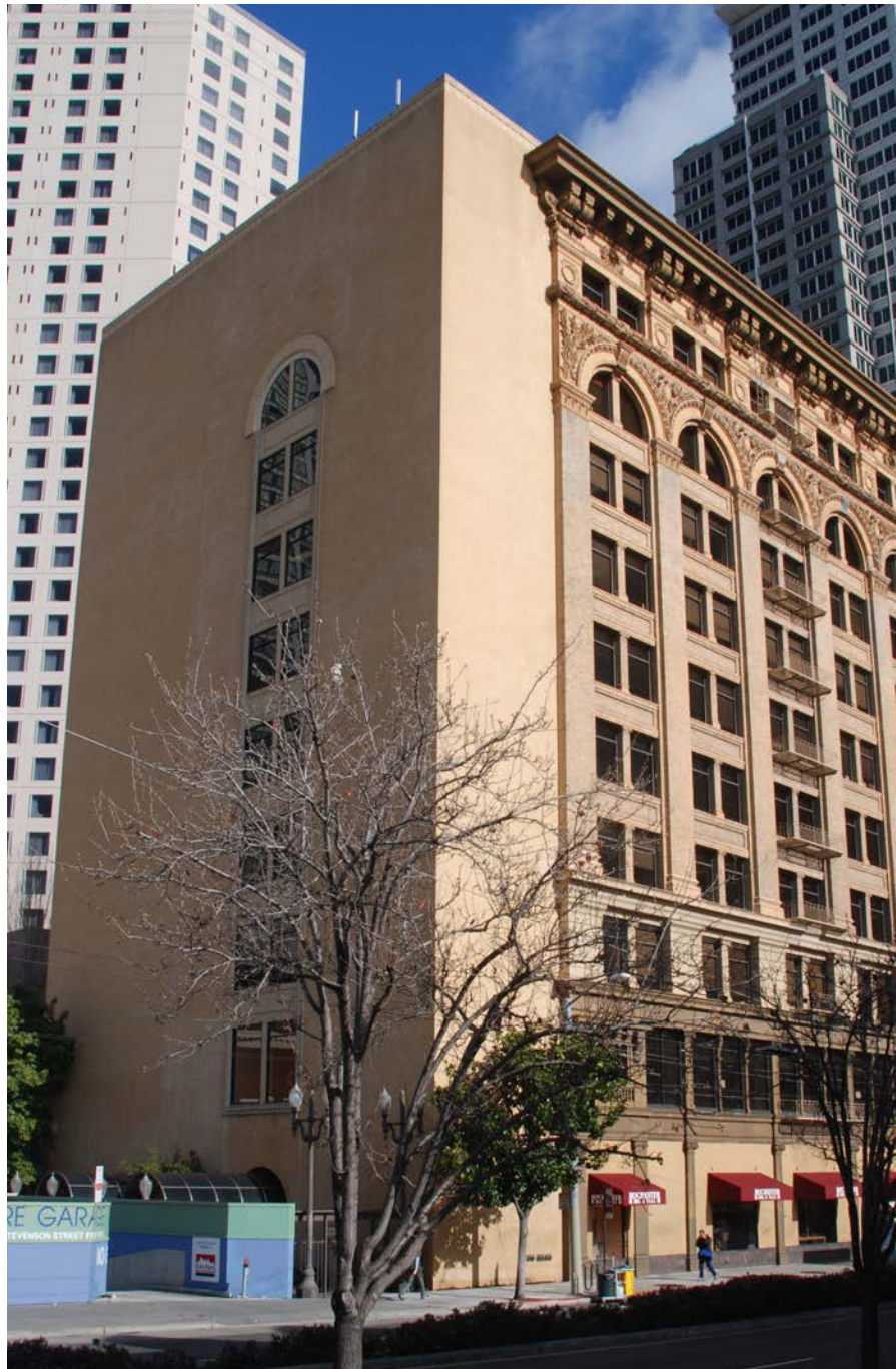
Non-historic addition at west facade, view from southwest
