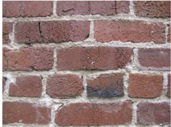
Figure 36. Exterior brick face. Source: Page & Turnbull, March 2010.
