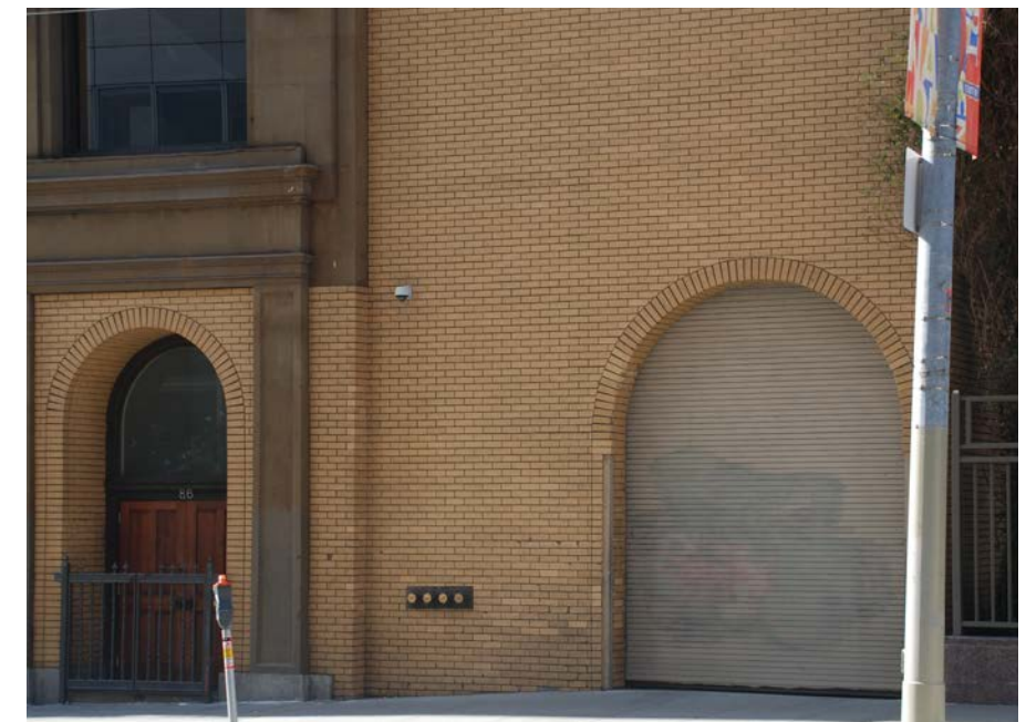
Ground level view of non-historic addition at north facade
