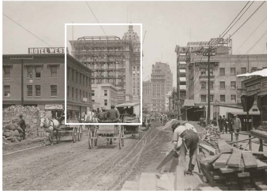
Aronson Building during the reconstruction after the 1906 Earthquake and Fire. (The Bancroft Library)
