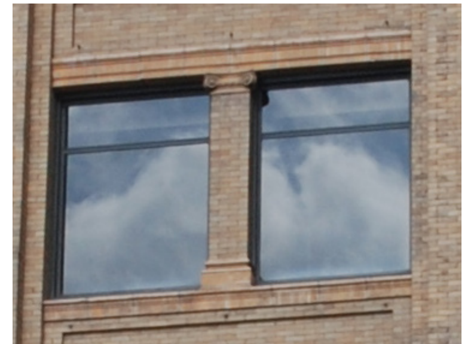
Enlarged View of Typical Existing Windows
