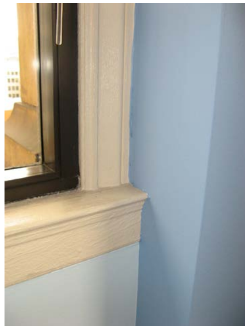
Figure 66. Interior window trim. Source: Page & Turnbull, March 2010.
