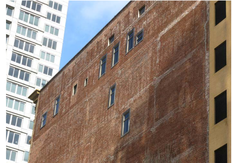
View of upper portion of north facade
