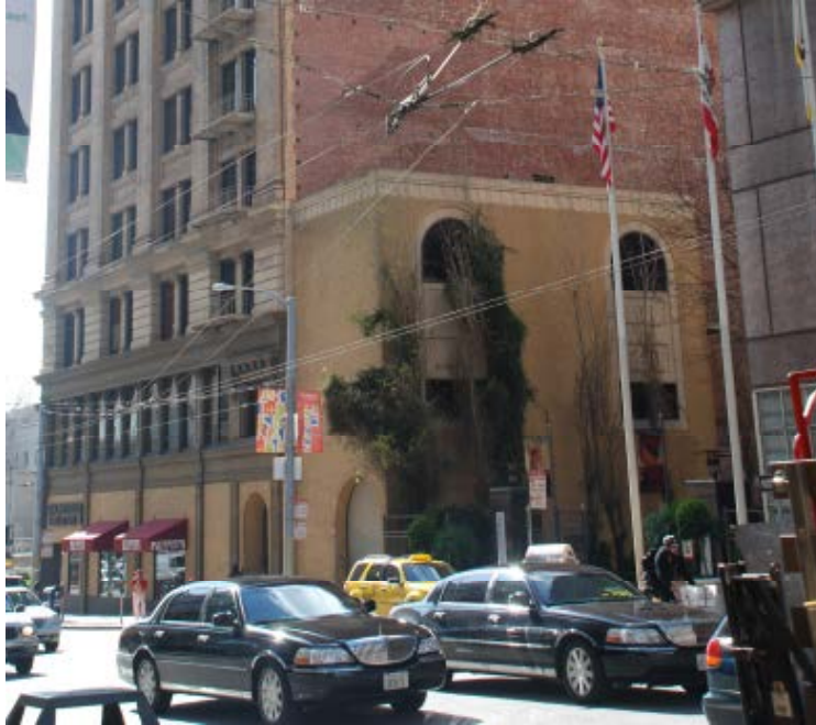
Figure 29. Northeast façade, three-story addition. Source: Page & Turnbull, March 2010.
