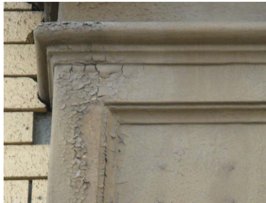
View of pilaster to be repaired
