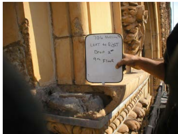
Figure 45. Removal of cracked piece shown at left. Source: Rainbow Waterproofing, 2006.
