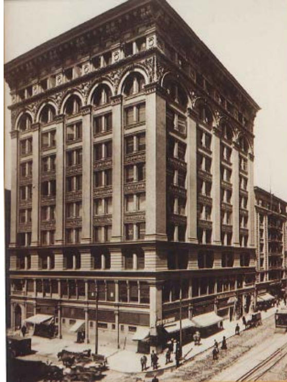
Figure 15. The Aronson Building at 3 rd and Mission streets, ca. 1909. Source: San Francisco Historical Photograph Collection, AAB-4731.
