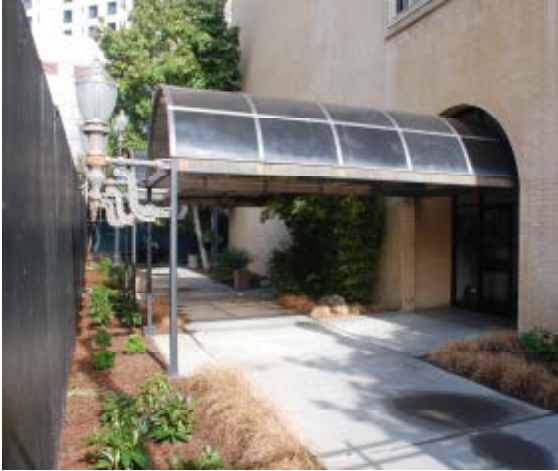
Figure 30. Southwest façade, walkway and entrance canopies.
