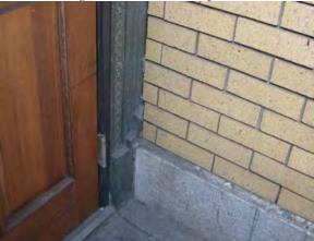
Figure 65. Corrosion of bronze frame. Source: Page & Turnbull, March 2010.
