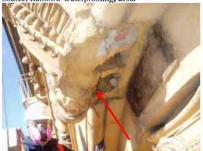
Figure 48. In-plane cracking of keystone. Source: Rainbow Waterproofing, 2006.
