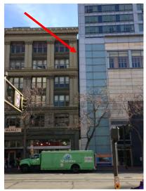
Photo of a seismic joint that is visible at 735 Market Street
