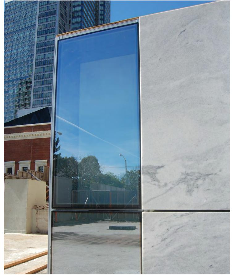
LOW-E HIGH PERFORMANCE INSULATING GLASS UNIT AND BACK-PAINTED SPANDREL PANEL
