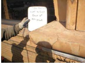
Figure 44. Cracking at cornice. Source: Rainbow Waterproofing, 2006.
