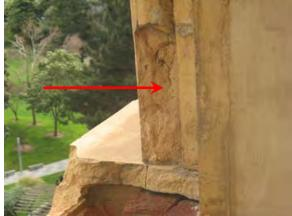
Figure 55. In-plane cracking at bisque spall. Source: Page & Turnbull, March 2010.
