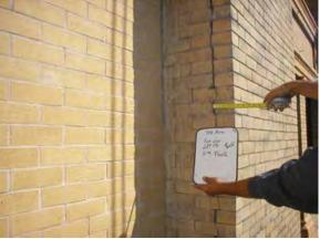
Figure 51. Cracking of terra cotta brick. Source: Rainbow Waterproofing, 2006.
