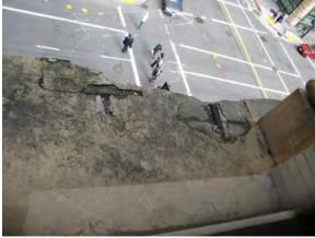
Figure 40. Cracking/spalling of concrete at steel corrosion. Source: Page & Turnbull, March 2010.
