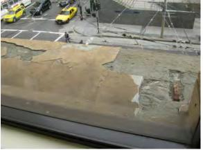
Figure 42. Exfoliation of crust. Source: Page & Turnbull, March 2010.
