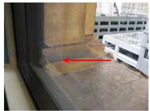
Figure 54. Cracking at column base. Source: Page & Turnbull, March 2010.
