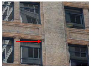
Figure 59. Missing brick. Source: Page & Turnbull, March 2010.
