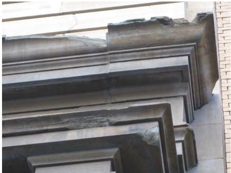
View of deteriorated colusa sandstone
