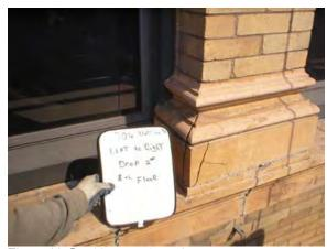
Figure 46. Cracking at column base. Source: Rainbow Waterproofing, 2006.
