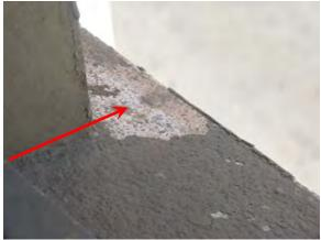
Figure 60. Corrosion of cast iron. Source: Page & Turnbull, March 2010.
