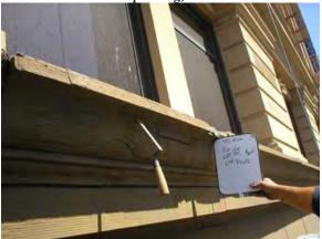
Figure 50. Cracking of sandstone. Source: Rainbow Waterproofing, 2006.
