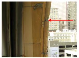
Figure 53. Shallow bisque spalls at joints. Source: Page & Turnbull, March 2010.
