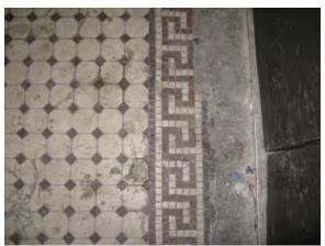
Figure 67. Cracking and soiling of ceramic tile. Source: Page & Turnbull, March 2010.
