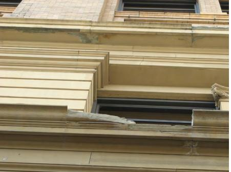
View of deteriorated colusa sandstone
