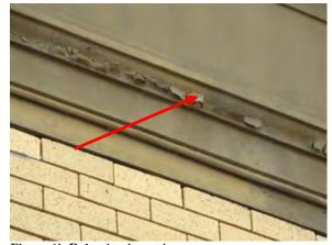
Figure 61. Delaminating paint. Source: Page & Turnbull, March 2010.
