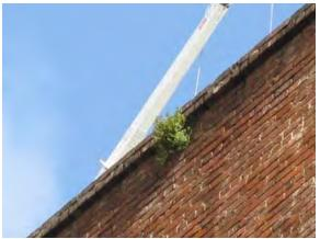
Figure 37. Weeds growing out of a parapet wall. Source: Page & Turnbull, March 2010.
