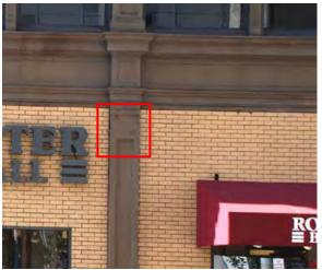
Figure 63. Missing scroll at column capital on 3<sup>rd</sup> Street facade. Source: Page & Turnbull, March 2010.
