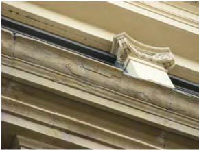
Figure 39. Cracking and spalling of sandstone at edge. Source: Page & Turnbull, March 2010.
