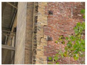
Figure 35. Cracking at terra cotta to brick interface. Source: Page & Turnbull, March 2010.
