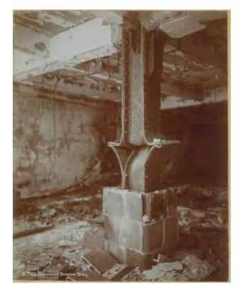
Figure 13. Buckled I-beam encased in failed hollow tiles in the basement, 1906. Source: Bancroft Library.
