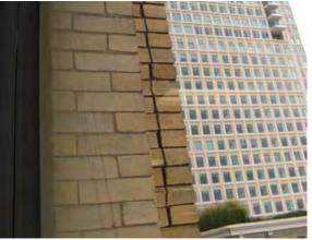
Figure 58. Cracking at column corner. Source: Page & Turnbull, March 2010.
