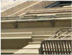
Figure 41. Spalling of sandstone at edge. Source: Page & Turnbull, March 2010.
