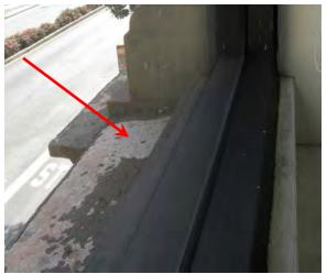
Figure 62. Area of exposed cast iron with no paint. Source: Page & Turnbull, March 2010.
