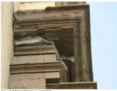
View of deteriorated colusa sandstone
