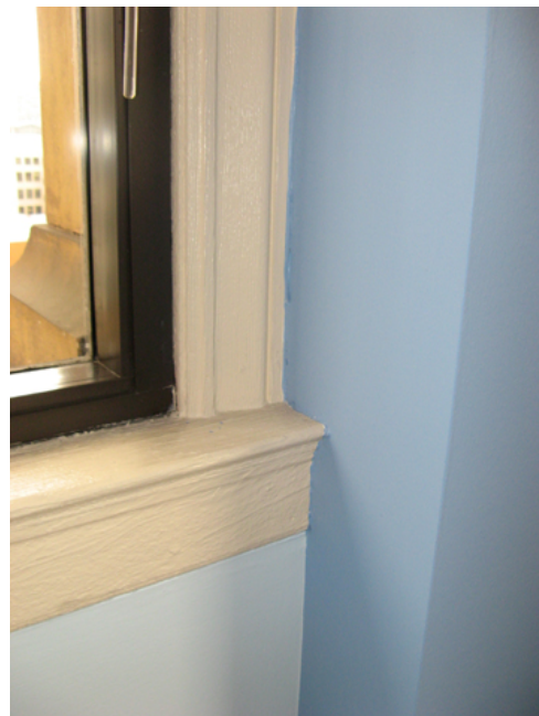
Figure 66. Interior window trim. Source: Page & Turnbull, March 2010.
