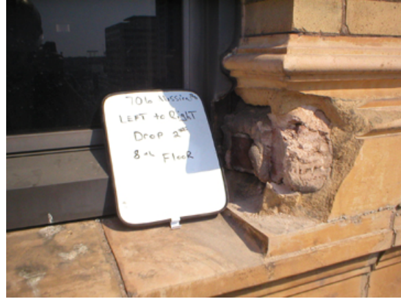
Figure 47. Removal of cracked piece shown at left. Source: Rainbow Waterproofing, 2006.
