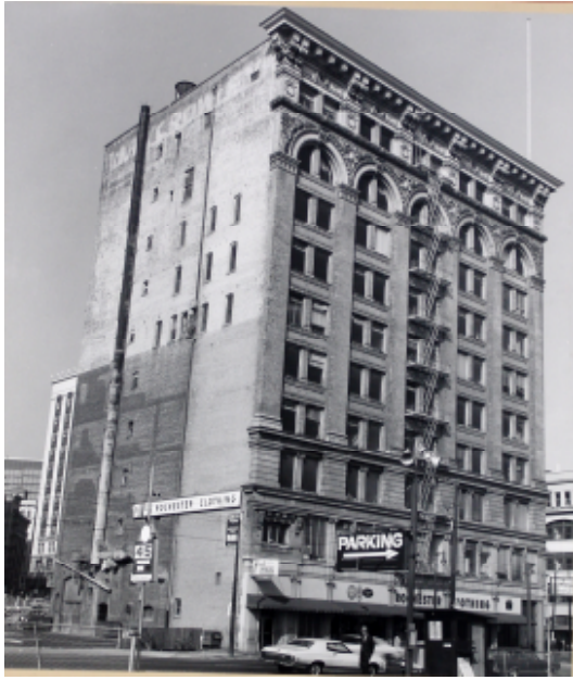
Figure 18 and 19. The Aronson Building, ca. 1970s Source: Turnstone Consulting.
