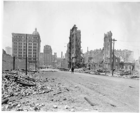
Figure 11. The Aronson Building is on the left. Source: San Francisco Historical Photograph Collection, AAC-3600.
