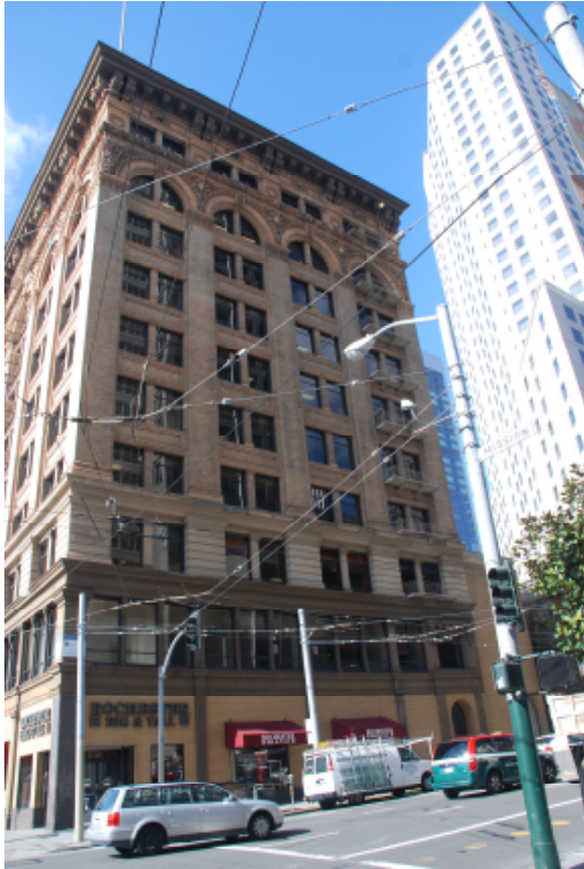
Figure 27. Northeast (3rd Street) façade. Source: Page & Turnbull, March 2010.
