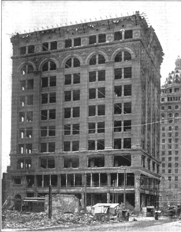
Figure 12. The caption to this 1906 newspaper photo reads: "ARONSON BUILDING. Northwest Corner Third and Mission Streets. The facades for the three lower stories consist of Colusa sand-stone, which is badly spalled and damaged. The upper stories of buff terra cotta pressed brick, with terra cotta ornaments, are but slightly injured, the terra cotta being spalled and cracked in a few places. The metal cornice is completely wrecked. The rear walls of common brick were considerably racked and damaged by the earthquake. All the walls remain practically plumb. Columns in the basement, first, fifth, eighth and tenth stories have buckled on account of the failure of the hollow tile protection. The Roebling concrete floors, with crimped wire lath and cement plastered soffit protection, remain in first-class condition throughout, notwithstanding the warped condition of the steel work, due to the buckling of the columns. The 4" hollow tile partitions are badly wrecked throughout, about 80 percent of the entire work having fallen down. The failure of the hollow tile partitions totally wrecked the cast-iron and marble tread stairways." Source: Unknown (clipped file).
