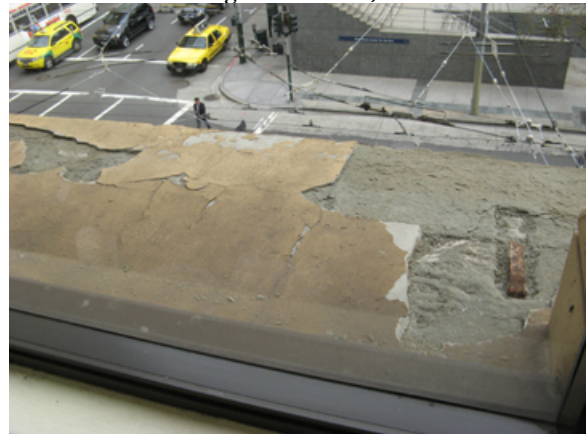
Figure 42. Exfoliation of crust. Source: Page & Turnbull, March 2010.
