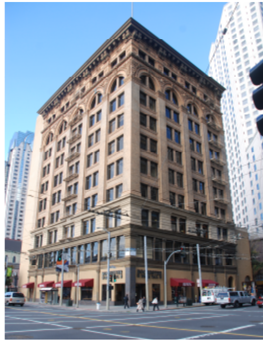
Figure 24. Southeast (Mission Street) façade and northeast (3 rd Street) façade.
