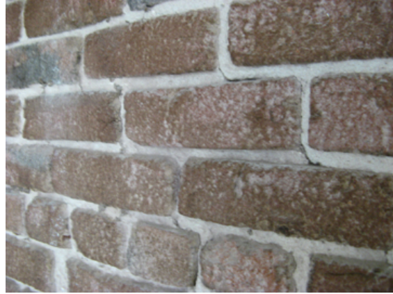
Figure 38. Interior brick face. Source: Page & Turnbull, March 2010.
