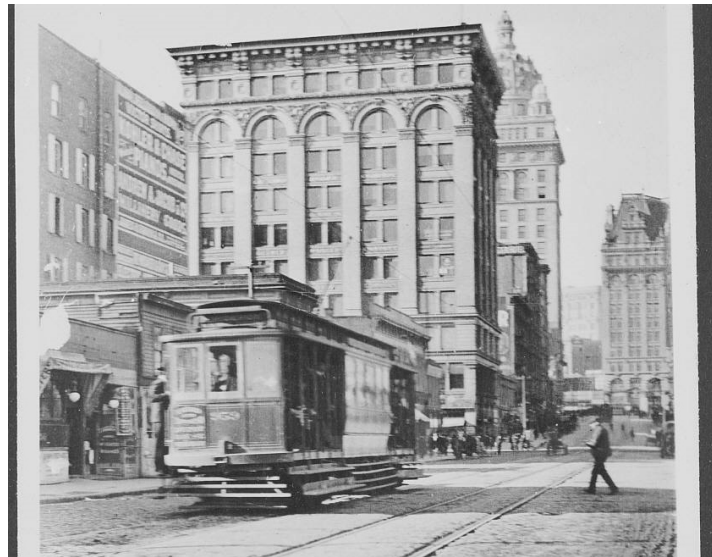
Figure 09. Looking north on 3 rd Street, 1905. Source: Bancroft Library.
