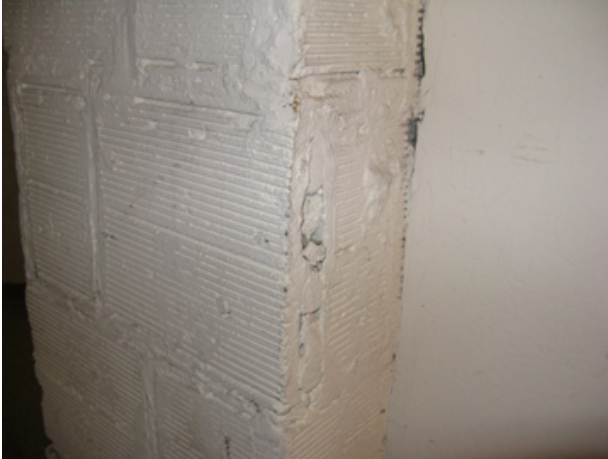
Figure 32. Column encased with terra cotta tile. Source: Page & Turnbull, March 2010.
