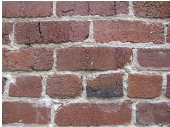
Figure 36. Exterior brick face. Source: Page & Turnbull, March 2010.
