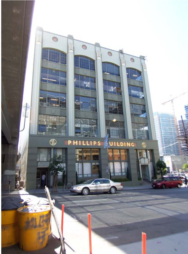
2 nd Street façade, 100_3718, 9.19.07
