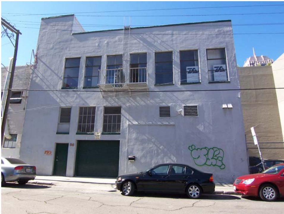
Tehama Street elevation, 100_4125, 9.24.07
