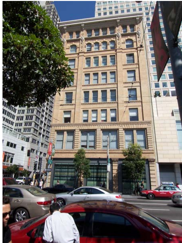
Third Street Façade, 100_4570, 9.27.07
