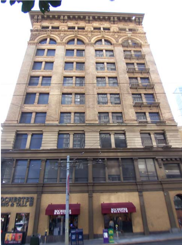
View of 3 rd Street façade, 100-4714, 9.27.07
