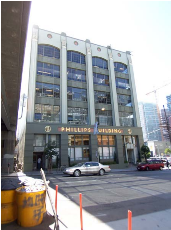
Figure 7. Phillips Van Orden Building, 2007
