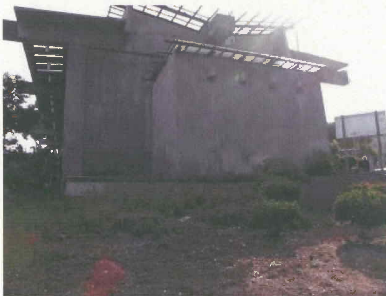
View south toward the Glen Park BART Station's north elevation, 2009.
