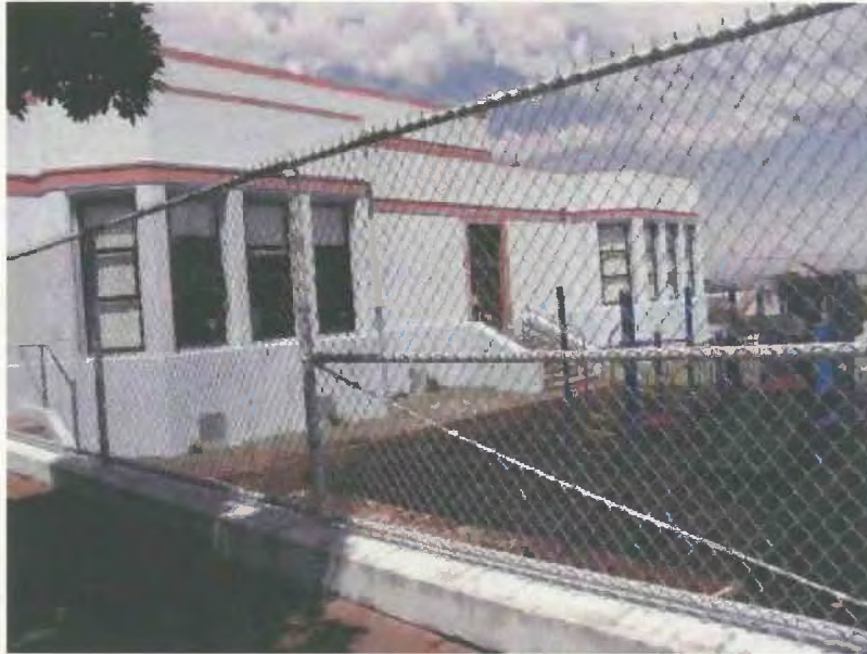
View north toward the school's south elevation, 2009.
