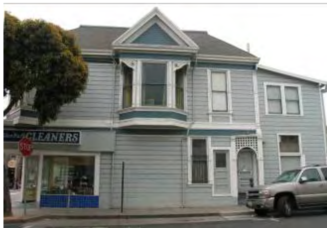
View south toward 107 Chenery Street, 2009.
