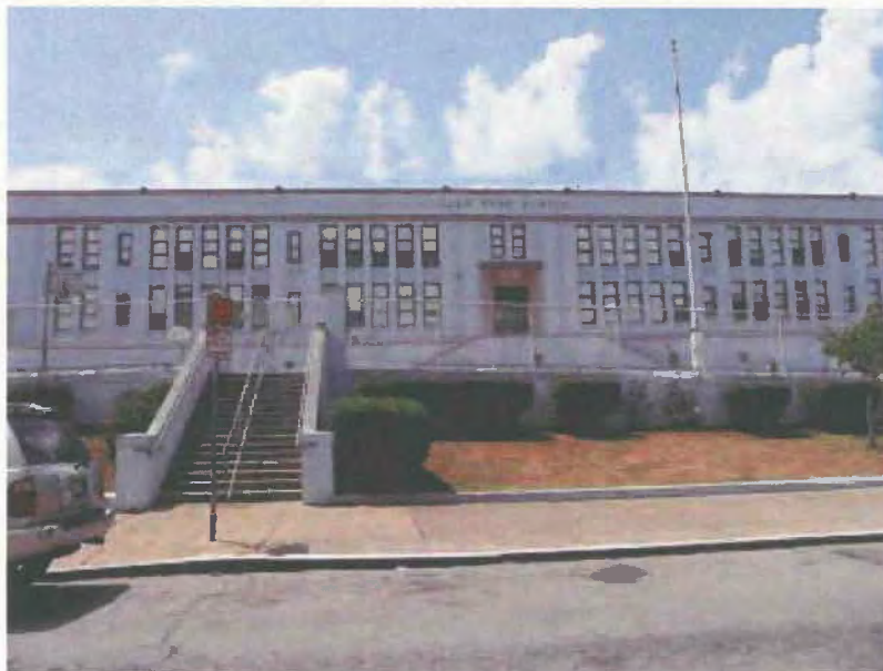
View west toward the school's east elevation, 2009.
