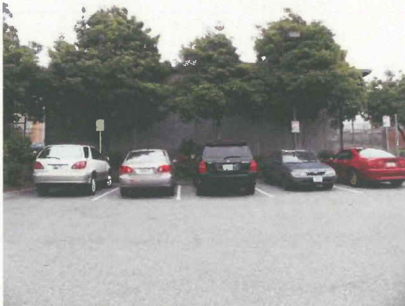
View north toward the Glen Park BART power station's south elevation, 2009.
