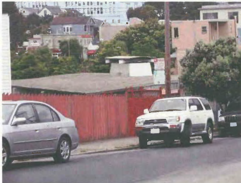
View south toward the Glen Park BART power station's north elevation, 2009.
