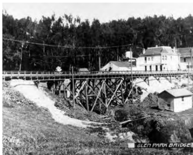
View of the SF & SM Railway’s trestle spanning Islais Creek, no date. Courtesy of the San Francisco Public Library.
