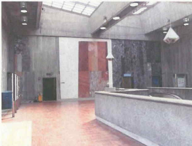
View of the station's interior tile mosaic along the south wall, 2009.
