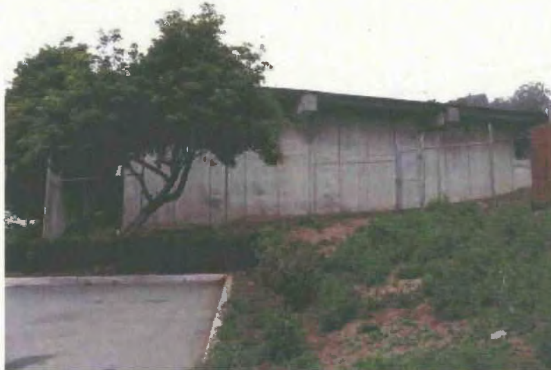
View west toward the Glen Park BART power station's east elevation, 2009.
