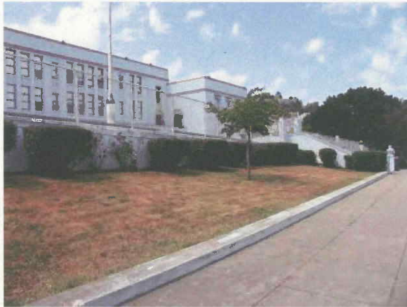
View northwest toward the school's east elevation, 2009.
