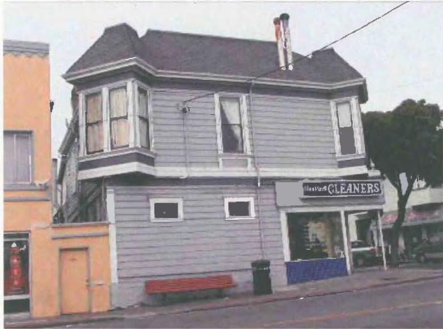
View of the east façade from Diamond Street (Carey & Co., June 2, 2009).
