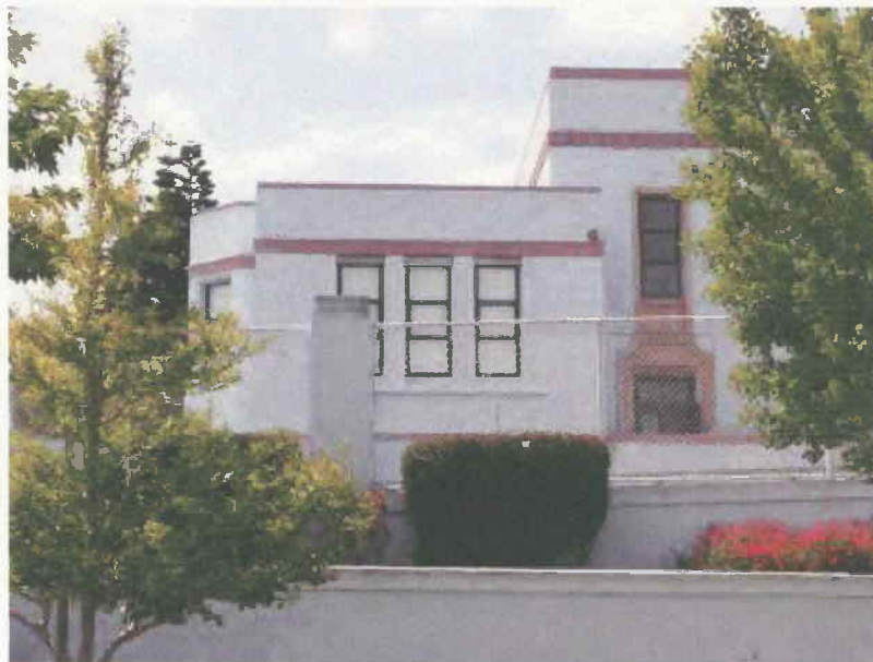
View west toward the school's east elevation, 2009.
