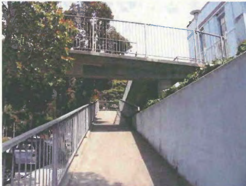
View east toward the pedestrian ramp on the school's north elevation, 2009.
