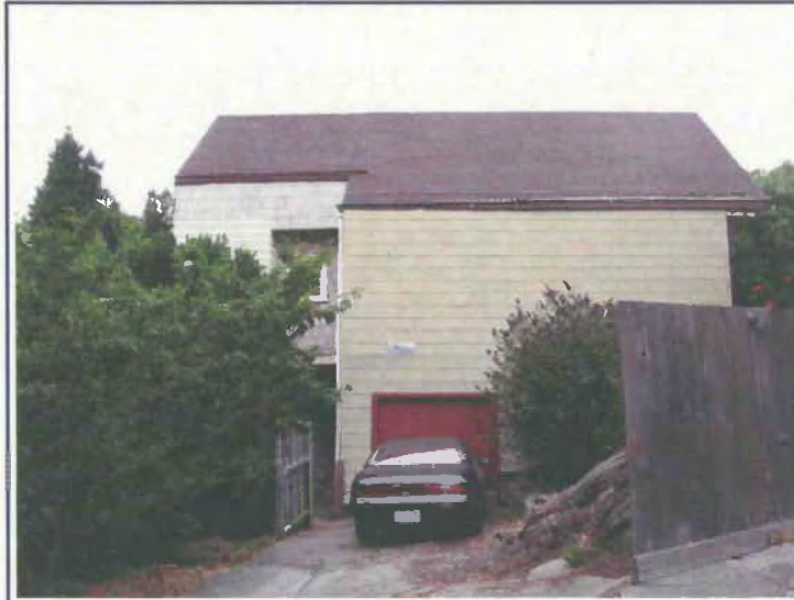
Description: View from Burnside looking west
