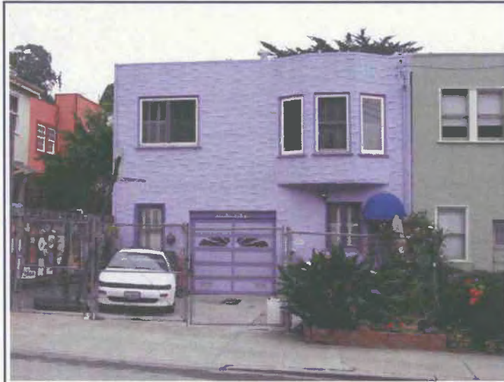
Description: View from Paradise looking north Photo Date: 07/17/2009
