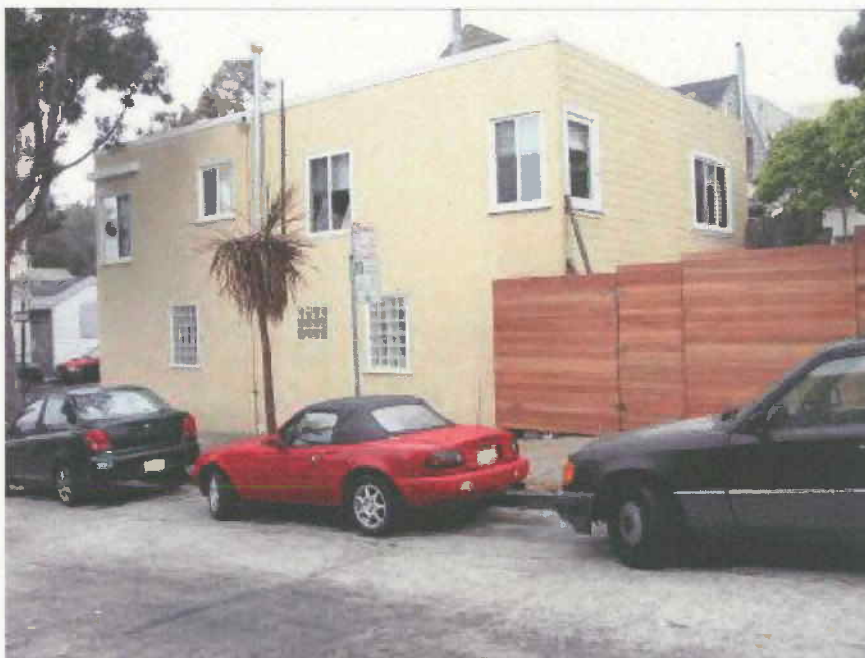
View of east and north elevations from Thor Avenue (Carey & Co., June 2, 2009).
