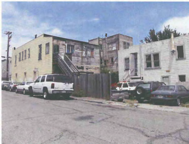
View northwest on Kern Street toward 23-25 Brompton Avenue, 2009.
